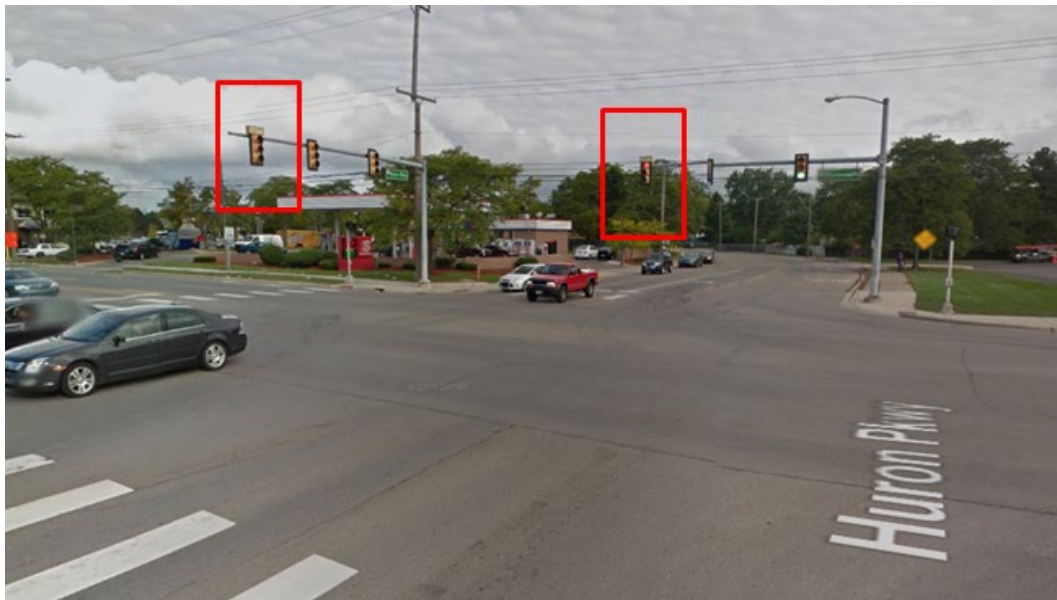
Figure 10. Left-Turn Arrows at an Intersection (Image Produced Using Google Street View)
