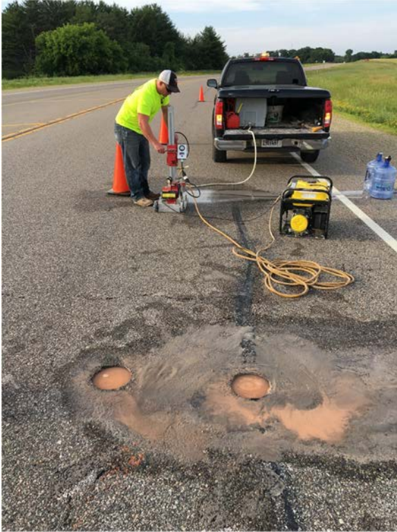
(a) Coring HMA surface
