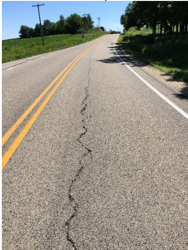
(b) Pavement section II with CA base layer in 2009 before mill and overlay
