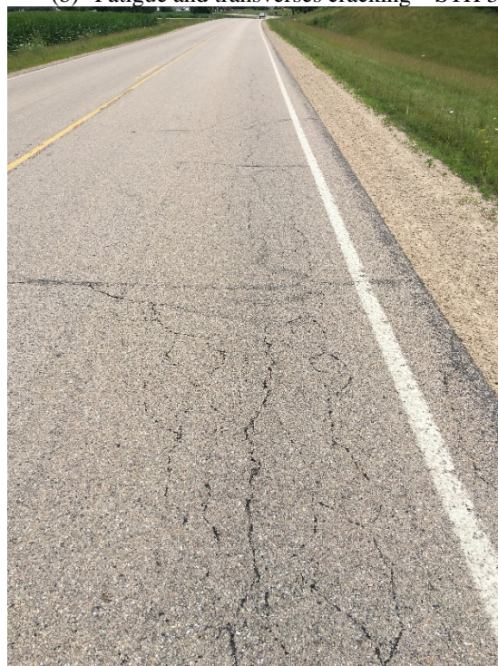
(b) Fatigue and transverse cracking – STH 33
