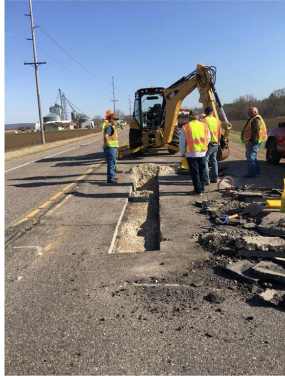
(b) Excavating HMA surface
