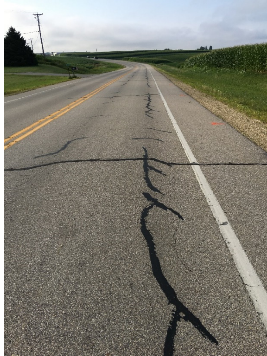
(b) Fatigue and transverse cracking – STH 33
