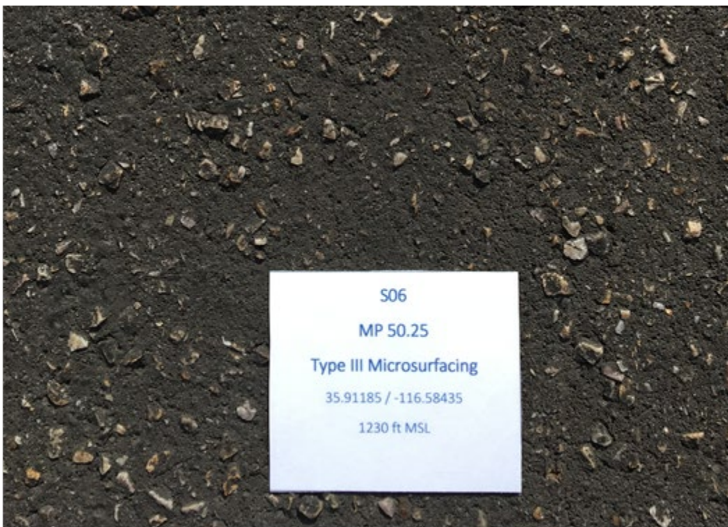
Figure 12. Type III microsurfacing treatment at site S06, March 2019 (VOLPE CENTER)
