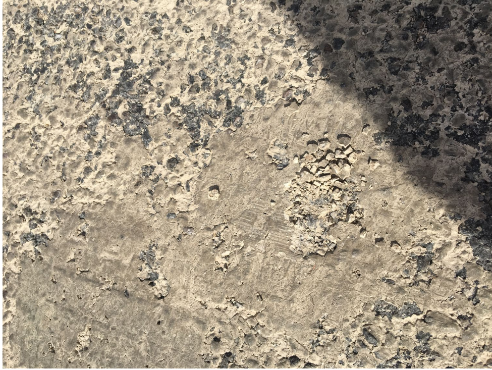
Figure 2. Example (worst-case) of mud-caked roadway as seen on northern Badwater Road, March 2019 (VOLPE CENTER)
