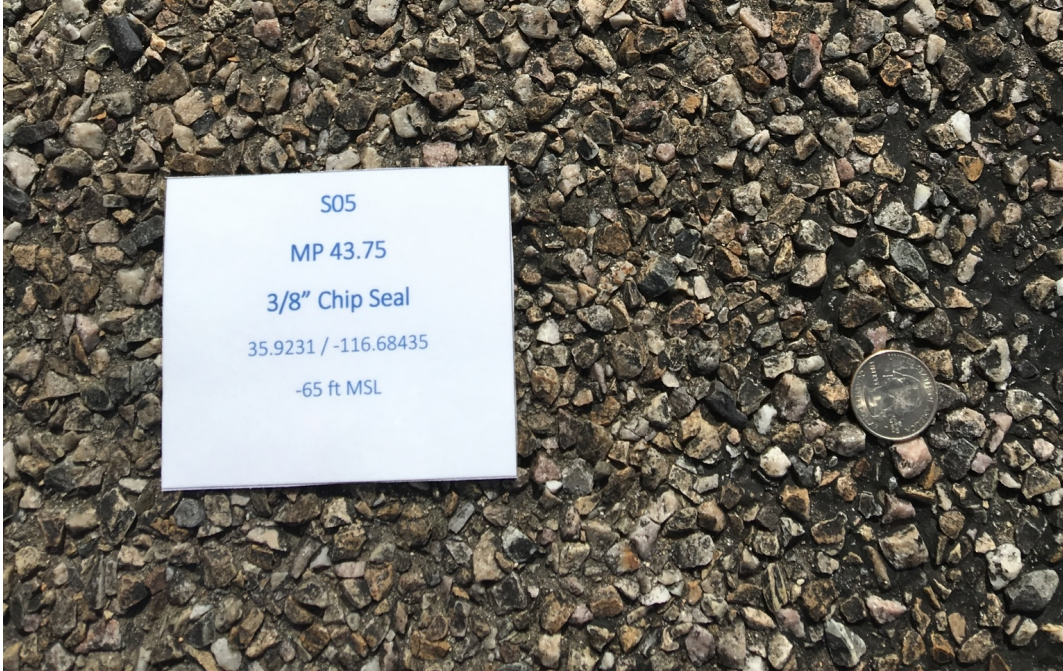
Figure 6. 3/8-inch chip seal treatment at site S05, March 2019 (VOLPE CENTER)
