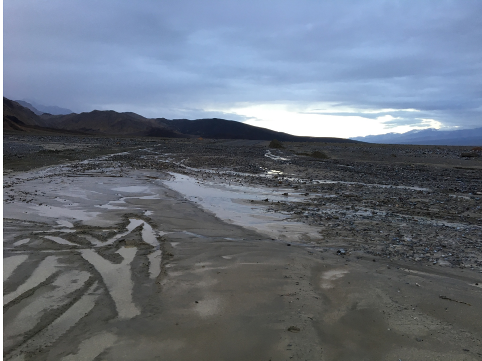
Figure 3. Example of March 2019 flood conditions on northern Badwater Road (VOLPE CENTER)
