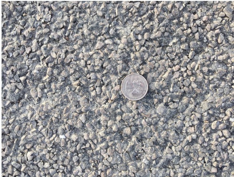
Figure 7. 1/4-inch chip seal treatment at site S02, March 2019 (VOLPE CENTER)
