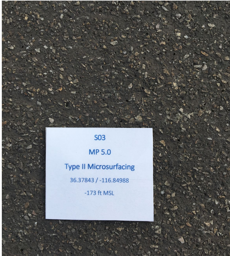
Figure 9. Type II microsurfacing treatment at site S03, March 2019 (VOLPE CENTER)
