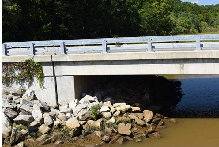
Figure 37. Photo. High-resolution UAS-collected imagery of riprap at Bacon Ridge Bridge.
