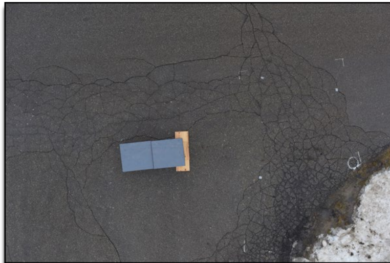
Figure 50. Photo. The model bridge with settlement in place as collected from the UAS with 36 megapixel camera at 50 ft (15m) height.
