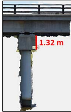
Figure 32. Illustration. Model of bridge cap-beam (Tuckahoe Creek Bridge) with its measured height.
