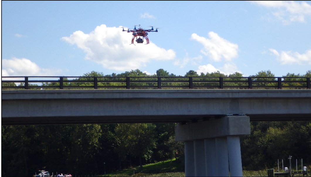
Figure 22. Photo. The hexacopter platform collecting bridge image data at the Tuckahoe Creek site.
