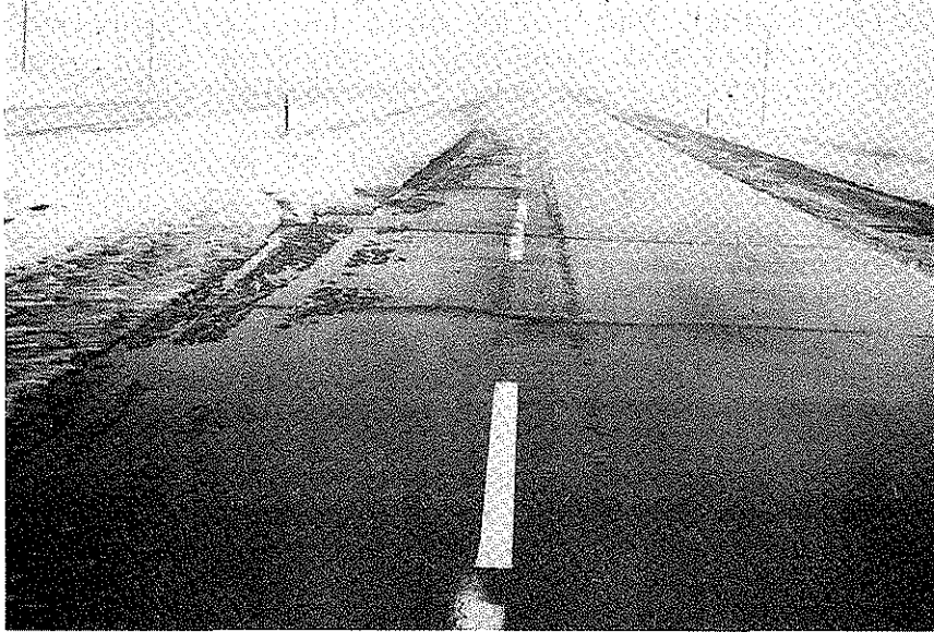
Figure 3. ETP Bituminous Concrete Pavement (US 40 Colorado) in March 1979.
