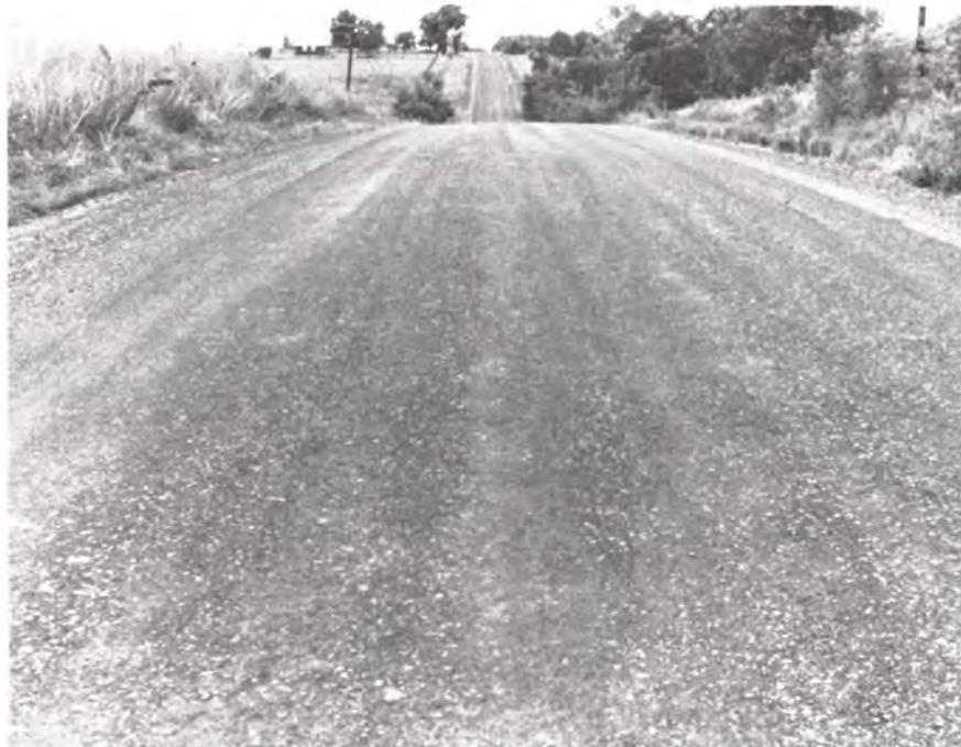
The recycled pavement shaped and compacted. Because traffic raveled the surface, it was decided that County forces would apply a chip seal coat.
