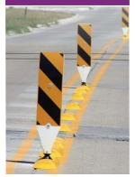
Temporary islands made of raised curbing and/or vertical markers can be removed and replaced, as needed, and give drivers the sensation of constricted lane widths, thus encouraging deceleration.
