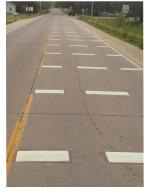
This pavement marking treatment creates a visual effect that encourages motorists to slow down. The bar placement guides motorists to direct the vehicle's wheels in gaps between the bars, which results in the driver unconsciously slowing down.
