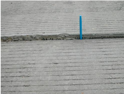
Figure 4.77: Faulting Example
