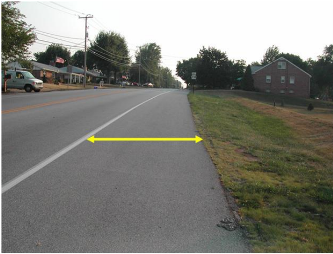
Figure 4.57: Bituminous Shoulder Measurement
