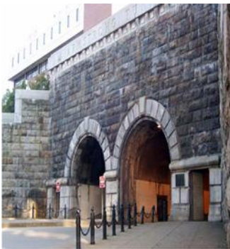
Figure 4.11: Tunnel (Code ‘2’) Example
