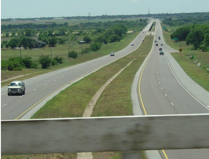
Figure 4.48: An Example of Median Type = 2, Unprotected
