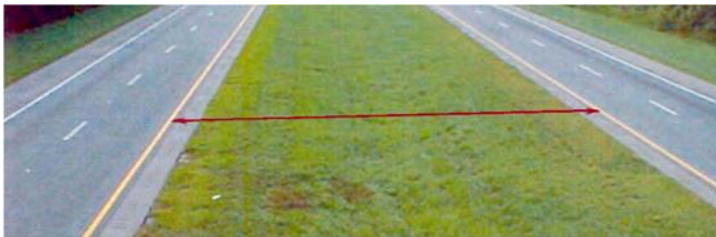
Figure 4.50: Median Width Measurement
