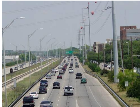
Figure 4.66: Major Rail Line (Code “B”) Obstacle Example
