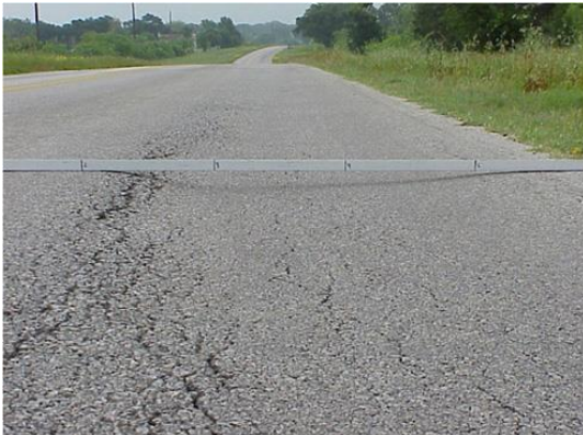
Figure 4.75 Rutting Example
