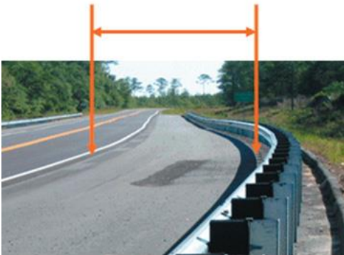
Figure 4.58: Measuring Shoulders with Guardrails
