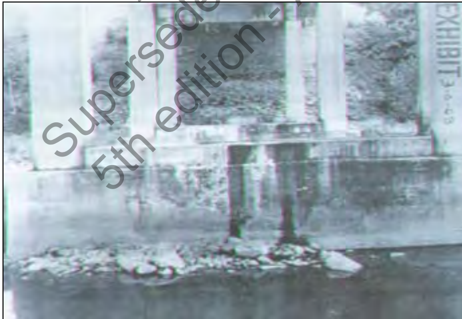
Figure 11.2. Photograph of riprap at pier 2, August 1977 (flow is from right to left). (98,99)
