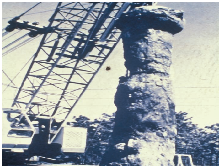
Figure 1. Defective drilled shaft with multiple types of anomalies (DiMaggio, 2008).
