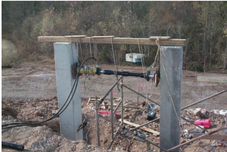
Figure 10.6 Photo of Field Static Load Test
