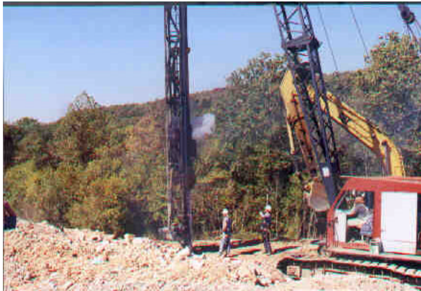
Figure 10.5 Driving of Pile Section
