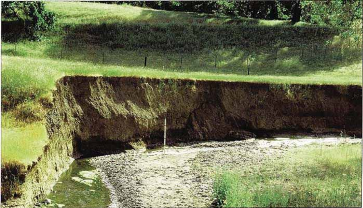
Figure 12. Photo. Unstable channel, evidenced by stream bank erosion and vertical bank. (6)
