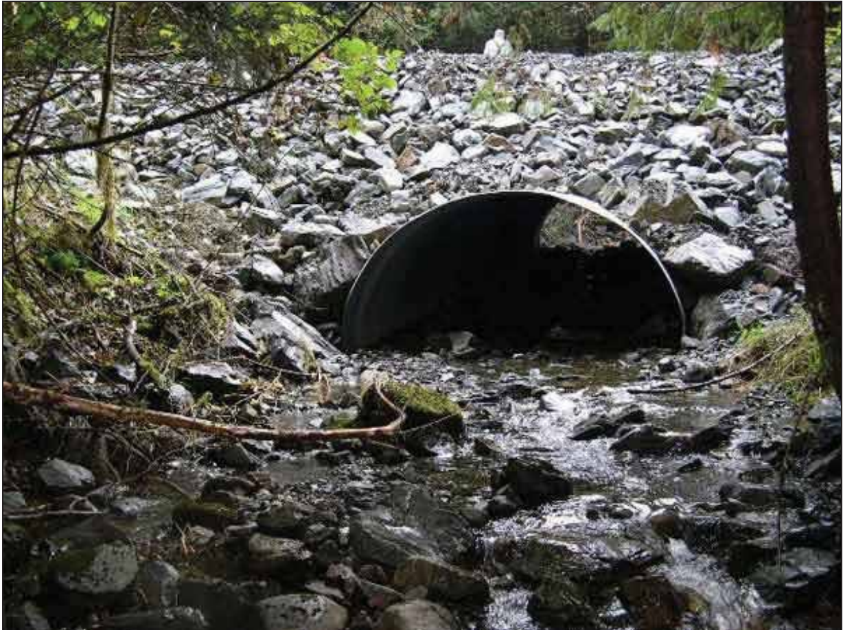
Figure 17. Photo. An aquatic organism passage (AOP) culvert. (8)
