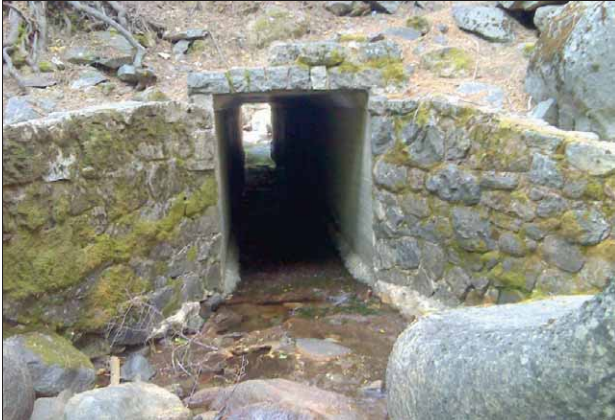
Figure 35. Photo. View downstream of concrete box culvert with masonry appurtenances.
