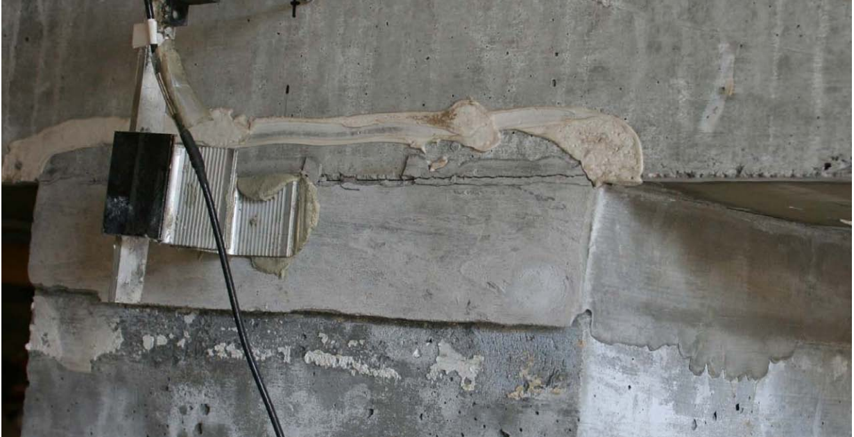
Figure 47. Photo. West end and south face of test specimen immediately after completion of test.
