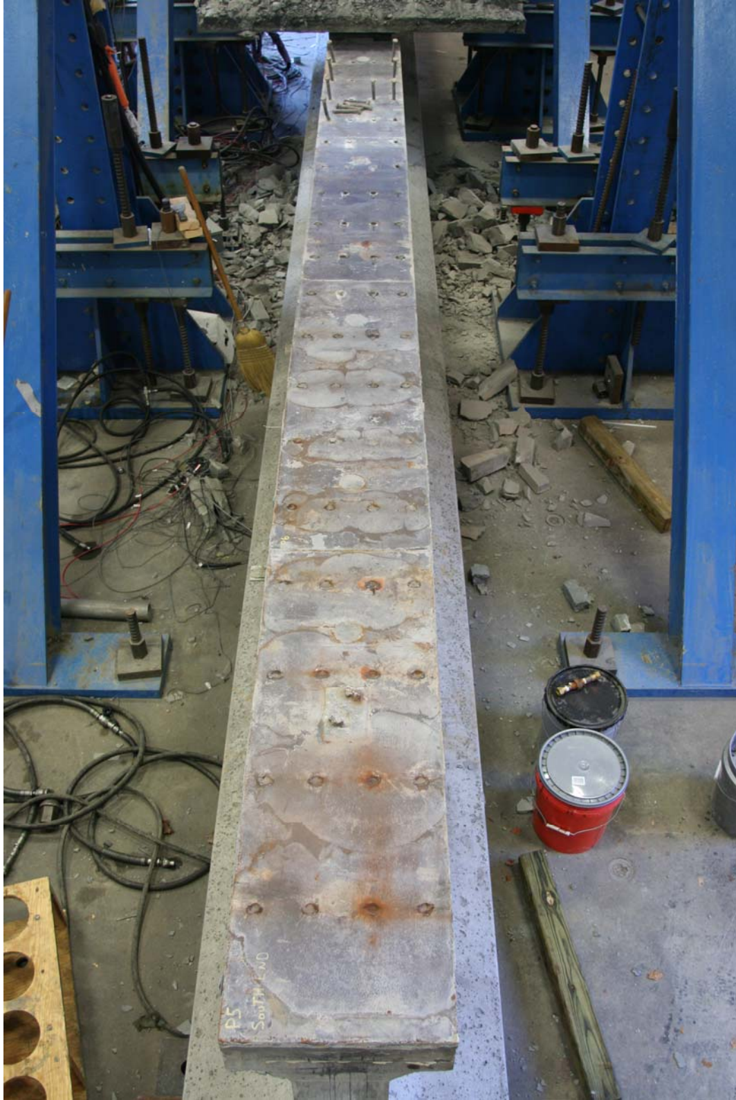
Figure 53. Photo. Emulated steel girder composite connection after completion of test and removal of haunch/deck.
