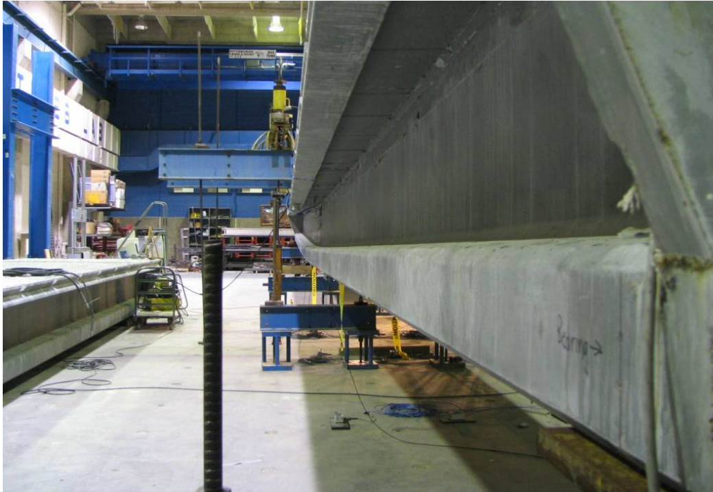
Figure 78. Photo. North face of Girder P2-70F after 230 mm (9 inches) of deflection.
