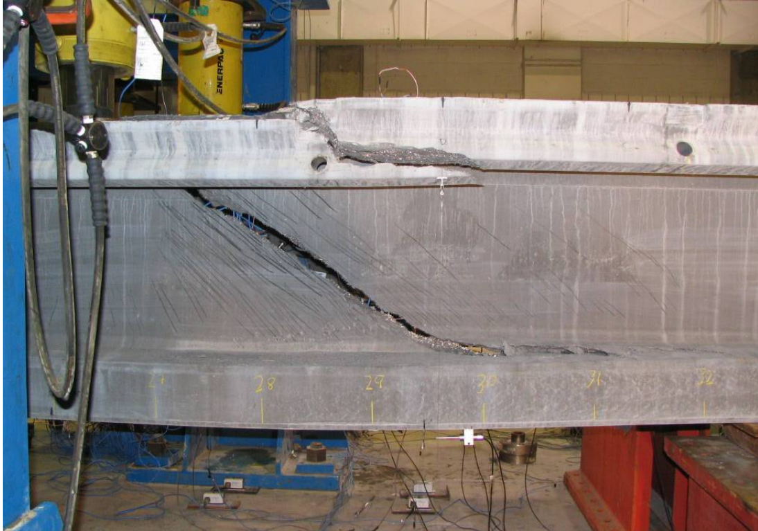
Figure 107. Photo. South face of Girder P2-21S after shear failure.
