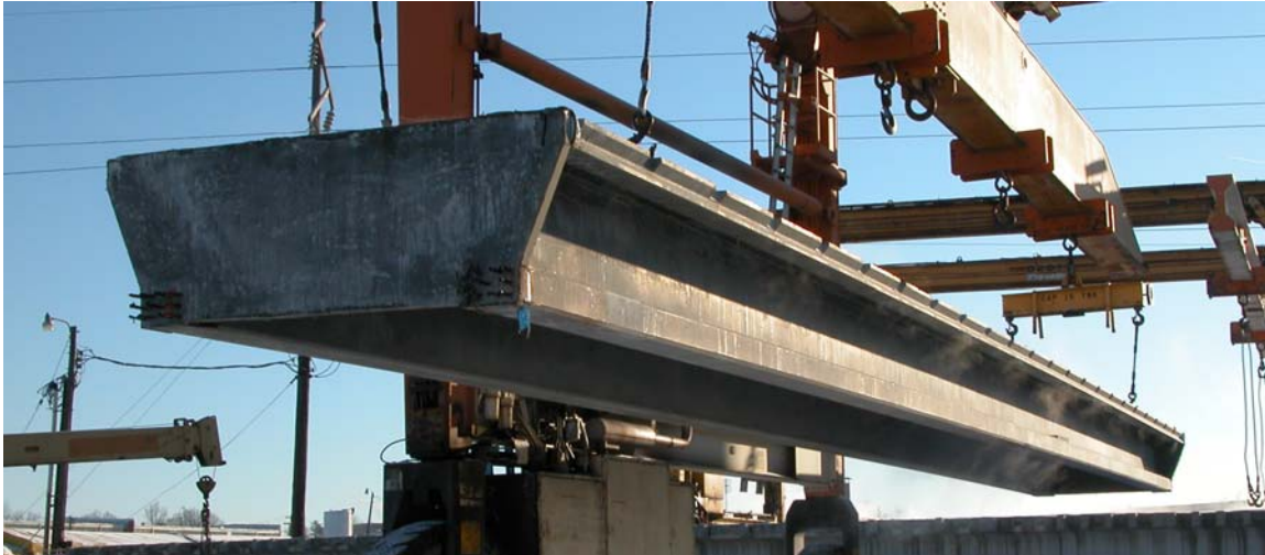
Figure 4. Photo. Fabricated girder with diaphragm prior to steam treatment.
