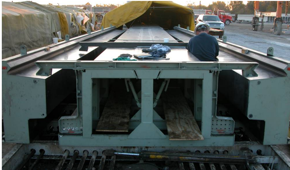
Figure 2. Photo. Girder formwork.
