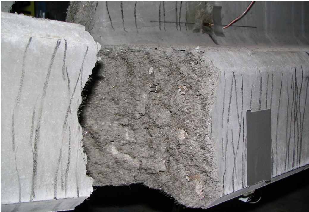
Figure 79. Photo. West face of Girder P2-70F south bulb failure surface.
