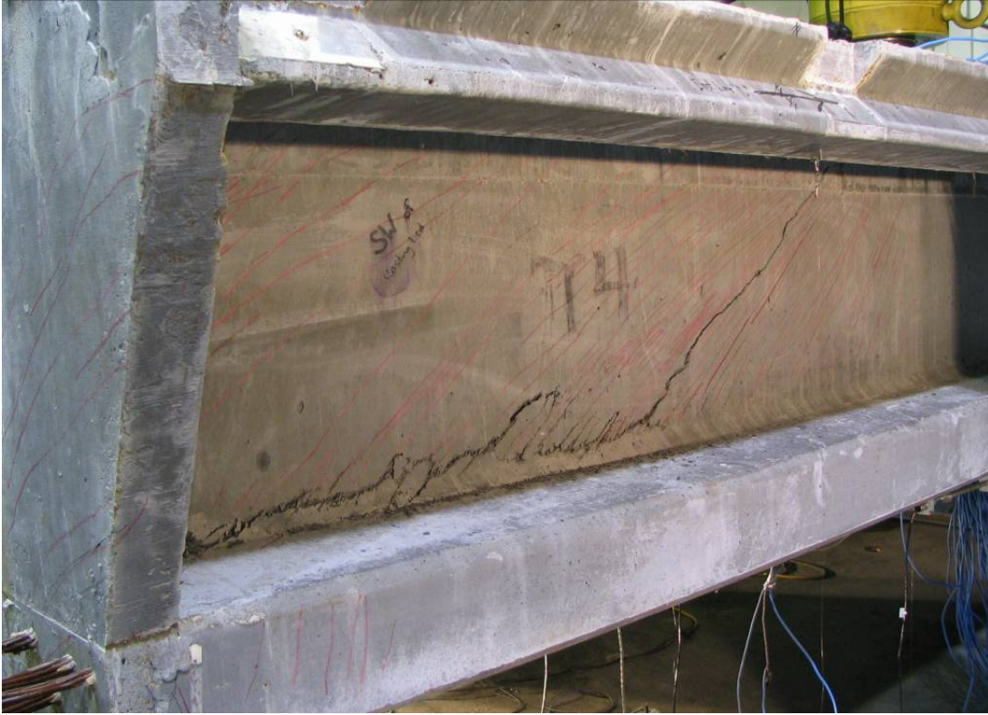
Figure 120. Photo. Northeast end of P4-57Sh after failure.
