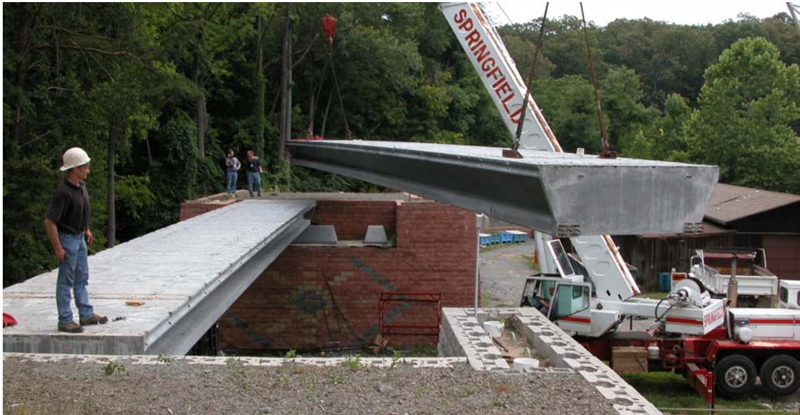
Figure 5. Photo. Erection of test bridge.
