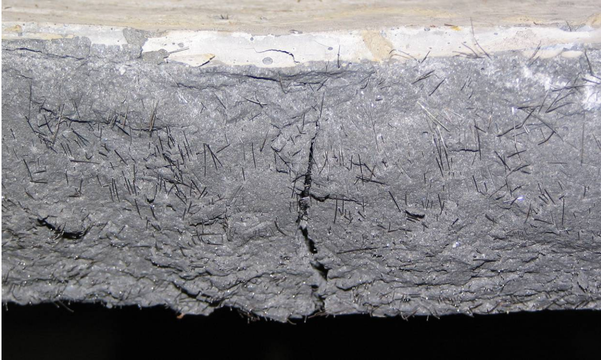
Figure 147. Photo. Failure crack in P4-24T as observed after conclusion of test.
