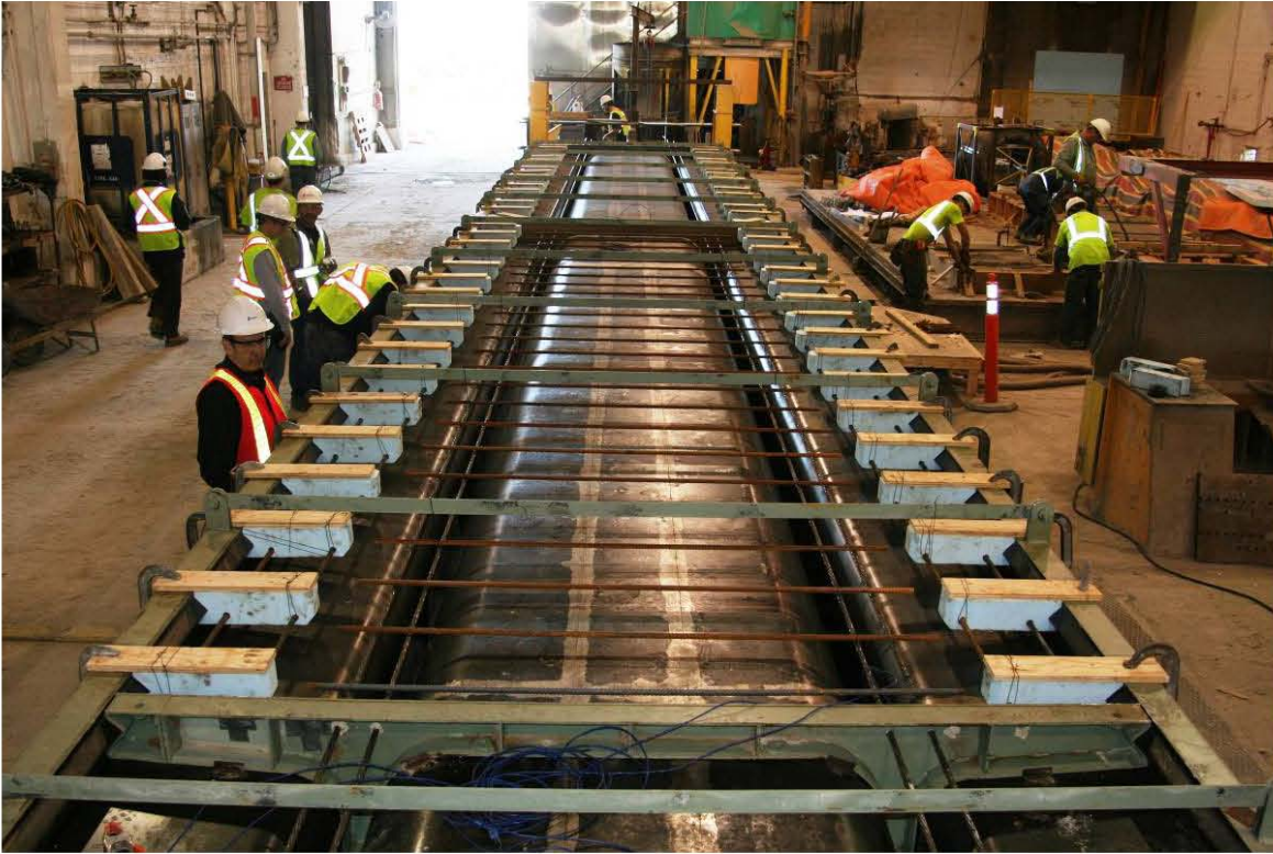
Figure 11. Photo. Girder formwork for T2 (near) and T1 (far).
