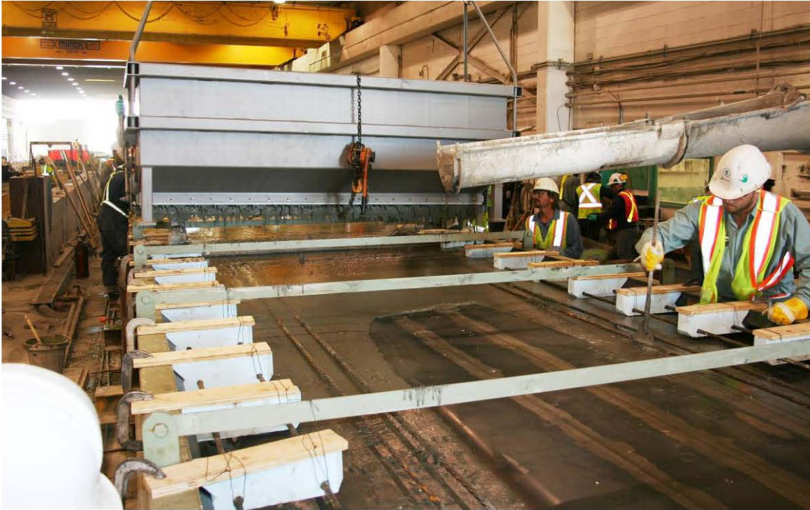
Figure 14. Photo. Concrete placement for girder deck.
