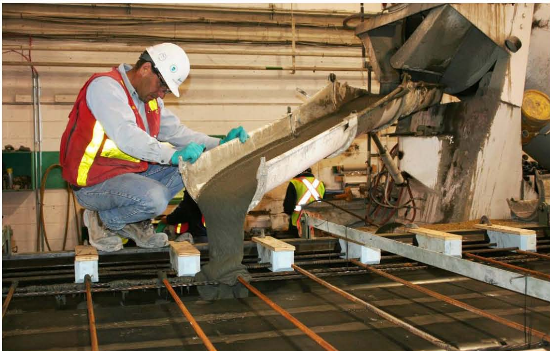
Figure 13. Photo. Concrete placement for girder legs.
