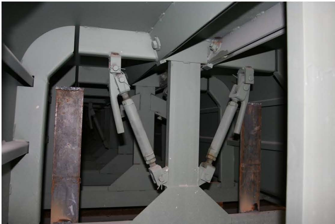
Figure 10. Photo. Girder formwork mechanism for releasing transverse restraint.
