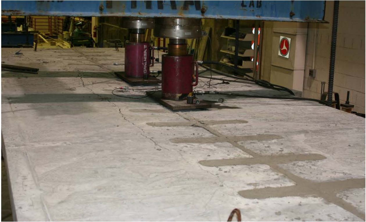
Figure 83. Photo. Top of deck at peak applied load during Test T2J.
