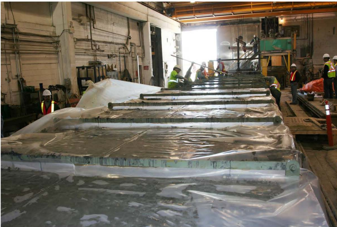
Figure 15. Photo. Plastic tarp installed immediately after concrete placement.
