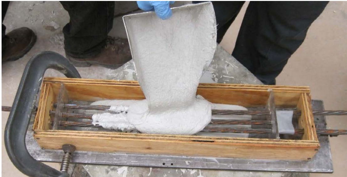
Figure 3. Photo. Casting of a 20 inch (50.8 cm) long test specimen.
