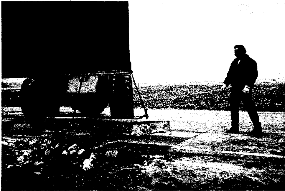
Figure 6: Contractors remove slab on 5 November 1997.
