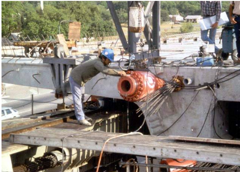
Figure 2.7 Jacking of Post-Tensioning Tendon
