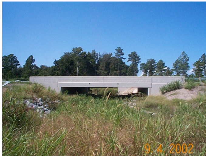
Figure 2.60 Precast Prestressed Plank (spans 20 to 40 feet)
