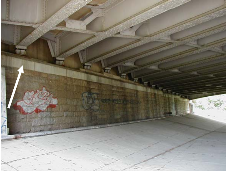
Figure 2.41 Discontinuous Cross Frame
