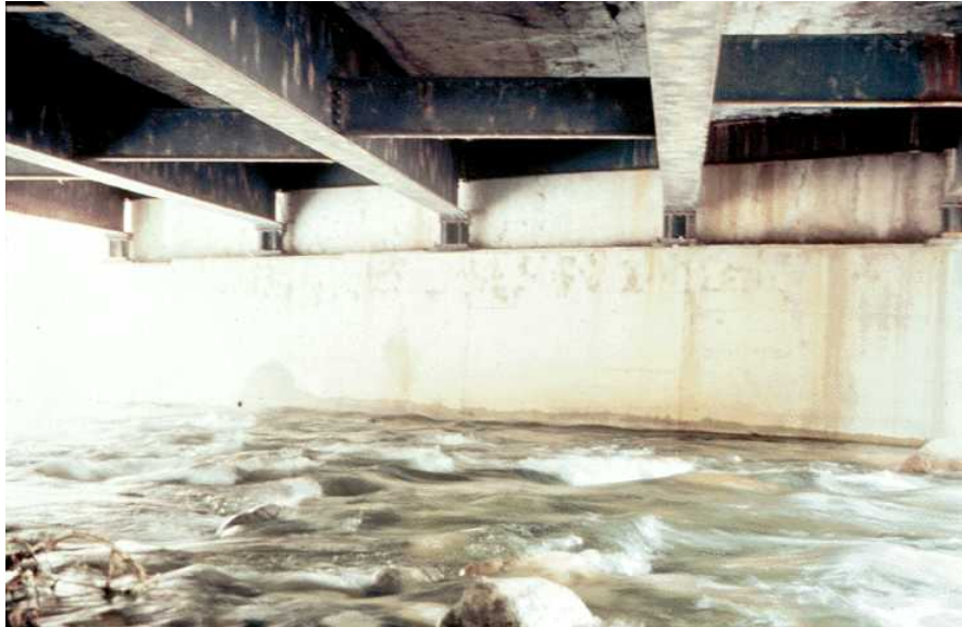
Figure 2.35 Diaphragms on Skewed Bridge
