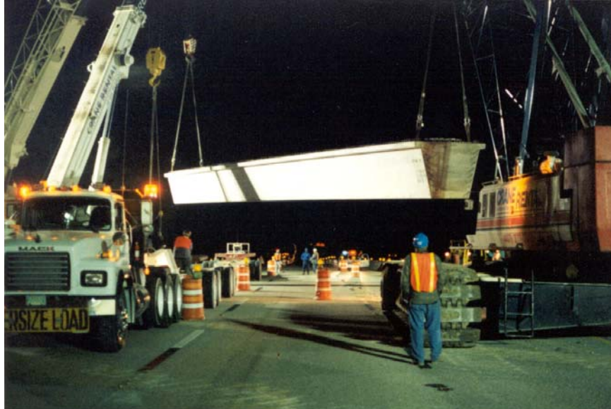
Figure 1.20 Erection using Two Cranes
