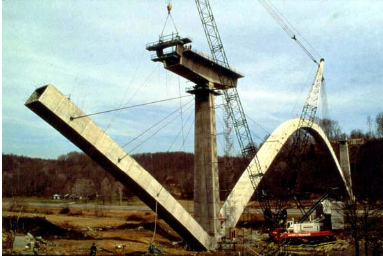
Figure 2.70 Precast Segmental Arch (600 foot span)
