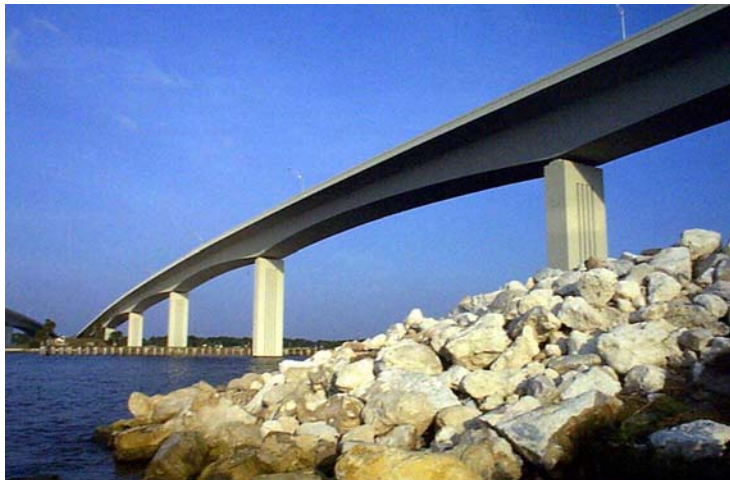
Figure 2.67 Precast Segmental Balanced Cantilever (spans 150 to 500 feet)
