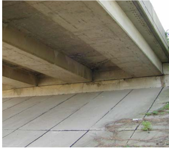
Figure 2.11 Stub Abutment (Longer Span)
