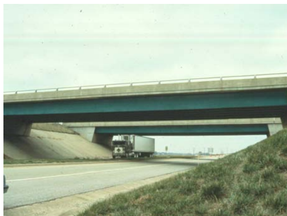
Figure 2.32 Fabricated Girder Superstructure
