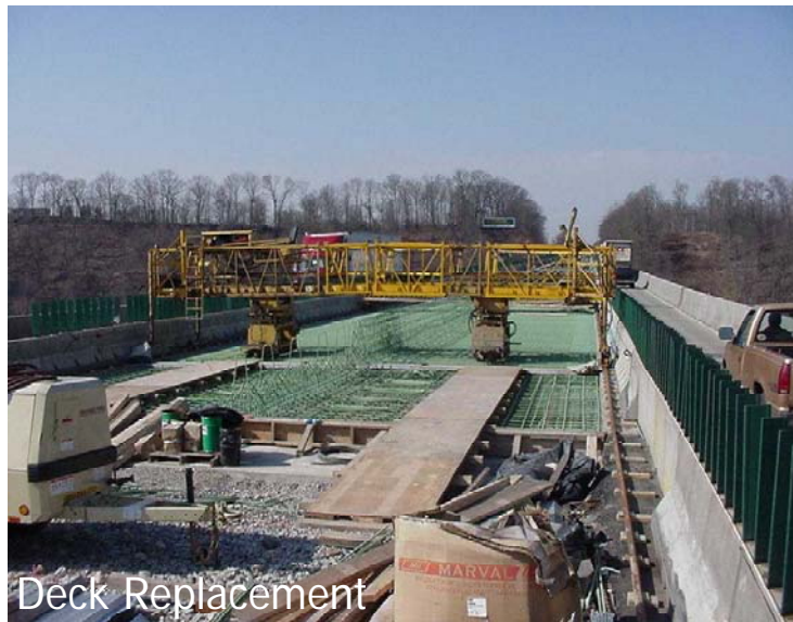
Figure 2.16 Conventional Deck Replacement Under Traffic
