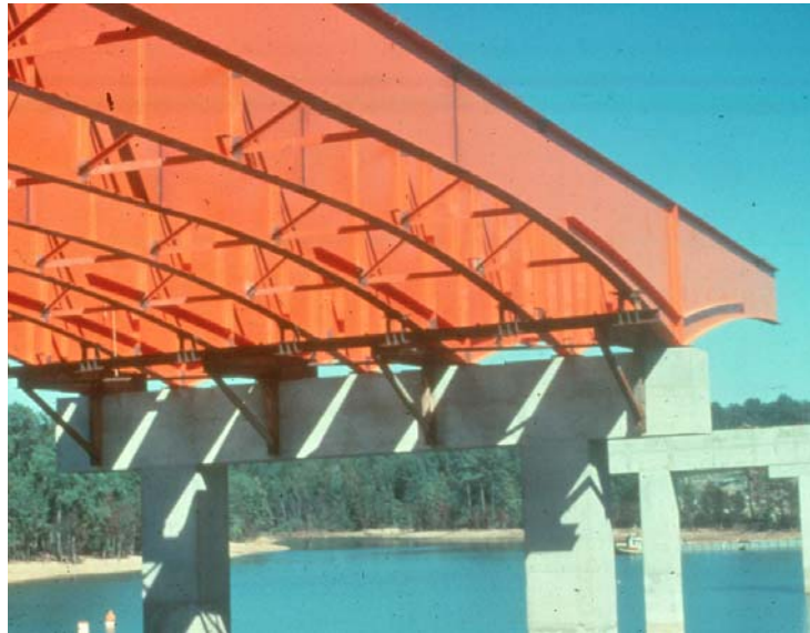
Figure 2.28 Variable Depth Girders
