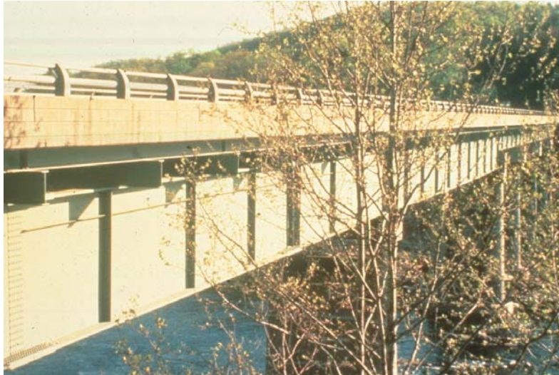
Figure 2.80 Transverse Web Stiffeners
