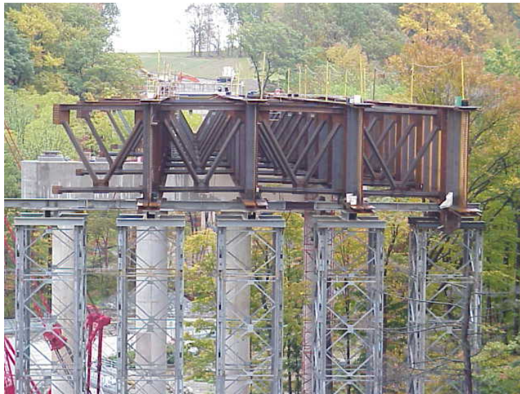
Figure 2.34 Cross Bracing During Construction
