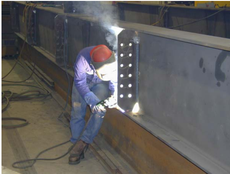
Figure 2.44 Shop Welding of Diaphragm Connection Plate
