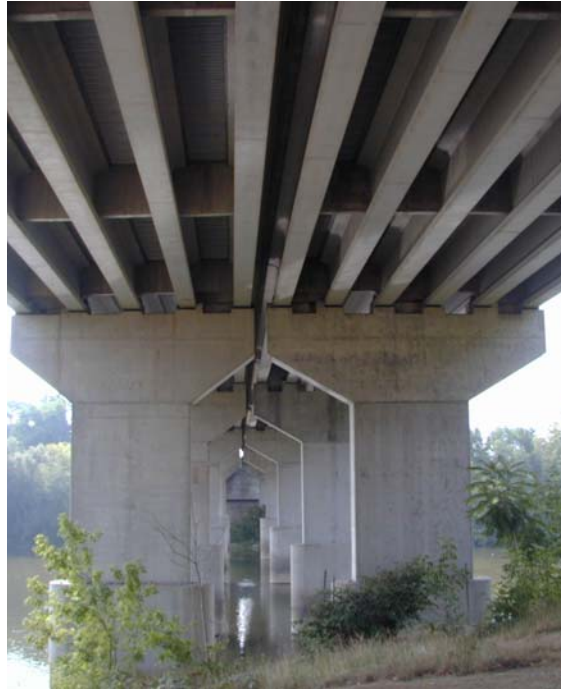
Figure 2.12 Hammerhead Piers
