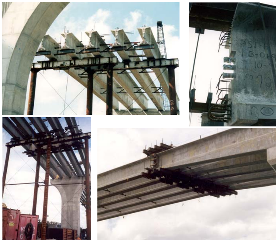
Figure 1.3 Temporary Falsework for Spliced Girder Construction
