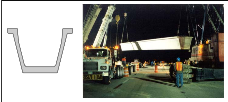
Figure 2.64 U-Beam (spans 50 to 125 feet)
