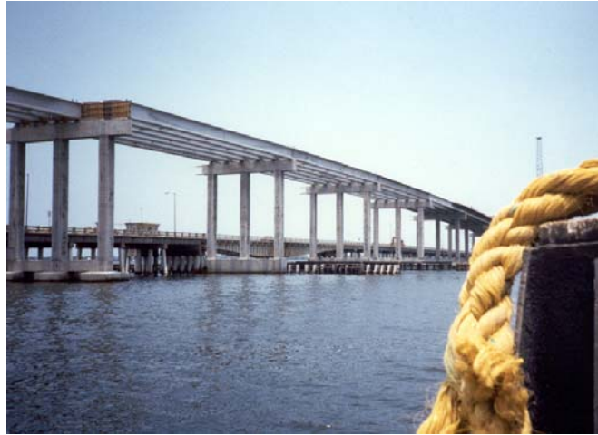
Figure 2.62 Precast Pretensioned I-Girders (spans from 40 to 140 feet)
