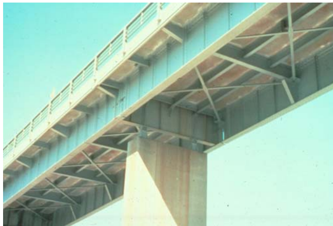
Figure 2.58 Deck-Type Two-Girder System
