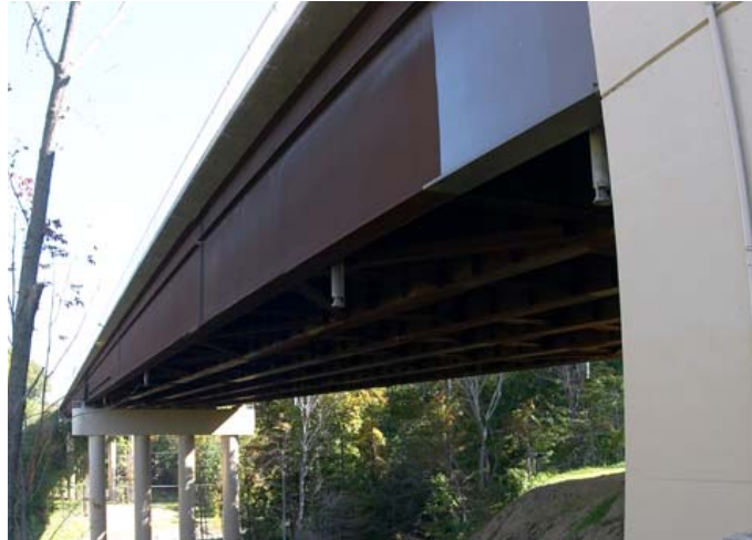
Figure 2.10 Girder with Longitudinal Stiffeners
