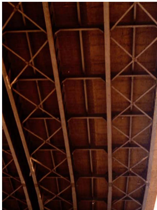
Figure 2.47 Lateral Bracing
