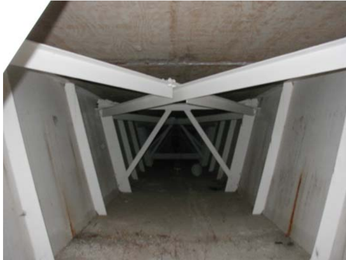
Figure 2.9 Interior of Box Girder with Inclined Webs
