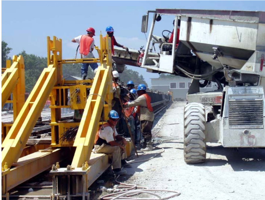
Figure 1.17 Placing and Consolidating Concrete
