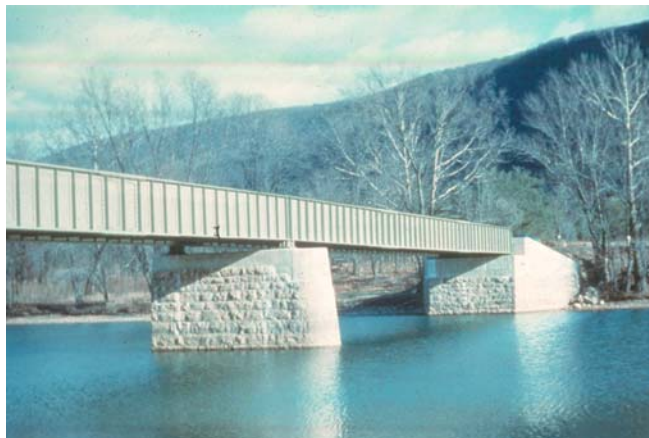
Figure 2.59 Through-Type Two-Girder System
