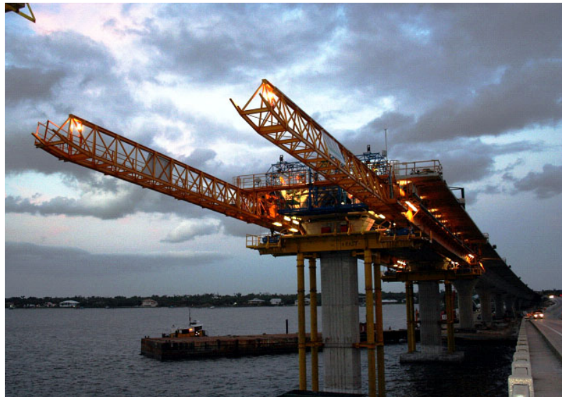
Figure 1.4 Span-by-Span Construction using Erection Trusses
