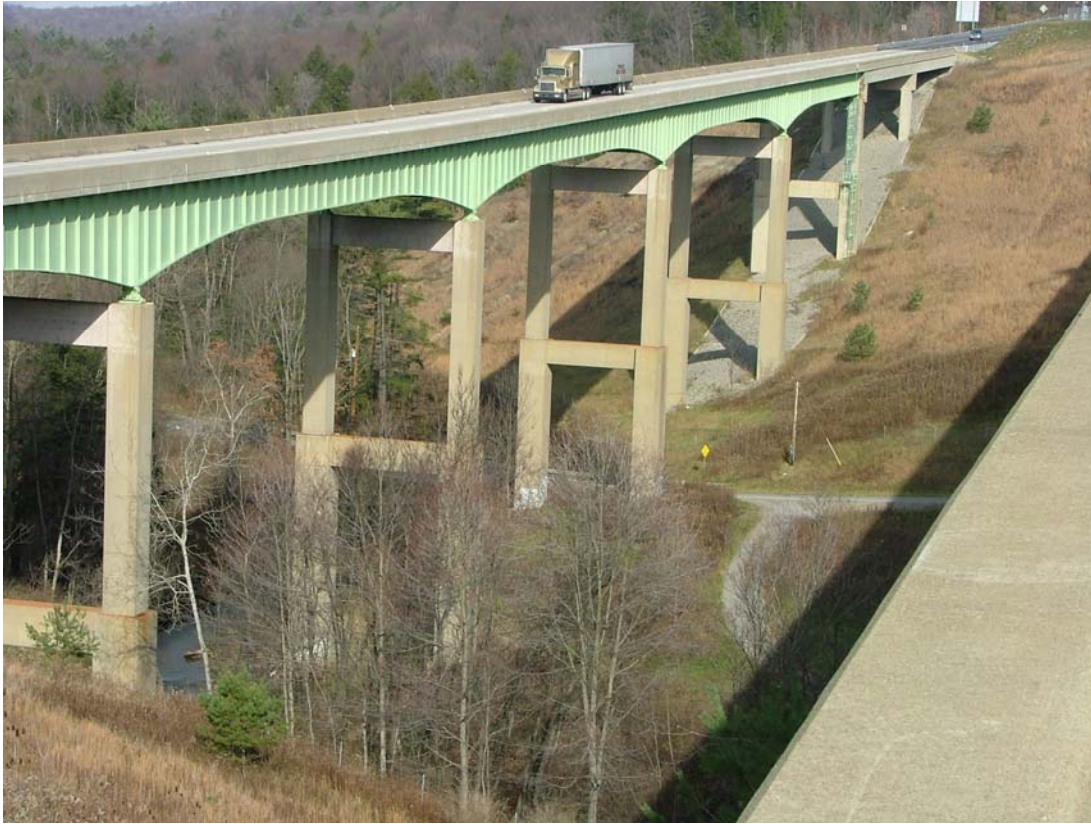
Figure 2.6 Haunched Girders Can Improve the Aesthetics of the Bridge
