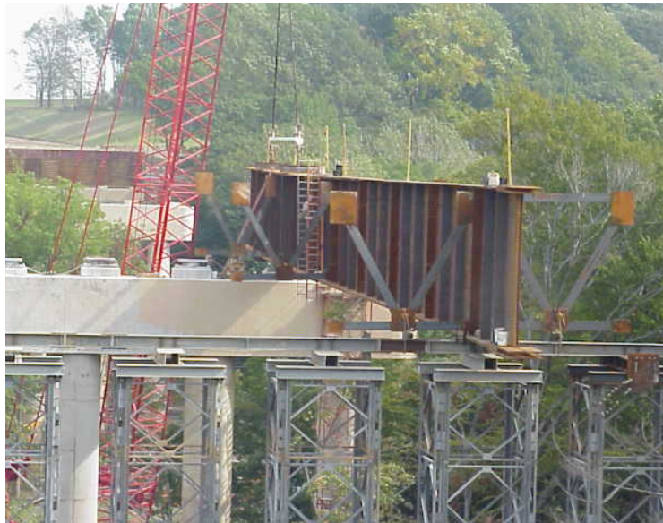
Figure 2.27 Bridge Girder Erection
