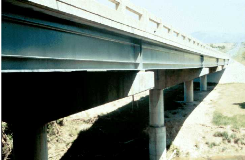
Figure 2.86 Longitudinal Web Stiffeners
