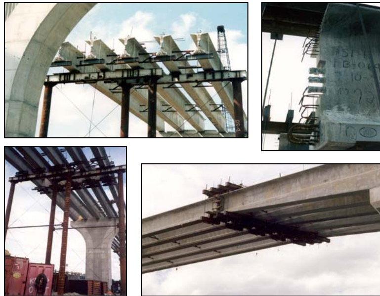
Figure 1.34 Construction of Haunched Spliced Girders
