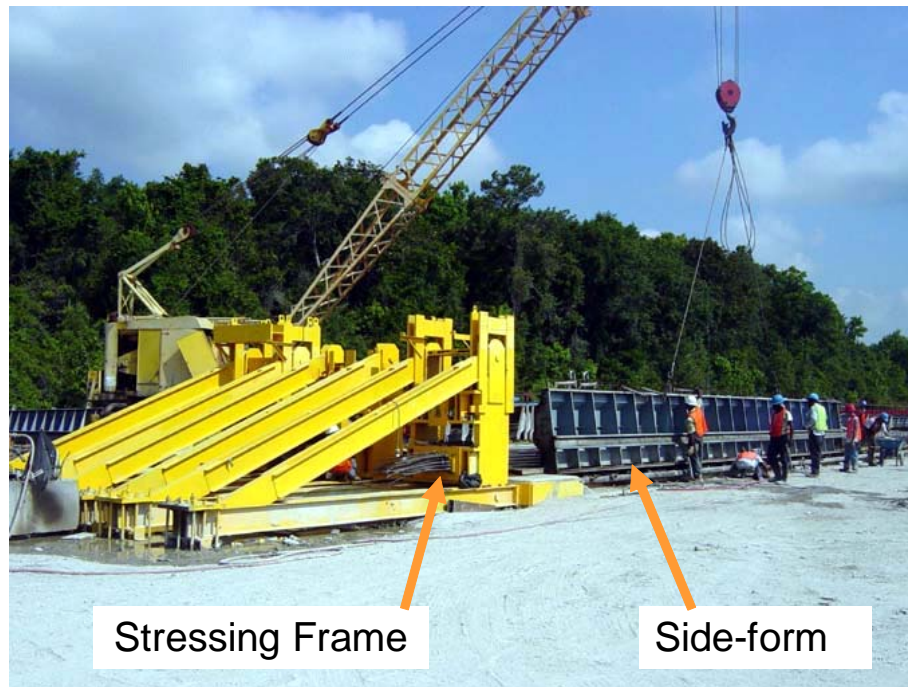
Figure 1.16 Stressing Frame and Side Forms
