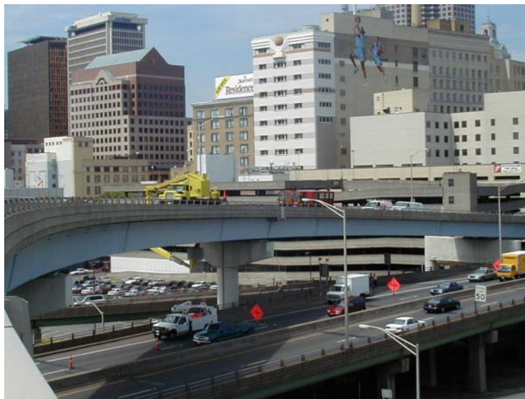
Figure 2.8 Continuous Span Steel Bridge
