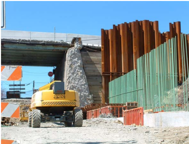
Figure 2.17 Phased Construction
