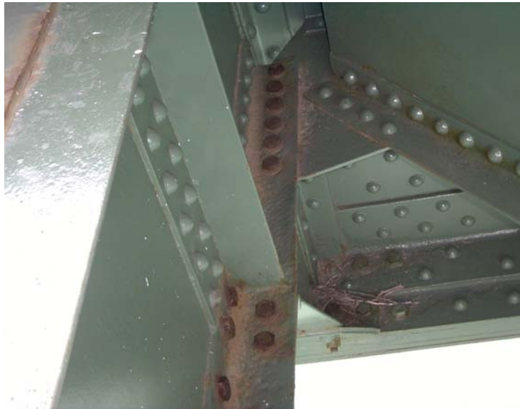
Figure 2.51 Bolted Gusset Plate
