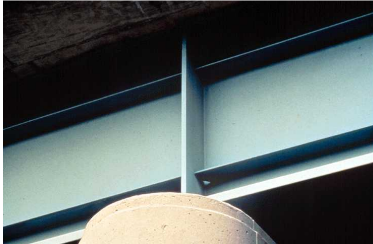
Figure 2.82 Bearing Stiffener
