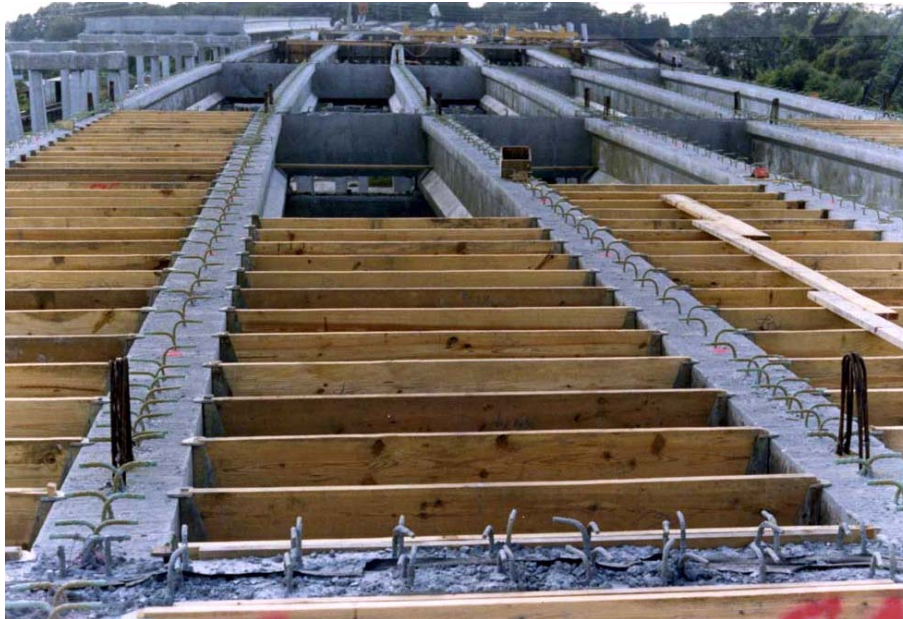
Figure 1.25 Lumber Joists to Support Plywood Formwork
