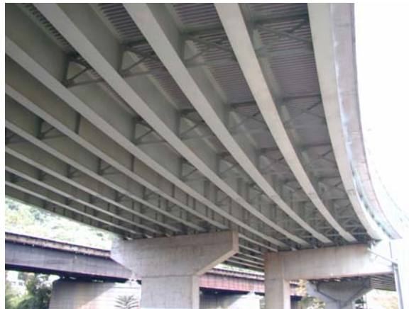
Figure 2.46 X-Type Cross Frame Configuration
