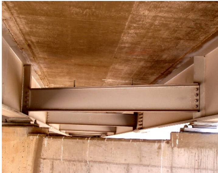
Figure 2.45 Rolled Shape Used as Diaphragm
