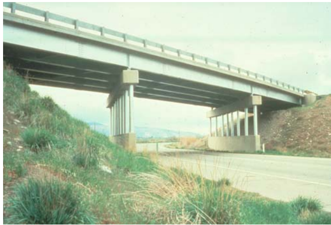
Figure 2.31 Rolled Beam Superstructure
