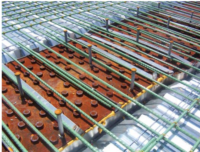
Figure 2.5 Reinforcement and Shear Connectors
