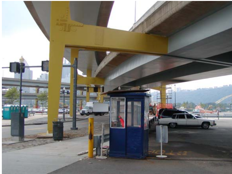
Figure 2.13 Integral Pier Cap
