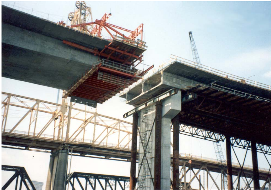
Figure 1.43 Side-Span Falsework for Cast-in-Place Box (Acosta Bridge)
