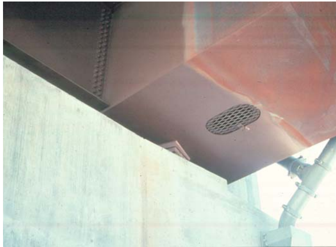
Figure 2.4 Inspection Access in Box girder Bottom Flange
