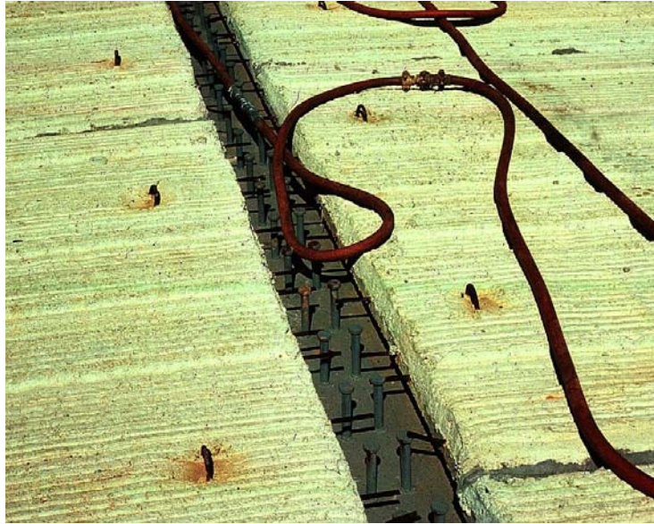
Figure 2.15 Precast Concrete Deck Panels
