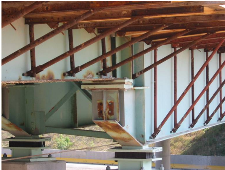
Figure 2.34 Deck Overhang
