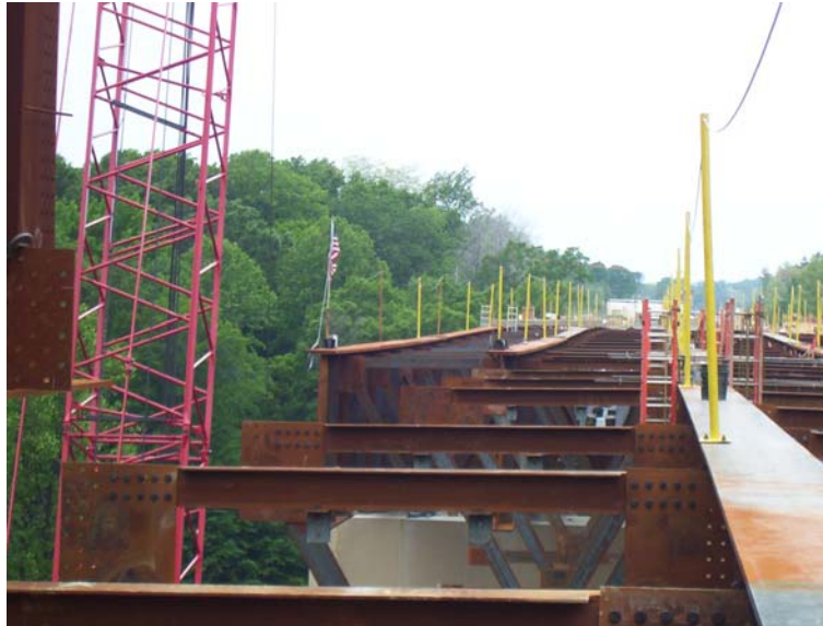
Figure 2.37 Cross-Frame Connections to Girder Top Flange
