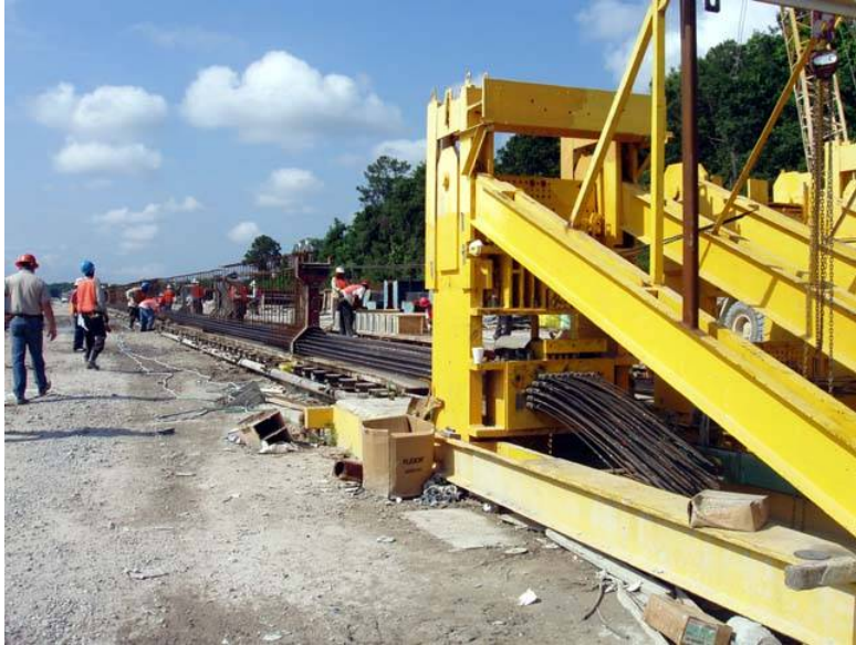
Figure 2.5 Casting Bed for Pretensioned Girders
