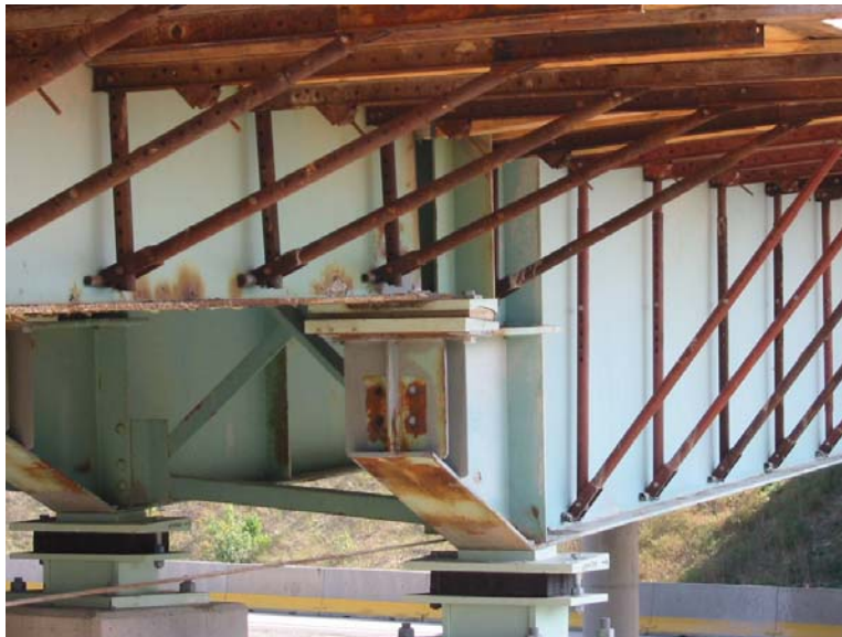
Figure 2.18 Cantilevered Forming Brackets
