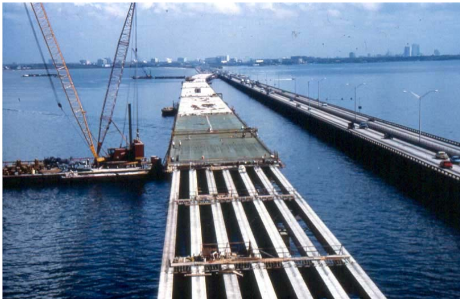
Figure 1.21 Crane on Barge
