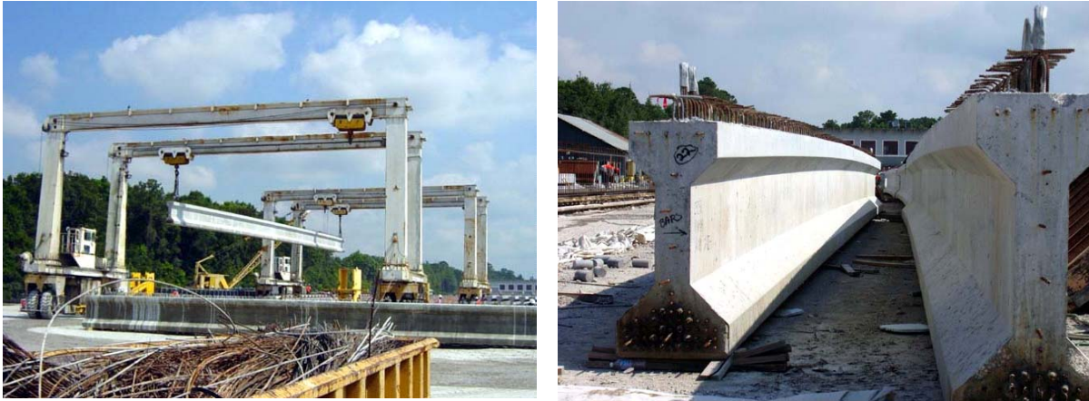
Figure 1.18 Handling and Storage of Girders in Casting Yard
