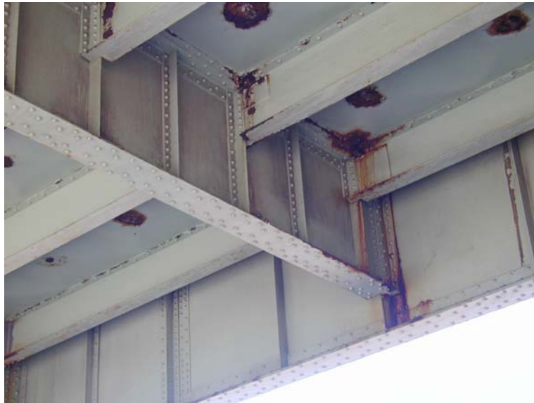
Figure 2.52 Riveted Girder and Floorbeam with Rolled Stringers
