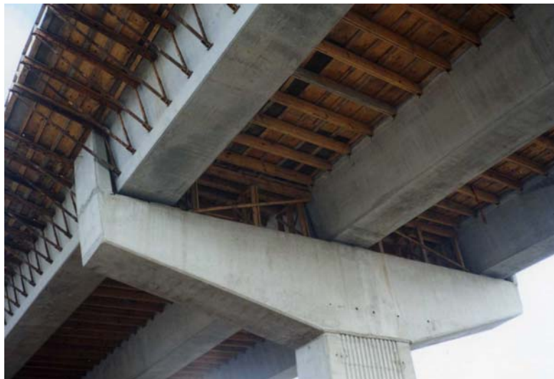
Figure 1.28 Lumber Form System for Widely Spaced U-Beams
