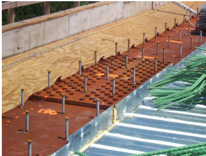
Figure 2.1 Steel Girder with Stud Shear Connectors
