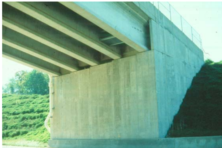
Figure 2.10 Full Height Abutment (Shorter Span)
