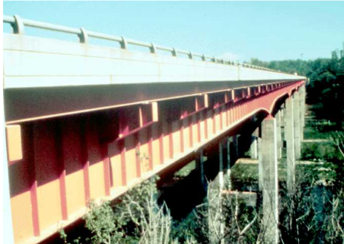
Figure 2.8 Continuous Steel Girder Bridge
