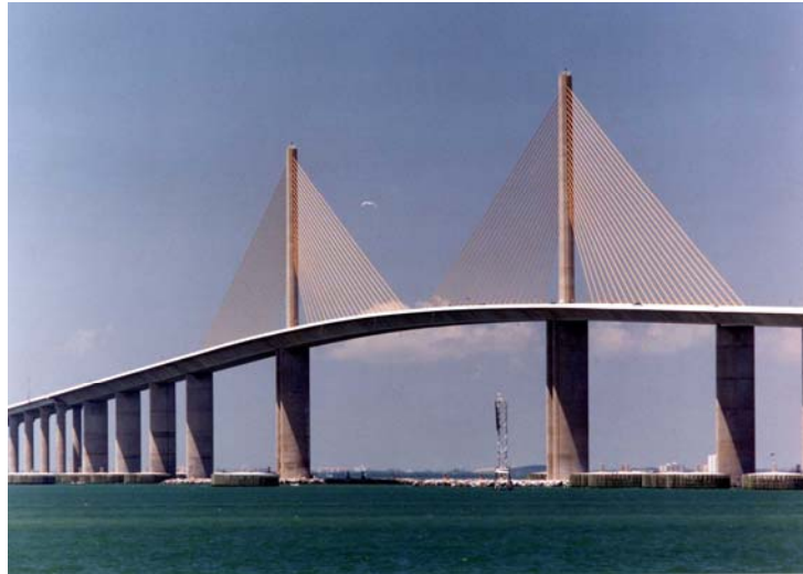
Figure 2.69 New Sunshine Skyway, Precast Segmental Cable Stay (1,200 foot span)
