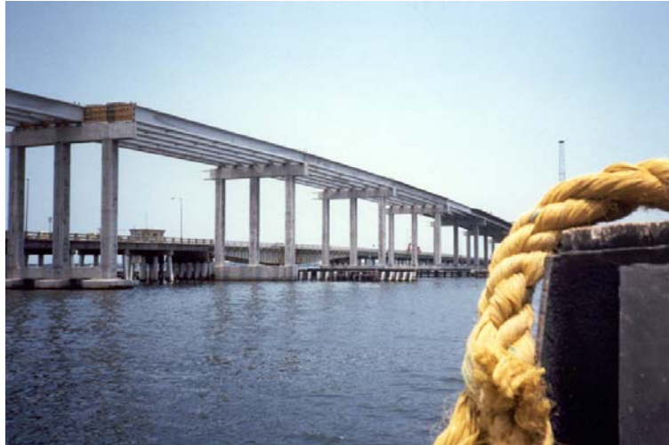
Figure 1.33 4-Span Continuous Precast Spliced Girder Construction
