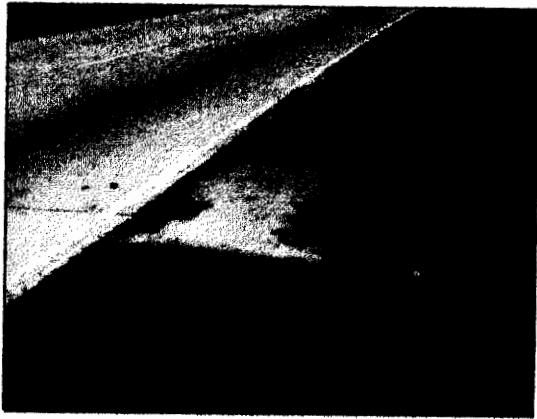
Pumping Stains on Shoulder
