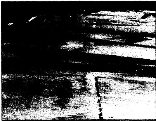
Jumbled Pavement Slabs
