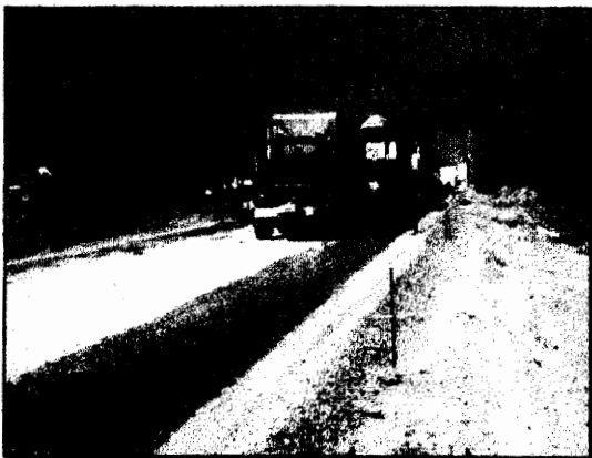
Delivery Trucks Running on Permeable Base
