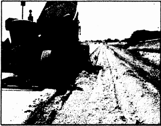
Backfilling Edgedrain Trench
