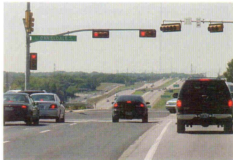
In addition to traffic signalization improvements, CMAQ funds were used to add a right-turn lane at Daniel Dale Road to further mitigate congestion.
