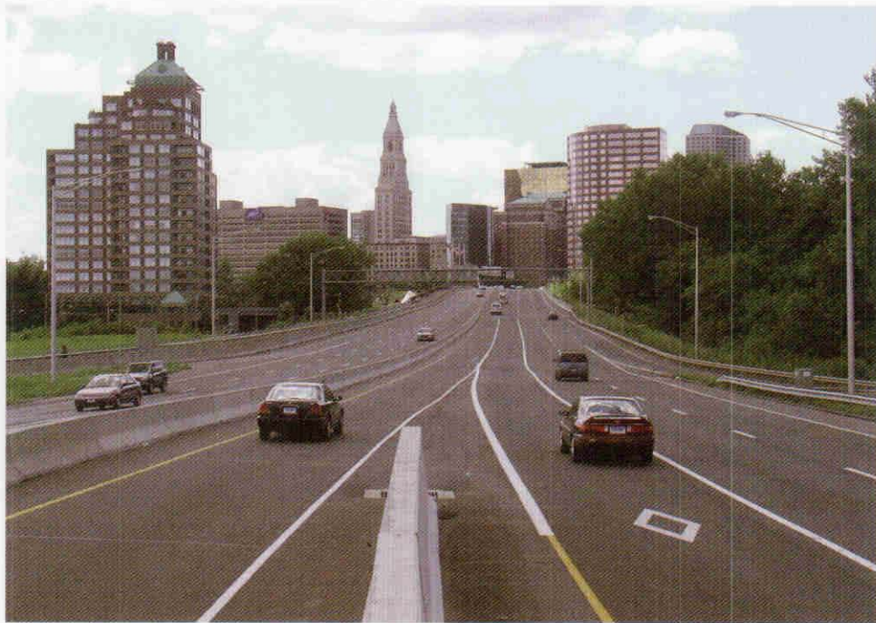
Drivers head west in the HOV lane from East Hartford toward the Founders Bridge.
