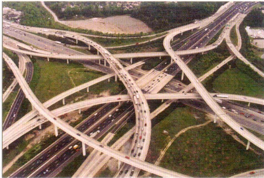
I-85 and I-285 intersection north of Atlanta.
