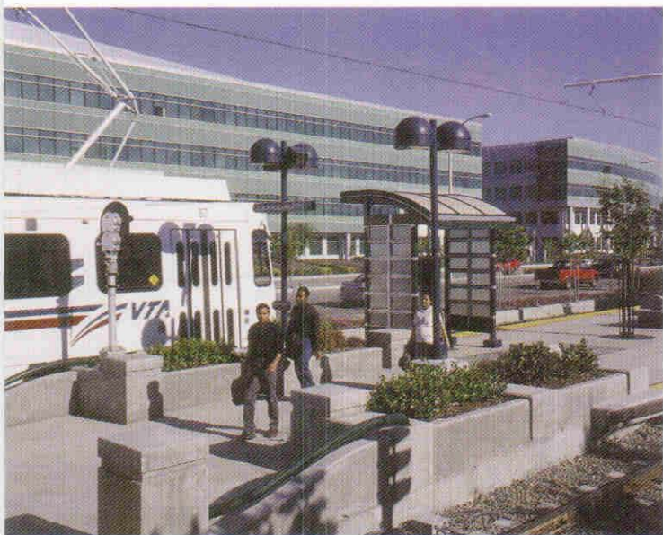
VTA station on the Tasman Corridor line.
