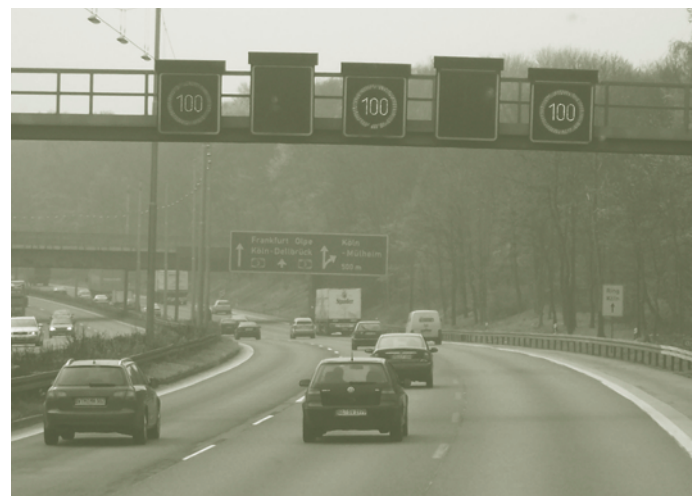
Figure 11. Example of variable speed limit in Germany
