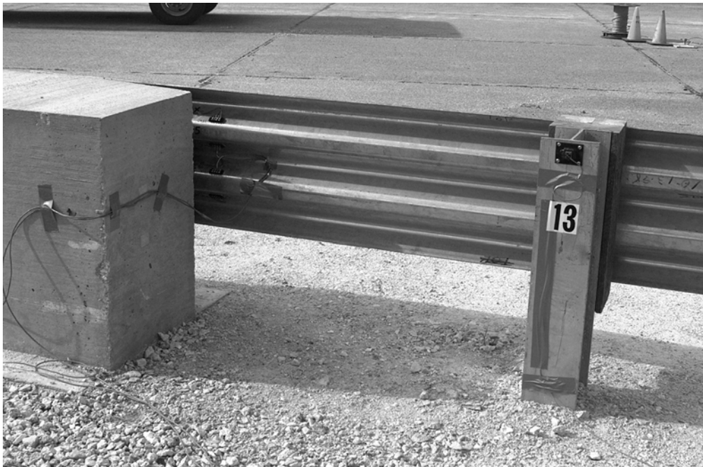
b) Transition from field side.
