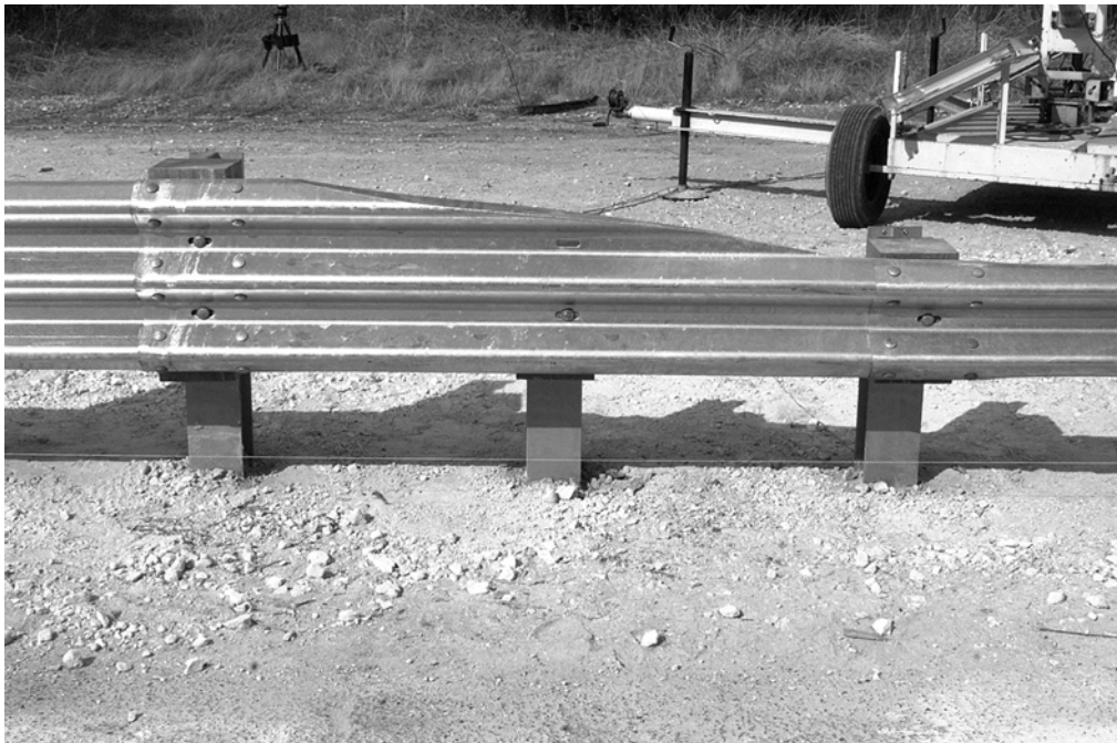
b) Closeup view of transition section.
