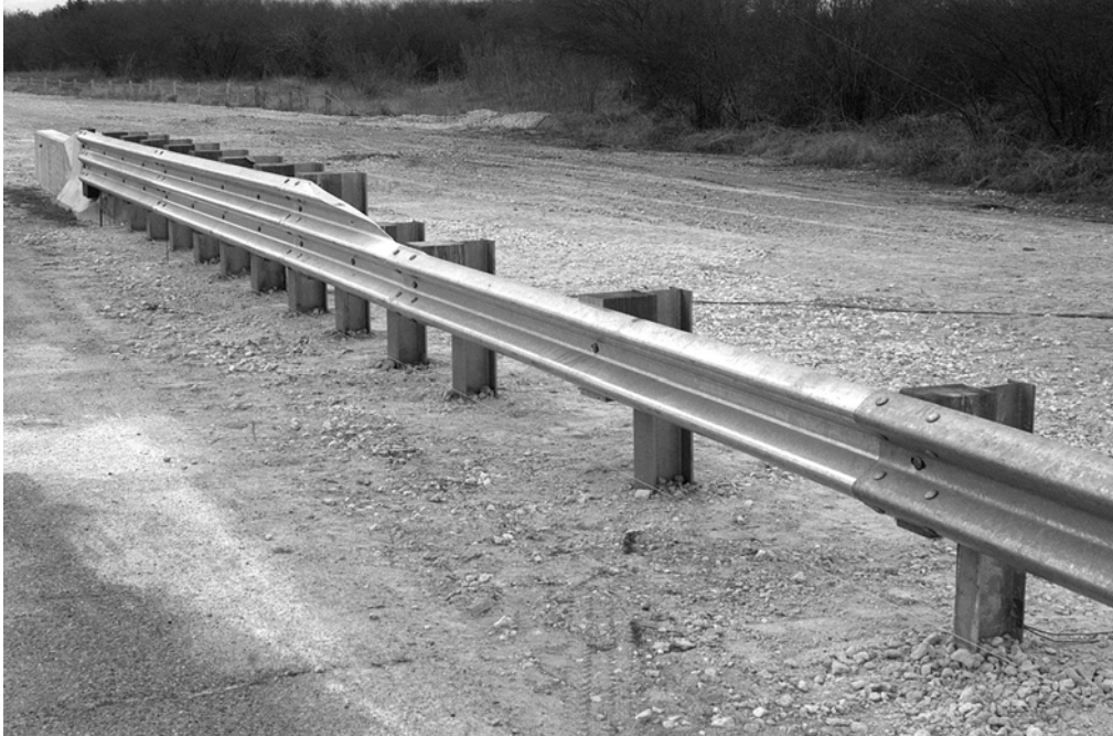
a) Overall view of transition from traffic side.
