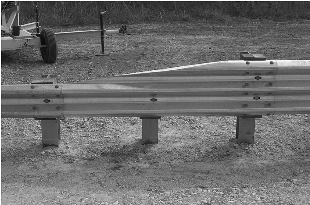
b) Closeup view of Ohio transition section.
