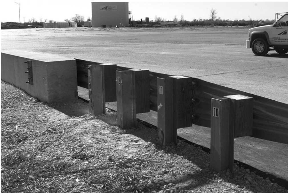
b) Transition from field side.
