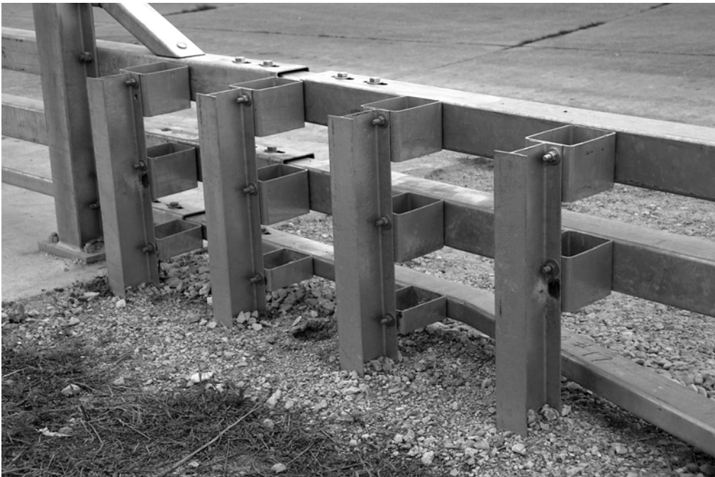
b) Field side of transition section.
