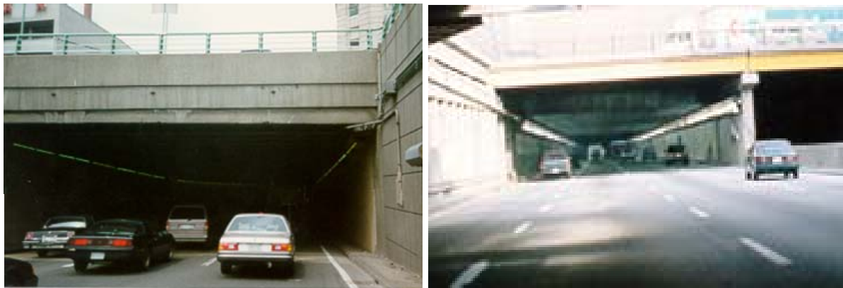
Figure 2-7 “Black Hole” (Left) and Proper Lighting (Right)
