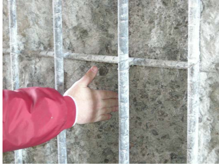
Figure 16-7 Substrate after Hydro-demolition, Shawmut Jct. Boston
