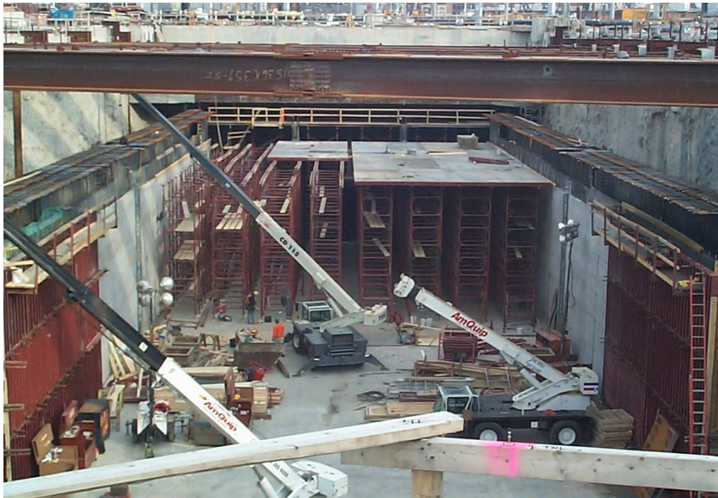
Figure 12-4 Tunnel Structure Construction Operation
