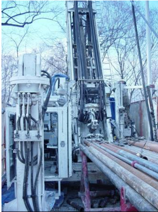
Figure 3-6 Horizontal Borehole Drilling in Upstate New York
