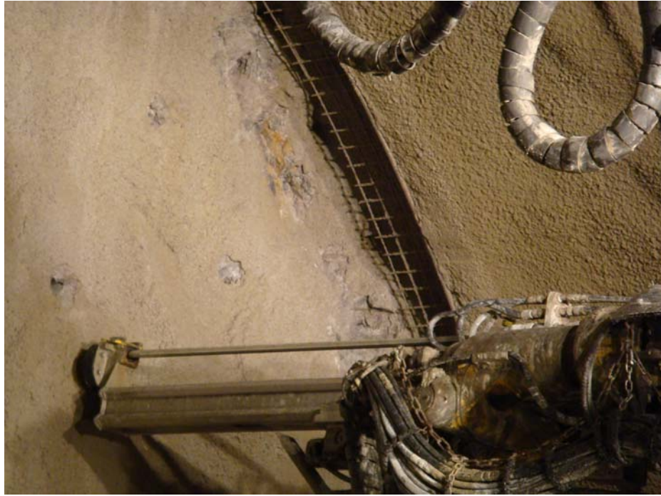
Figure 9-11 Shotcrete Lining Installed at the Face in a SEM Tunnel Excavated by Drill-and-Blast (Andrea Tunnel, Austria)
