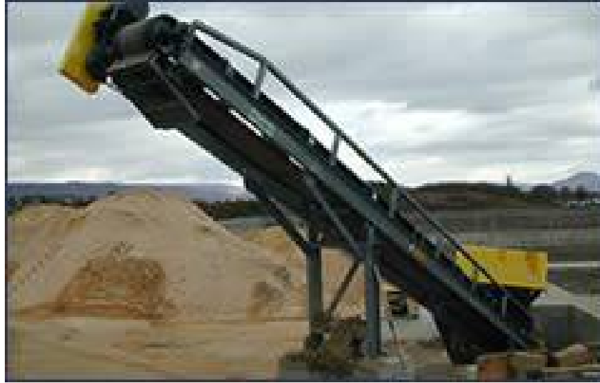
Figure 14-5 Surface Muck Storage Area
