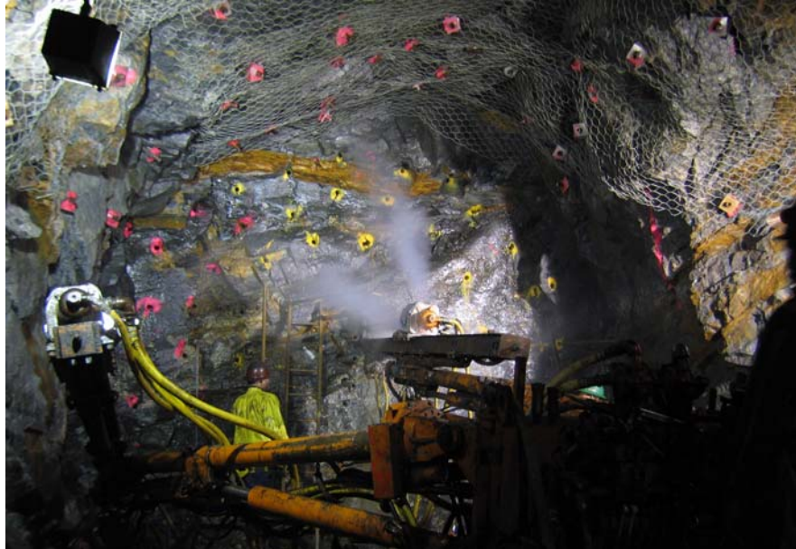
Figure 6-8 Drilling for a Tunnel Blast
