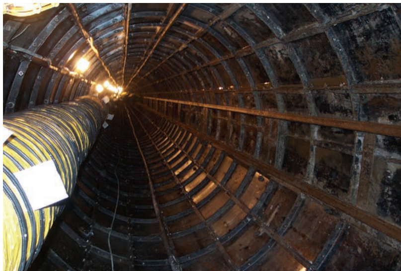
Figure 10-3 Baltimore Metro Steel Plate Lining
