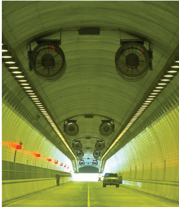
Figure 10-1 Cumberland Gap Tunnel
