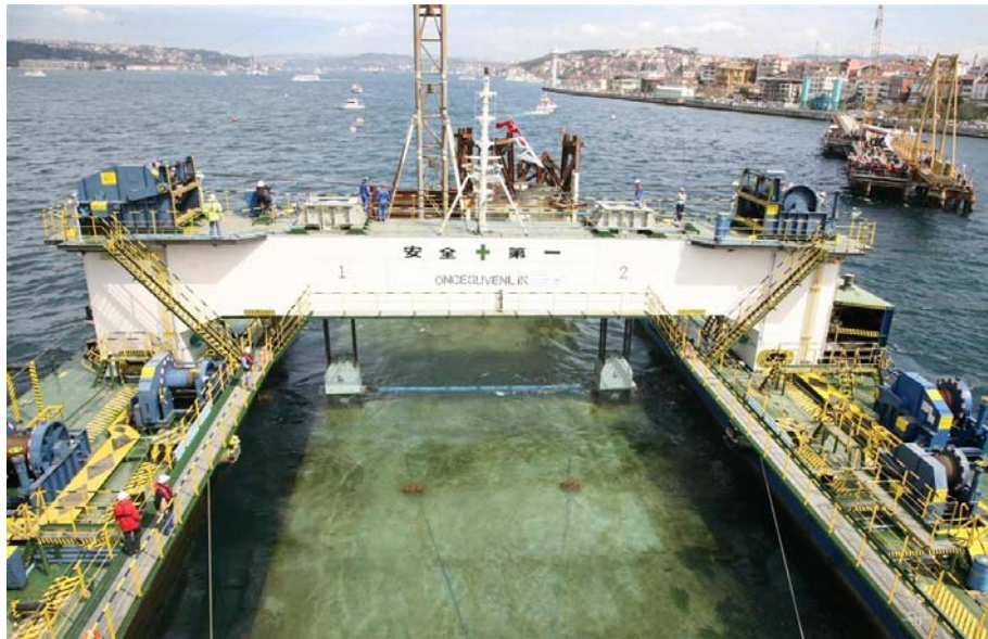
Figure 11-15 A Tunnel Element is Being Placed.
