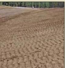
**Figure 10.12** – An alternative form of imprinting road cuts and fills that does not compact soils is welding angle iron onto the bucket of an excavator. As the excavator pulls topsoil into place and contours the slope, it presses the face of the bucket into the soil surface to form surface imprints.
