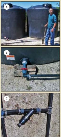
The drip tubing diameter determines the volume of water that can be carried in the lateral lines and the rate it will be delivered based on friction losses. A two inch pipe, for instance, carries four times as much water as a one inch pipe, but the costs are correspondingly much higher. For long stretches, increased frictional losses inside narrow diameter pipes can cause inadequate water coverage. Increasing water pressures or increasing pipe diameters can compensate for this.
