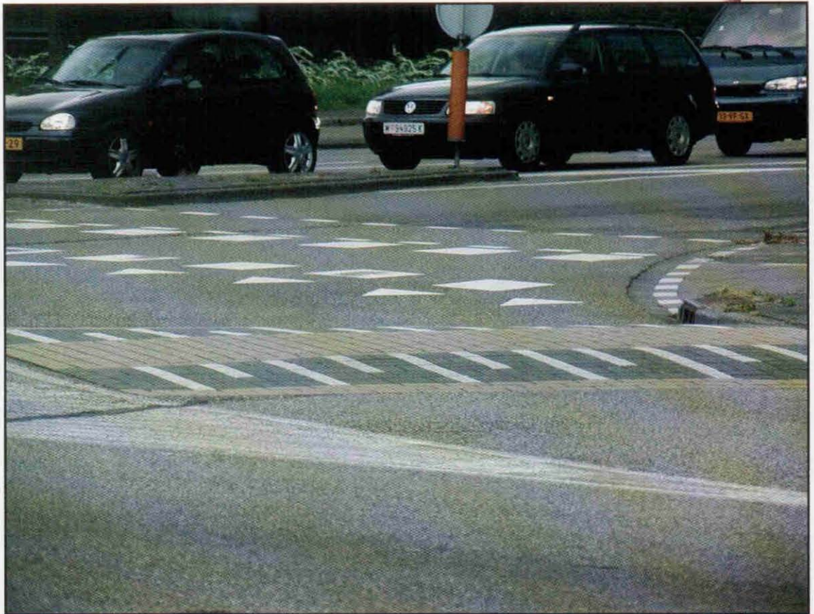
Figures 5-7. Speed table in right-turn lane.
