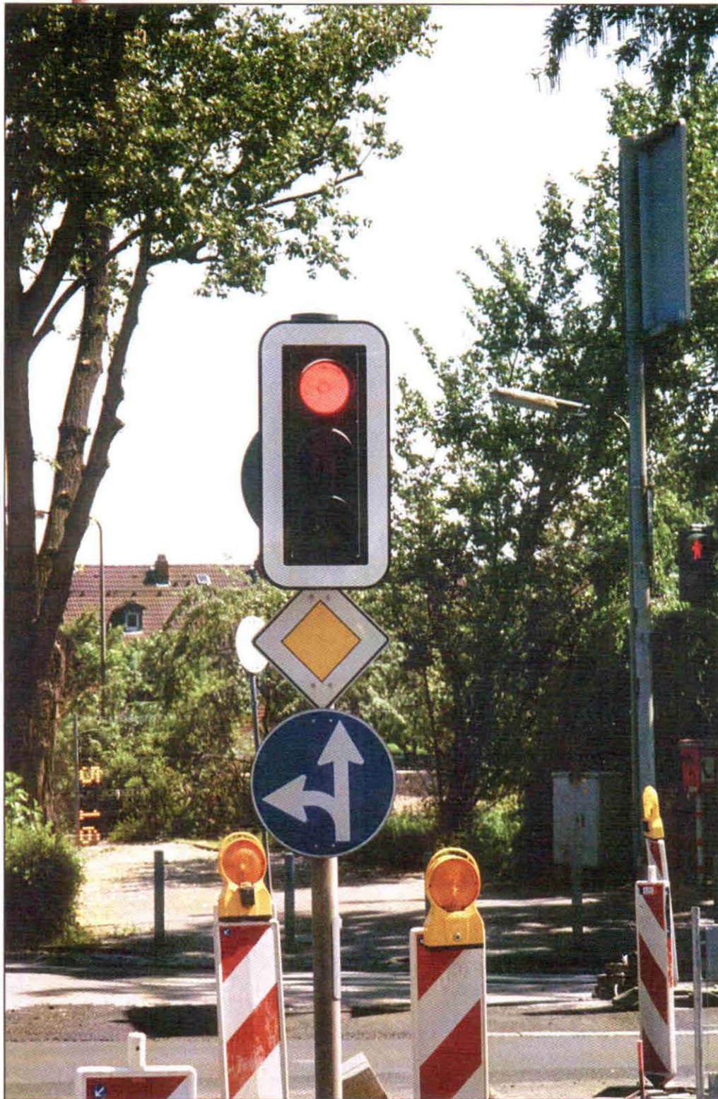
Figure 4-6. Traffic signal with back plate in Germany.
