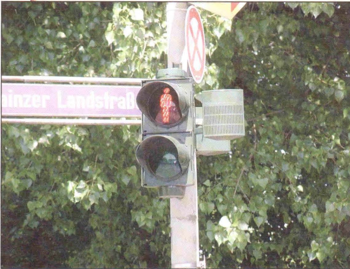
Figure 3-3. Audible pedestrian signal head in Germany.
