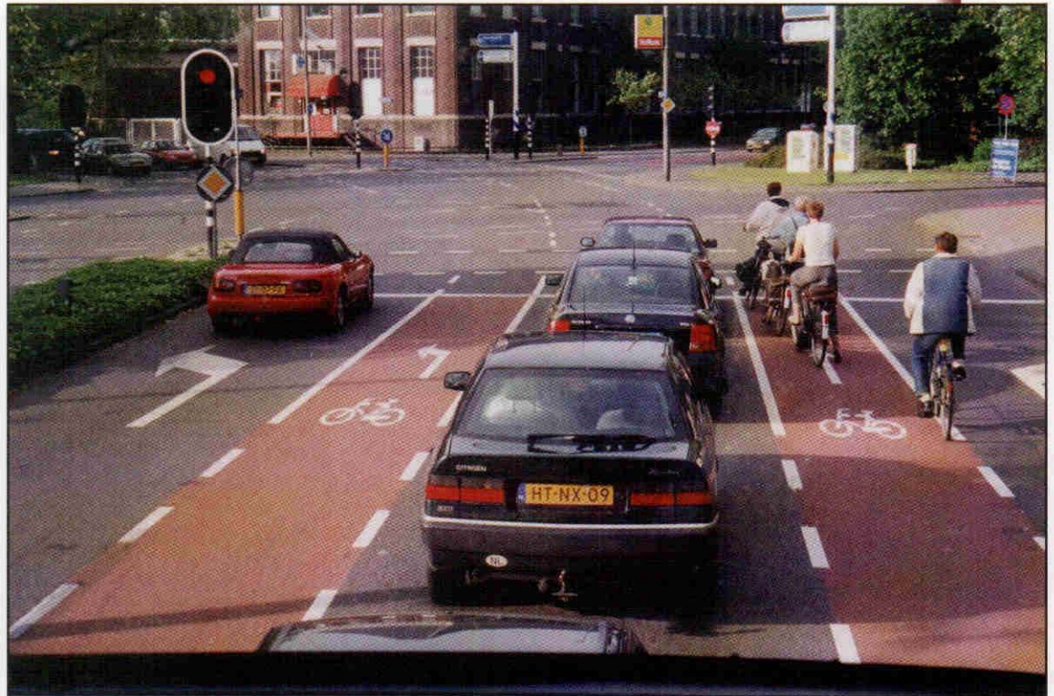
Figure 4-12. Colored pavement used to distinguish bike lanes in the Netherlands.
