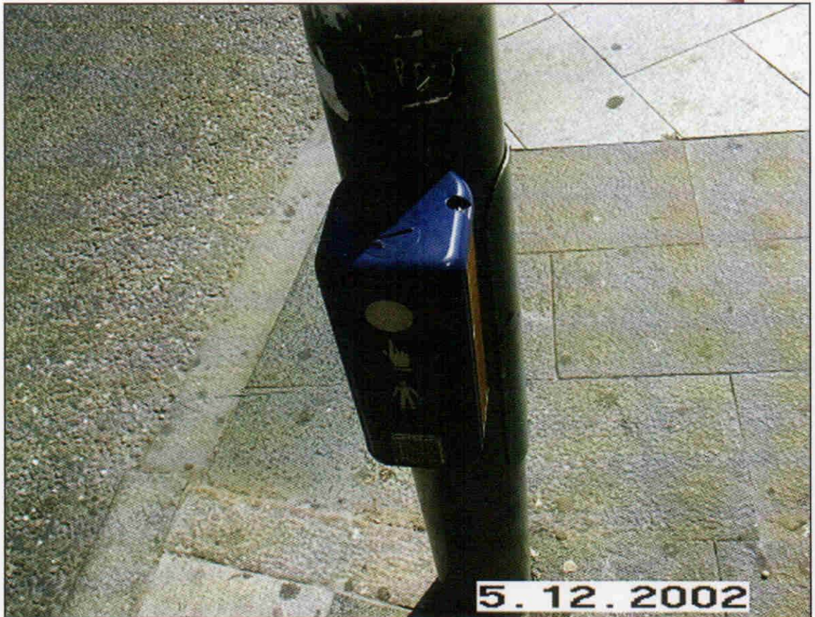
Figure 4-4. Pedestrian push button equipped with acoustic locator tone in Sweden.
