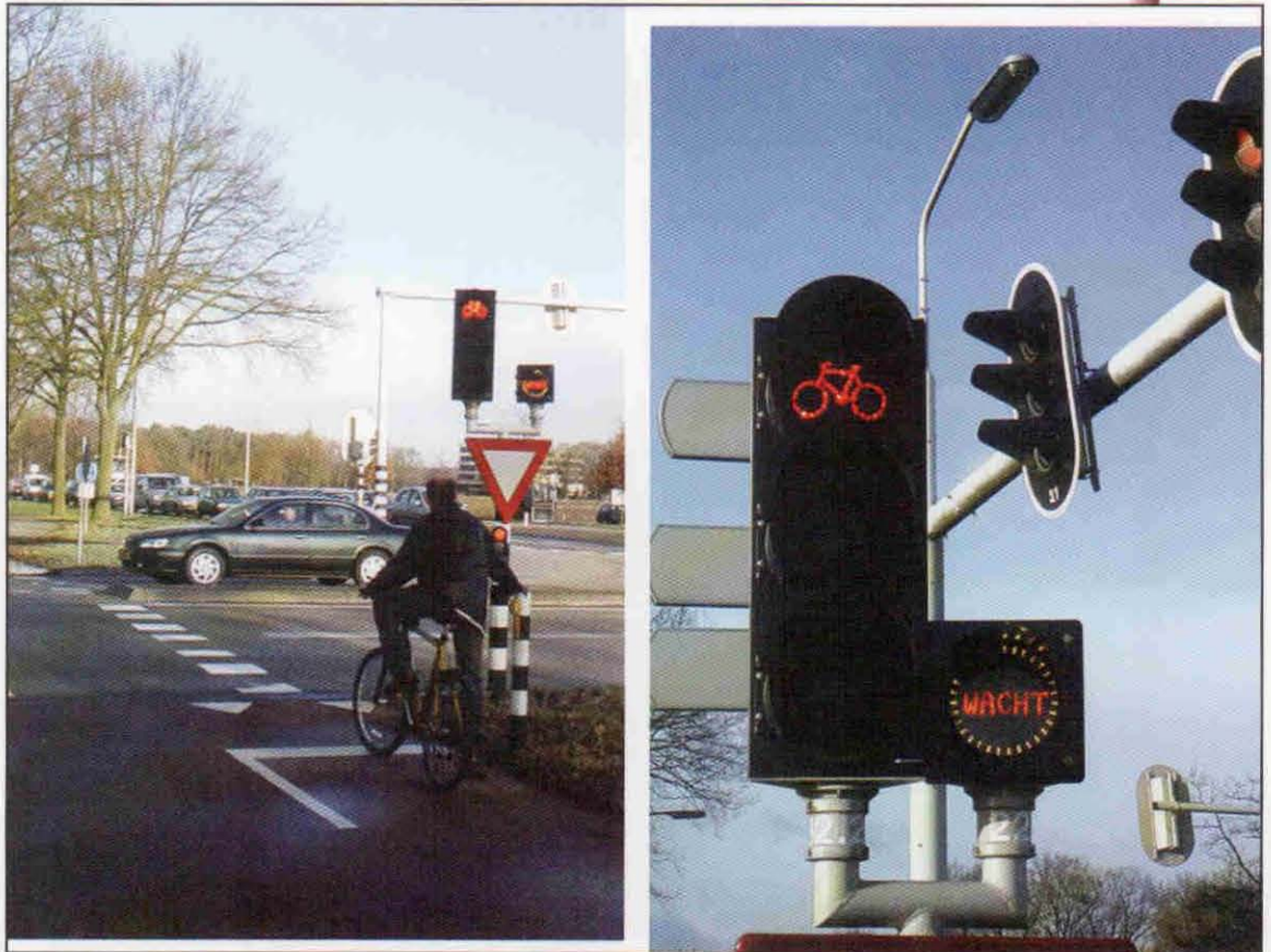
Figure 4-20. Countdown indicator for bicycle crossing.
