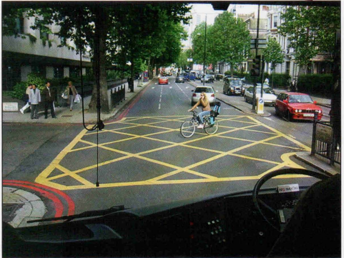
Figure 4-26. Yellow crosshatched intersection in the United Kingdom.
