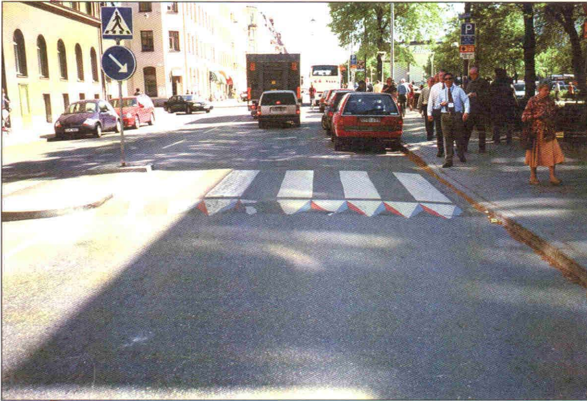
Figure 4-5. Virtually raised crosswalks in Sweden.
