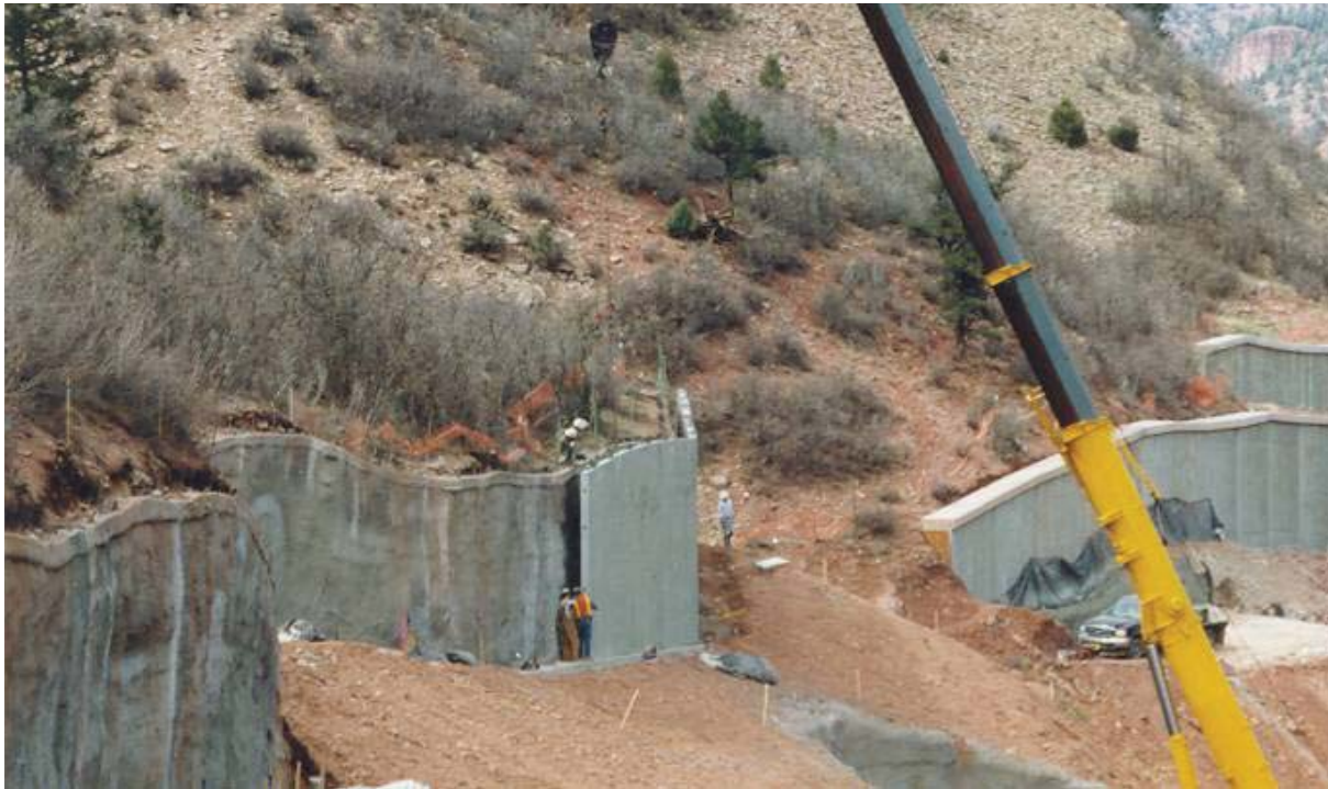
Figure 1. Photo. Installation of a permanent pre-cast concrete facing over a structural shotcrete soil wall.
