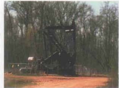
Oil pump station on Anderson Tract
