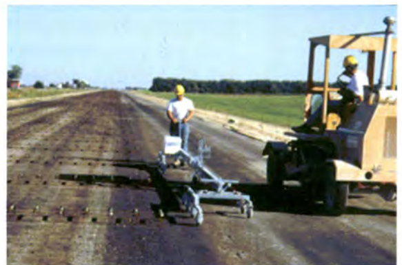
Figure 11. Contractor checking profile of trackline prior to paving.
