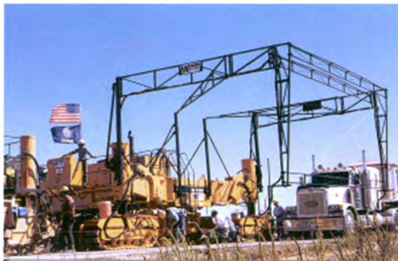
Figure 10. PCC paver with offset stringline.
