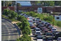
Traffic backed up on NB Wadsworth prior to the project. Restaurant (blue roof) had to be relocated.
