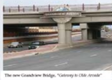
The new Grandview Bridge, "Gateway to Old Arvada"
