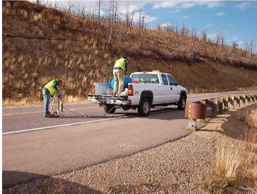
Figure 45. Photo. Coring at Site 4.
