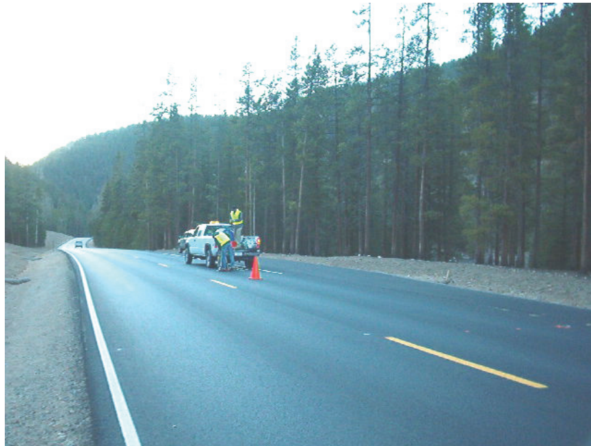
Figure 40. Photo. View of Site 3.
