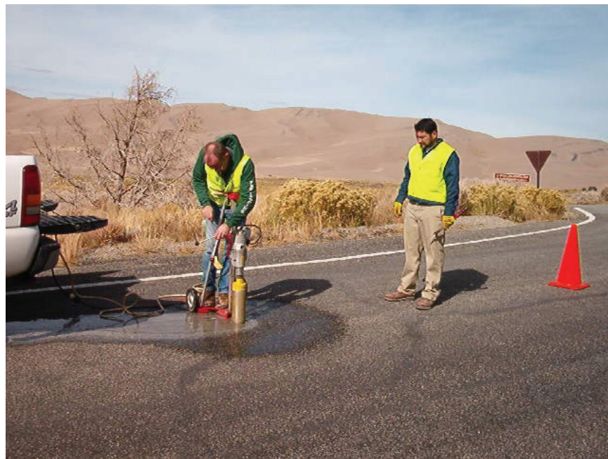
Figure 36. Photo. Coring at Site 2.
