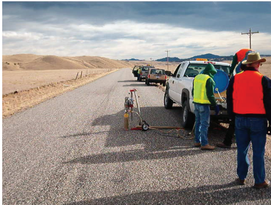
Figure 34. Photo. Coring at Site 1.
