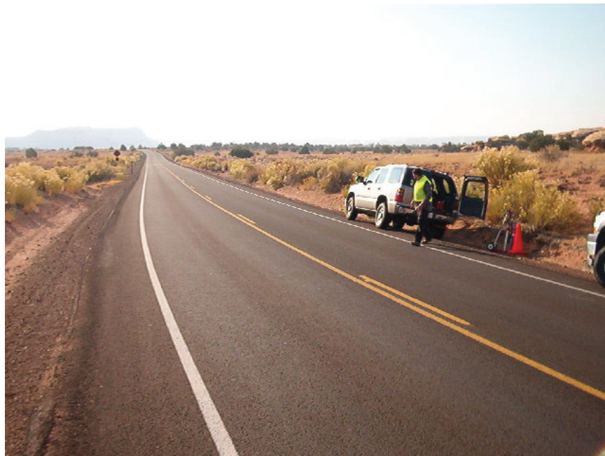
Figure 48. Photo. View of Site 5.
