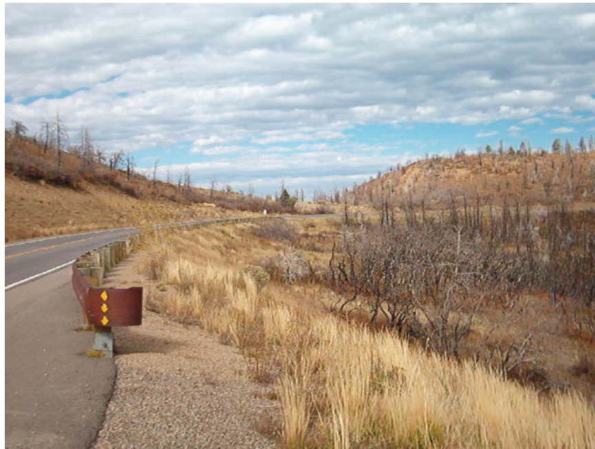
Figure 44. Photo. View of Site 4.
