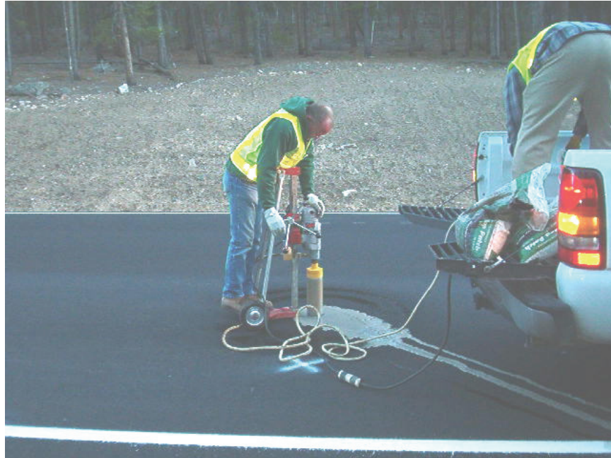
Figure 41. Photo. Coring at Site 3.
