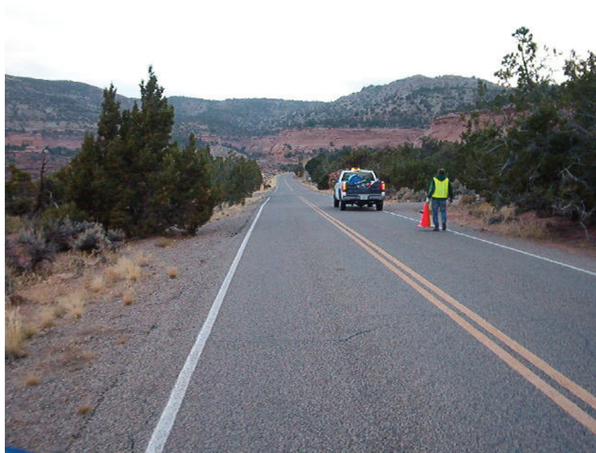
Figure 53. Photo. View of Site 6.
