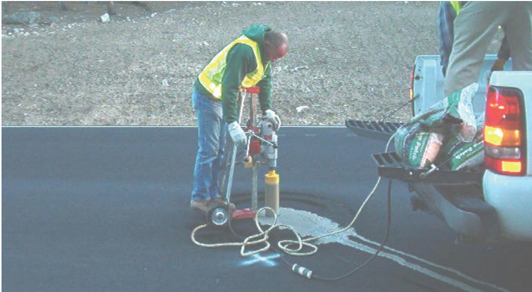
Figure 20. Photo. Typical Coring Operation by CFLHD Staff.
