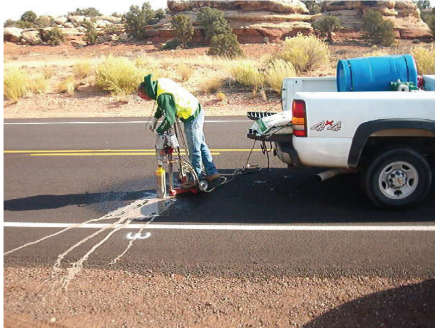
Figure 49. Photo. Coring at Site 5.
