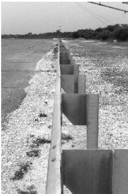
Figure 74. Modified three beam guardrail installation prior to test 404211-5.
