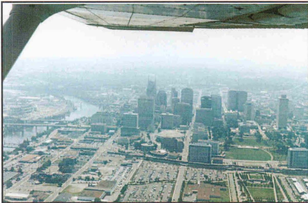
Figure 3.5 Aerial view of Nashville, looking east. The experimental site is to the north (left), just out of the picture.
