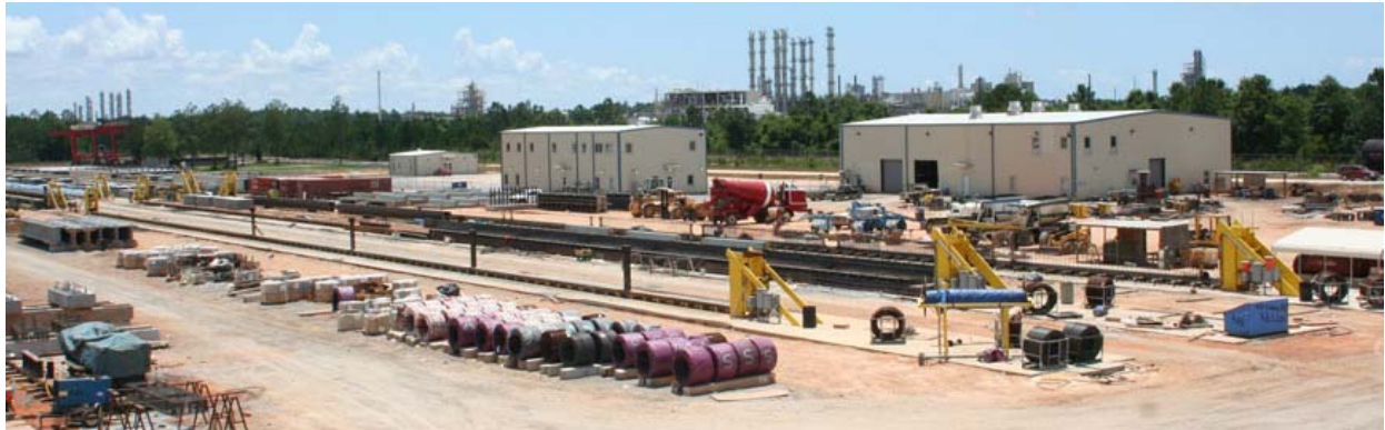
Figure 1. Photo. Prestress fabrication plant for the LWC girders and splice beams.
