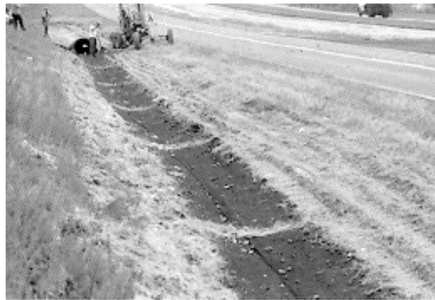
Figure 31. Installed synthetic mat channel lining.
