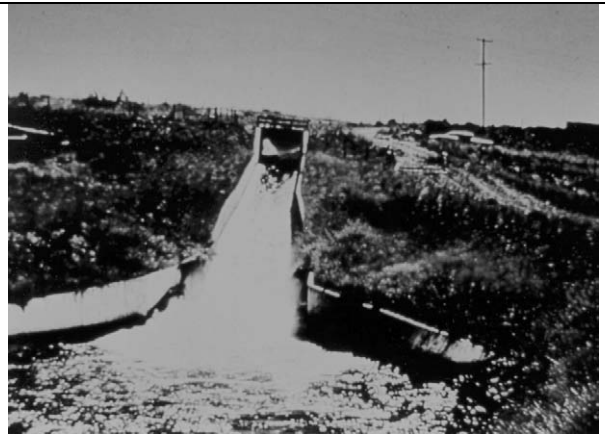
Figure 50b. SAF stilling basin.
