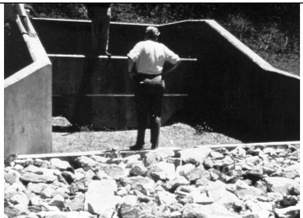
Figure 51b. Baffle-wall energy dissipator - USBR Type VI.
