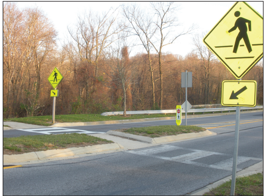
Figure 3: Unsignalized, midblock, ladder crosswalk. Usage of “State Law Stop for Pedestrian within Crosswalk” (R1-6) sign in median
