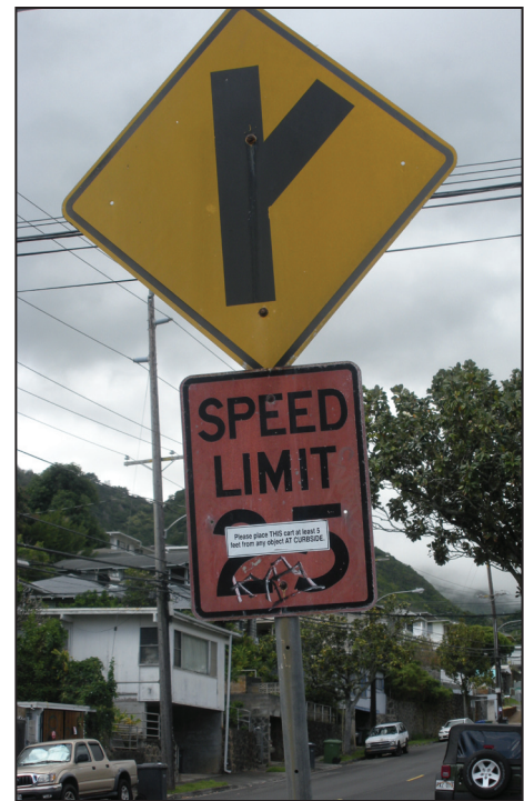
Figure 4: Common Problems 3, 6, 8. The black on orange speed limit is an improper design of a regulatory sign as orange is for temporary traffic control warning sign color. Each message on the sign needs to be placed on separate posts spaced sufficiently apart so that drivers can recognize, read, and process the information and take appropriate action. There is also graffiti on the SPEED LIMIT sign, which is indicative of poor maintenance.
