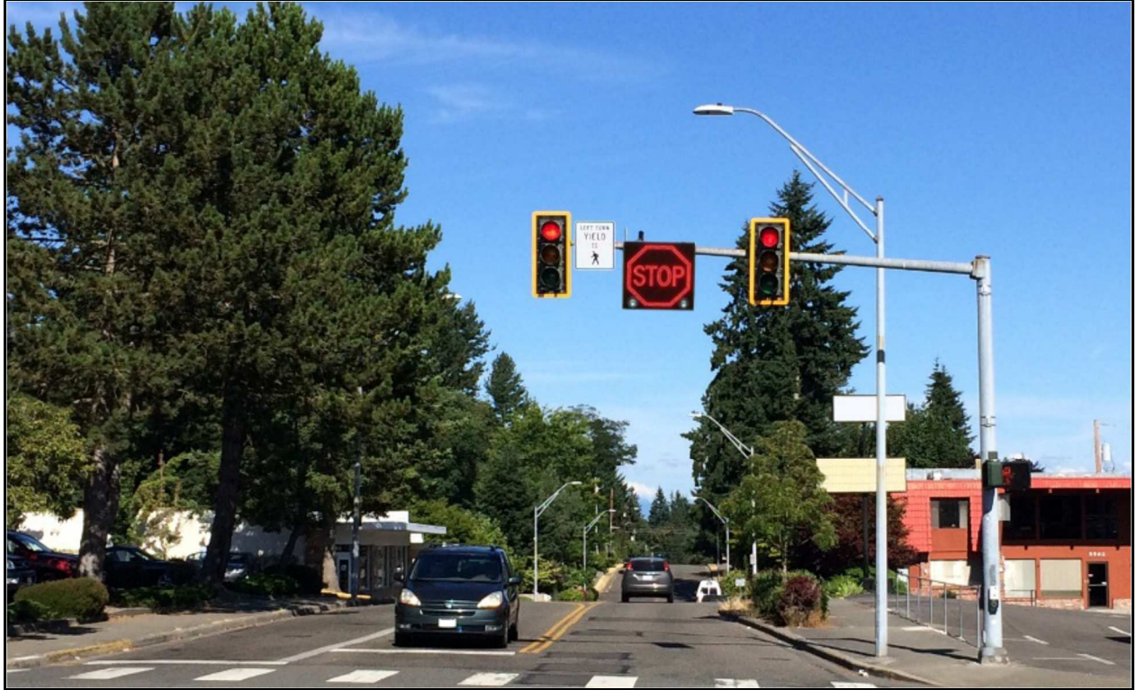
Figure 4-14 Example DII to Support an Intersection Safety Warning and Collision Avoidance to Reduce Red-Light Violation (Richard et al., 2015b)
