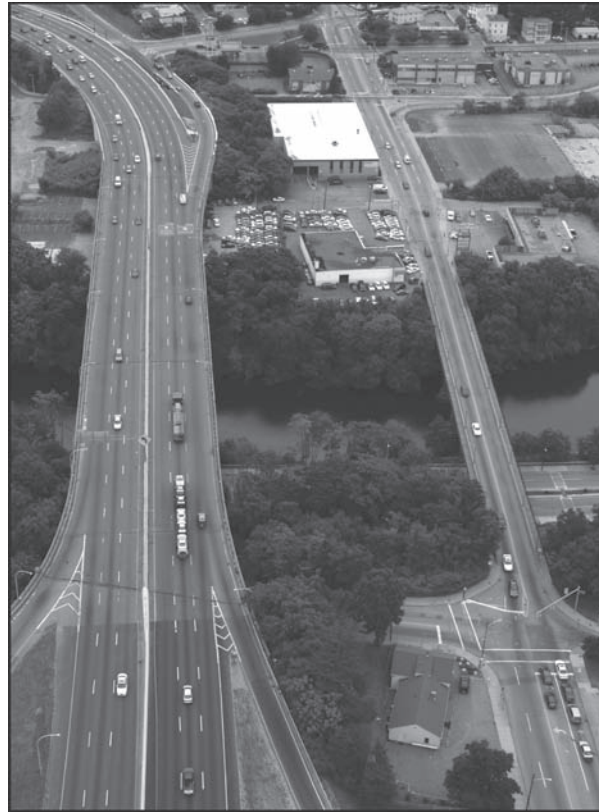
Figure 2 Bridge No. 550 Aerial View
