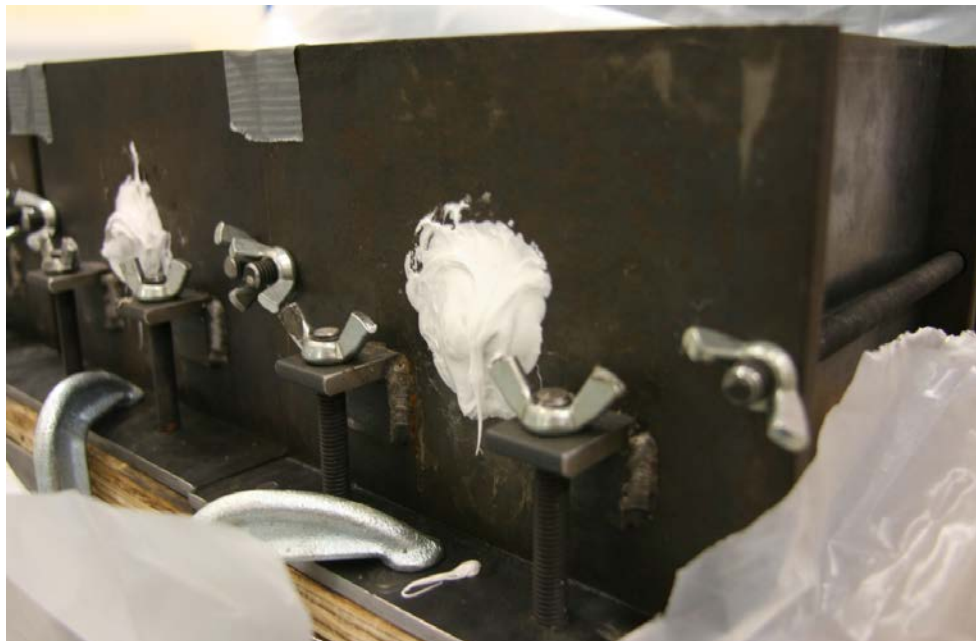
Figure 19. Photograph. Flexible caulk between the formwork and reinforcing bar.
