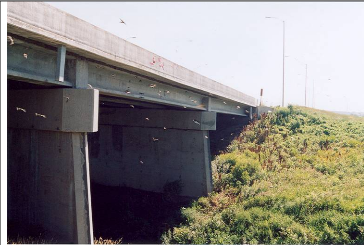
Photo 1: General view of the eastbound bridge facing south.
