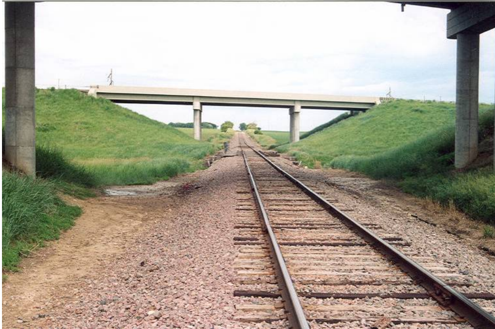
Figure 11. Photo. I-29 Northbound Bridge (Sioux Falls, South Dakota).
