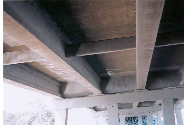
Photo 6: General condition of the girders at Span 2 facing west (southside).
