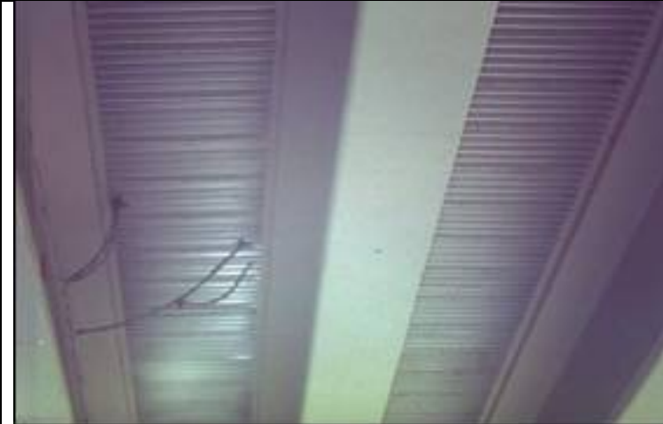
Photo 9. Underside of Deck (Note Stay-in-Place Forms and Connections for Instrumentation.
