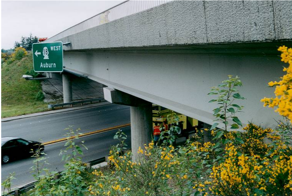
Figure 19. Photo. Eastbound SR18 over SR 516 (King County, Washington).
