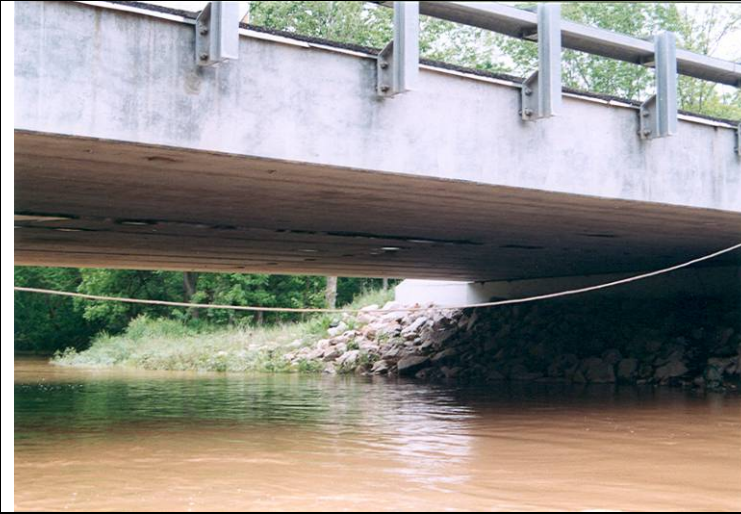
Photo 1: View looking of the east facing bridge from the bank.
