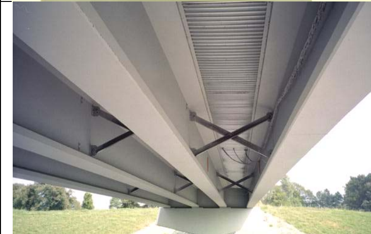
Photo 14: Underside of the deck. Note the connections for instrumentation.
