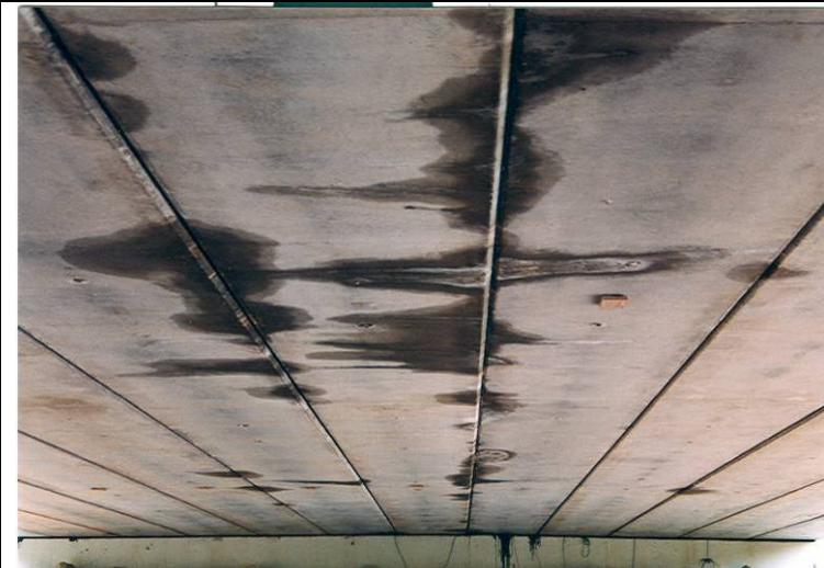
Photo 8: View of the underside of bridge.
