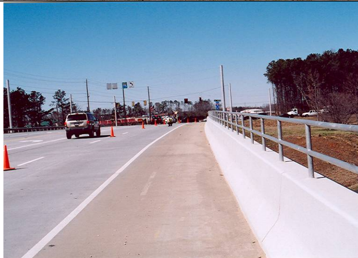
Photo 2: View looking west from the eastern end of the westbound bridge.
