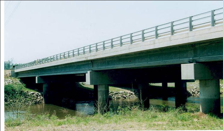
Photo 1: View looking south from the northern end of southbound bridge.
