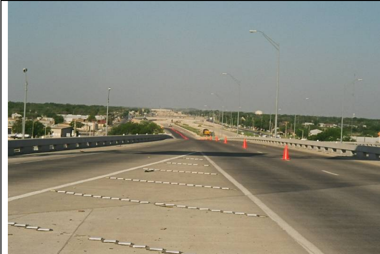
Photo 3: View looking west from the eastern end of the eastbound bridge.
