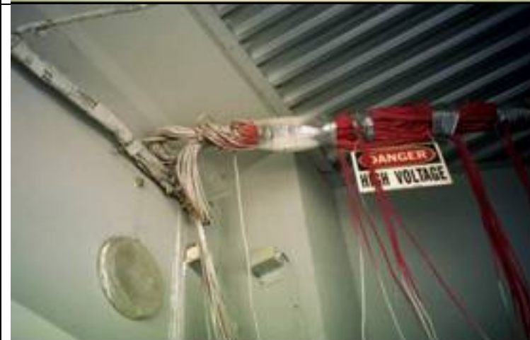
Photo 11. Underside of Deck (Note Instrumentation at Abutment 1, Span 1) Exterior Girder 4 on Left.
