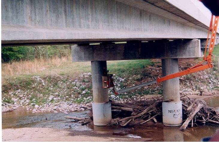
Photo 7: Close up view of bridge deck underside inspection using a snooper.
