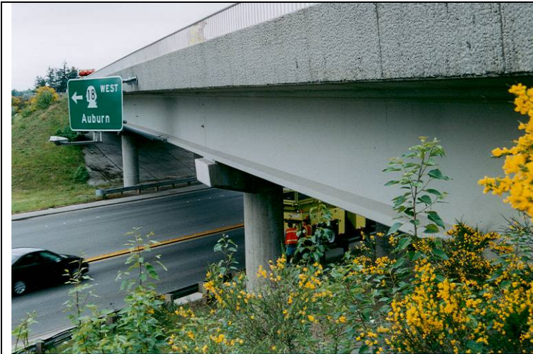
Photo 1: View looking northwest. The eastbound bridge is in foreground.
