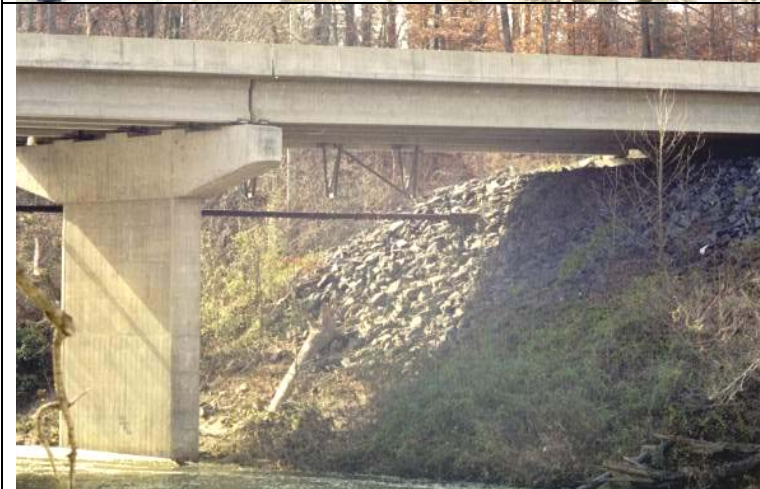
Photo 20: Span A, north elevation, exterior Girder A in foreground.
