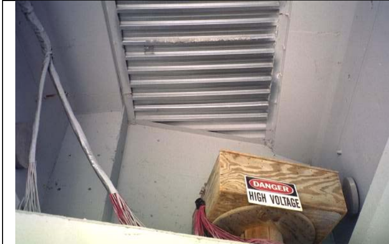
Photo 16: Underside of the deck. Note the instrumentation at abutment 2, girder 1 (exterior) left.
