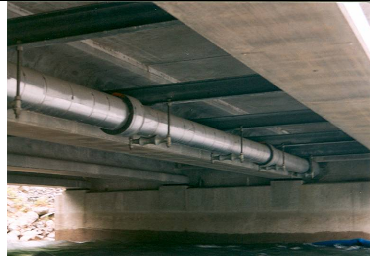
Photo7: Close up view of underside of the bridge.
