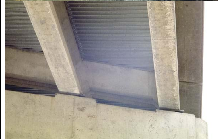
Photo 21: Underside of deck Pier 3, exterior Girder A on right.
