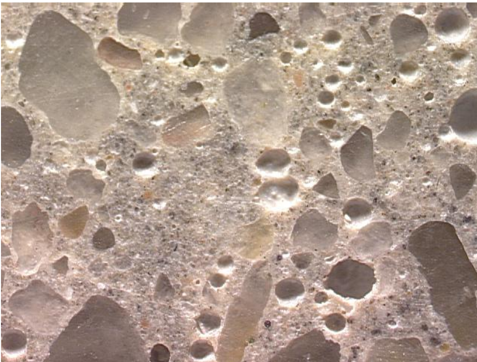
Figure E1-4: Entrained air voids in the concrete. Width of field is 4.0 mm, polished surface image.
