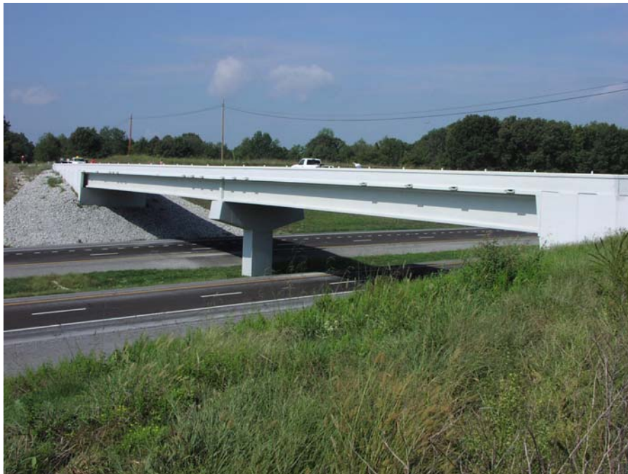
Figure 14. Photo. Hickman Road (Dickson County, Tennessee).
