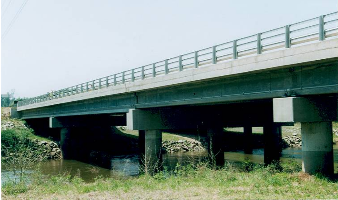
Figure 9. Photo. U.S. 401 Bridge Over the Neuse River (Raleigh, North Carolina).
