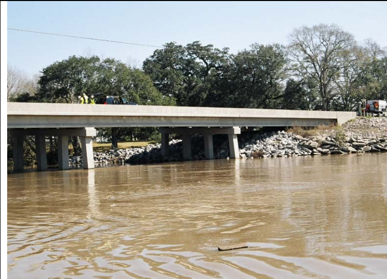
Photo 4: View looking northeast at the western end of the eastbound bridge.
