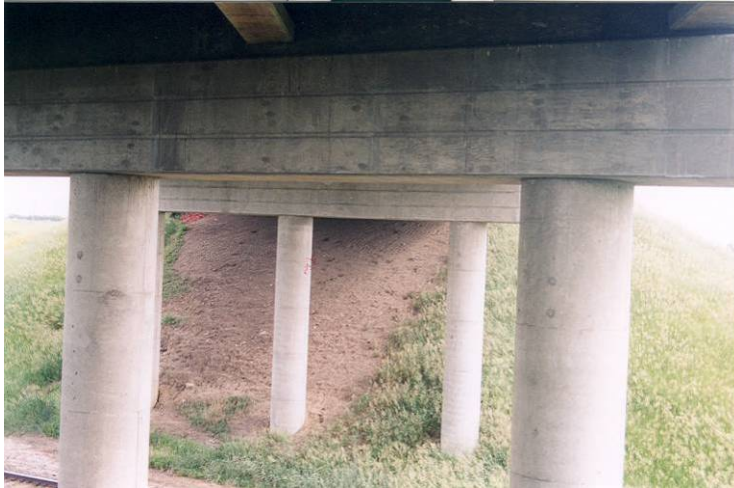
Photo 7: General overview of underside of the bridge.
