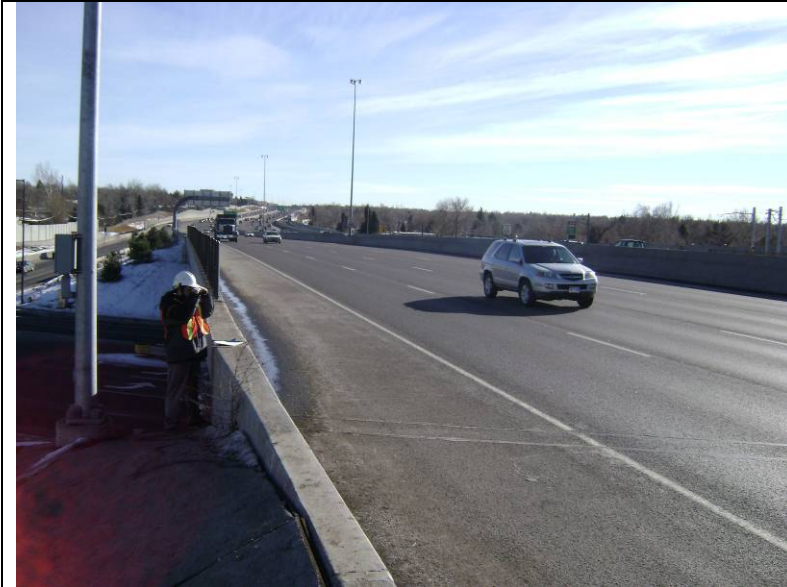
Photo 3: View looking south at the northbound lanes.
