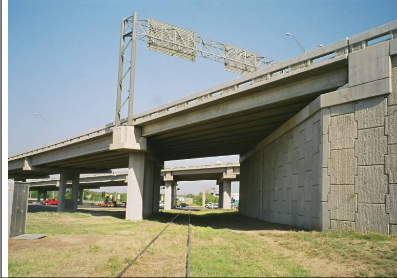
Photo 2: View looking northwest at the eastern end of the eastbound bridge.
