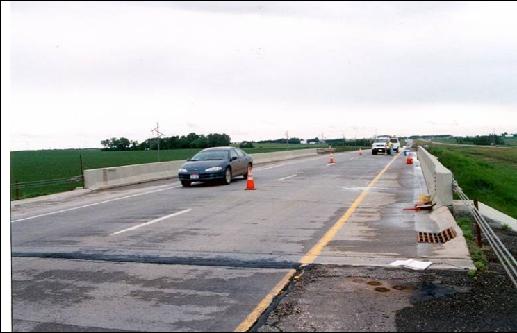
Photo 2: View looking north from the southern end of the Southbound Bridge.
