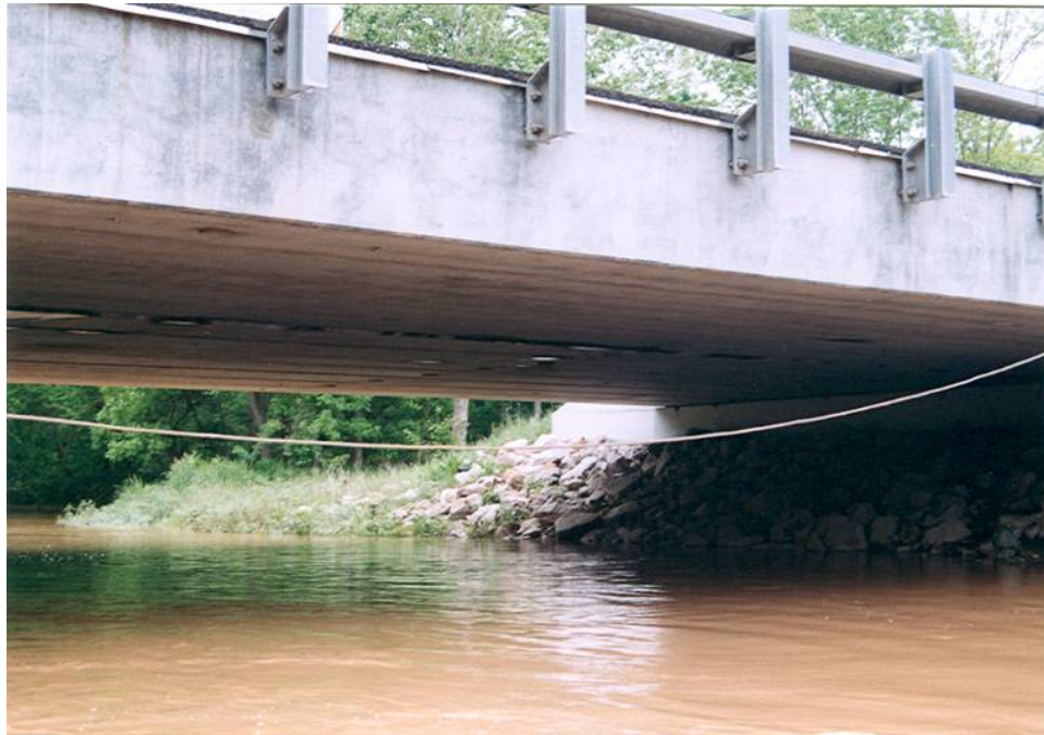
Figure 10. Photo. State Route 22 Bridge at Milepost 6.57, Near Cambridge, Guernsey County, Ohio.
