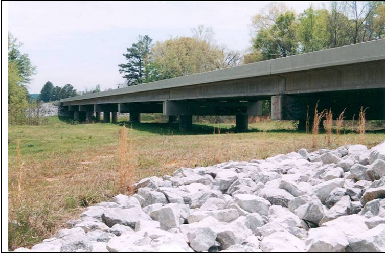
Photo 1: View looking south from the northern end of west facing bridge.
