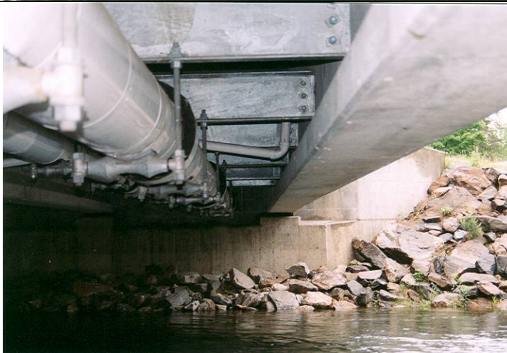
Photo 6: Close up view of bridge deck underside pipe lines.
