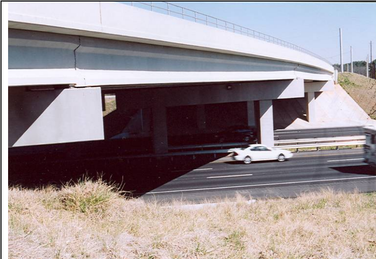
Photo 1: View looking northeast. The eastbound bridge is in foreground.
