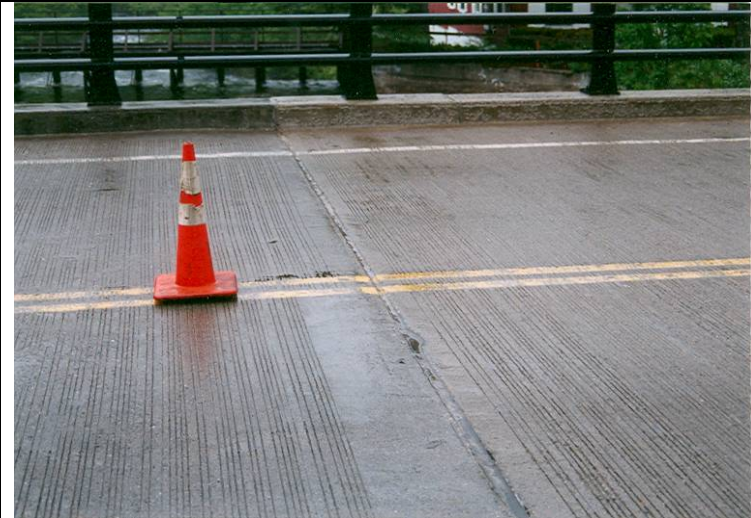
Photo 6: General condition of joint pattern.
