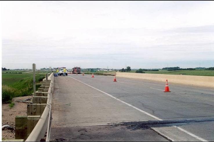
Photo 2: View looking north from the southern end of bridge.
