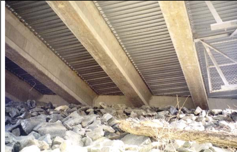
Photo 19: Underside of deck, under Span D.
