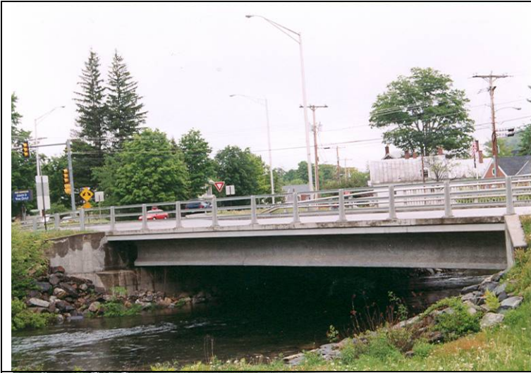
Photo 1: View looking south from the northern end of east facing bridge.
