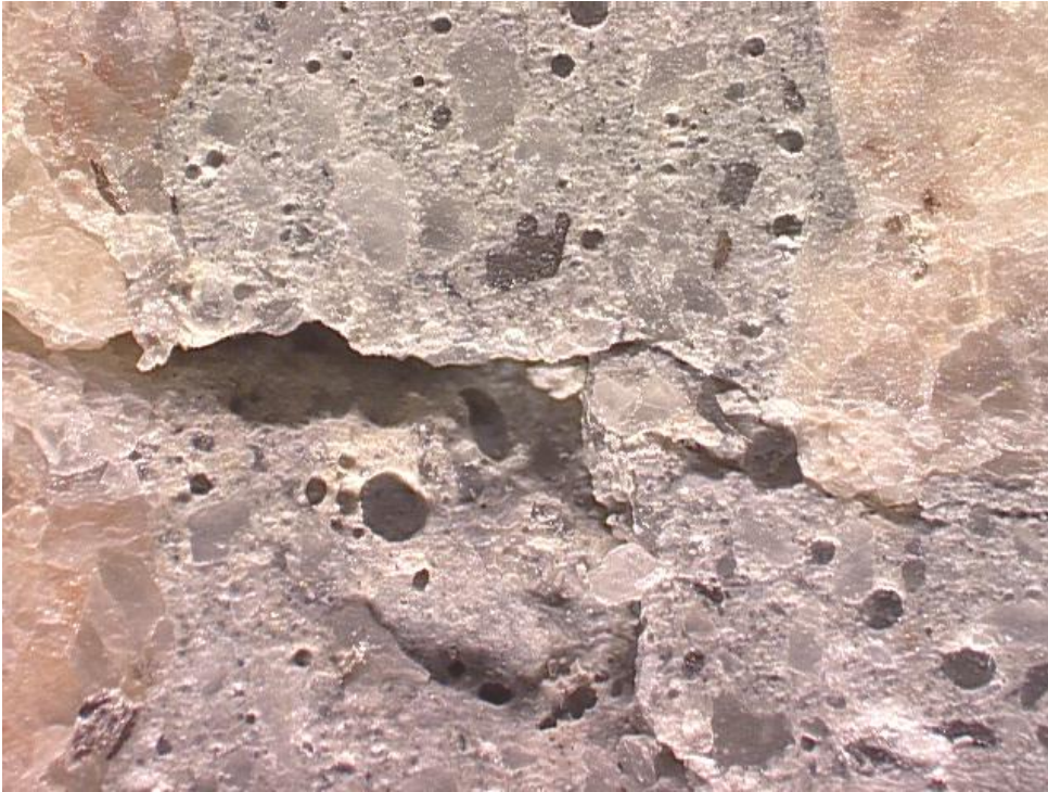
Figure I1-8. Another image of the major crack in core NC-5. Width of field is 6.5 mm.
