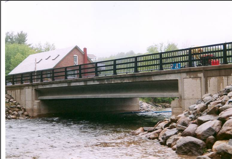
Photo 2: View looking north from the southern end of west facing bridge.
