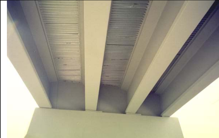
Photo 13: Underside of the deck. Note the stay-in-place forms.
