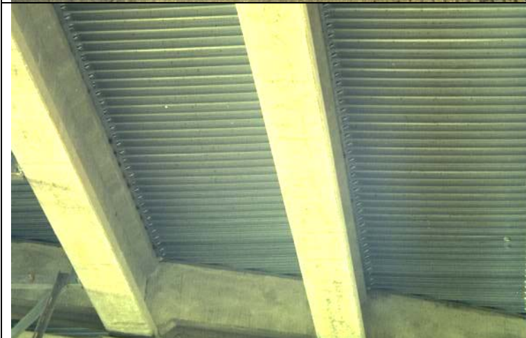
Photo 18: Underside of deck, note stay-in-place forms.
