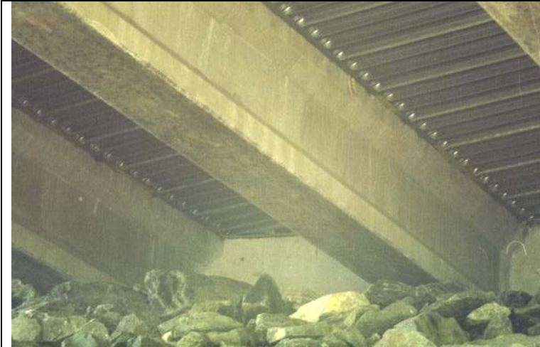
Photo 22: Underside of deck abutment B, exterior Girder A on left.
