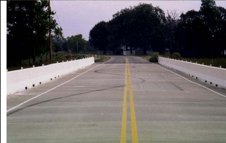
Photo 2: General view of the east approach.
