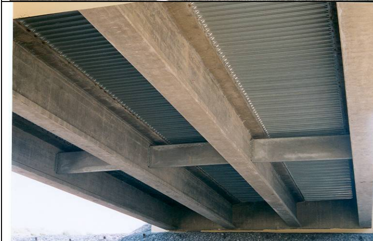
Photo 3: General condition of underside eastbound bridge.
