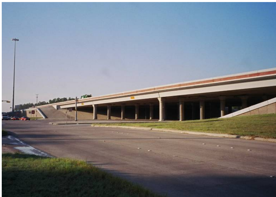
Figure 15. Photo. State Highway 249 (Tomball Parkway) over Louetta Road (Houston, Texas).
