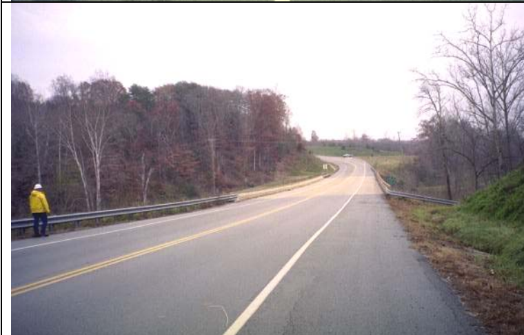
Photo 3: General view, west approach
