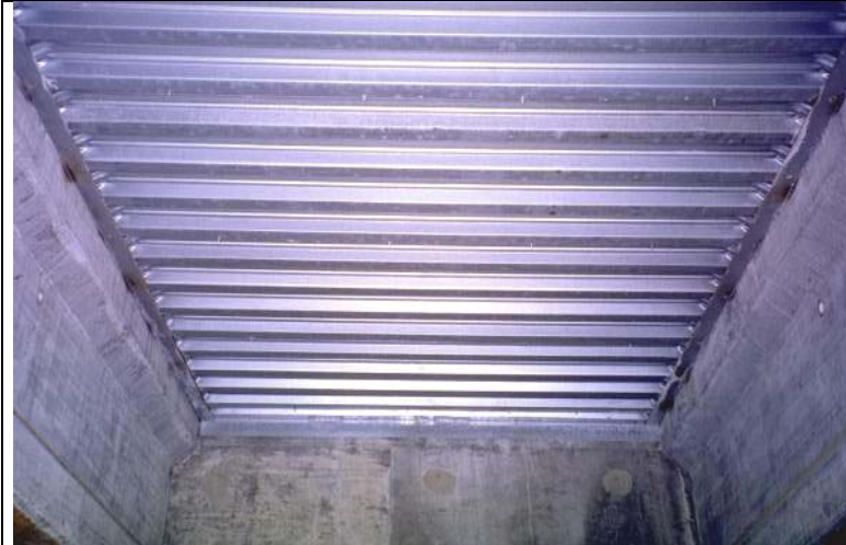
Photo 16: View of the underside of the deck showing the stay-in-place forms.
