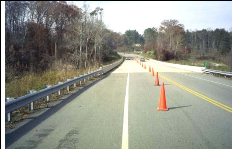
Photo 2: General view, east approach
