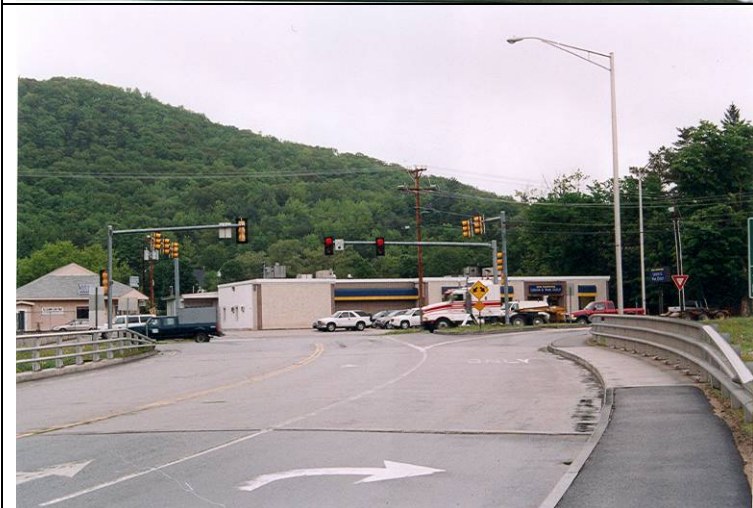
Photo 3: View looking north from the northern end of east facing bridge. Note the right-turn lane on bridge deck.
