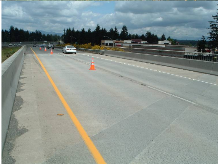
Photo 2: View looking southeast from the western end of the eastbound bridge.
