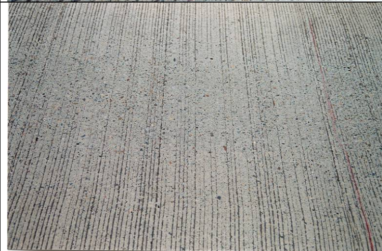
Photo 9: View of the typical polished surface area.
