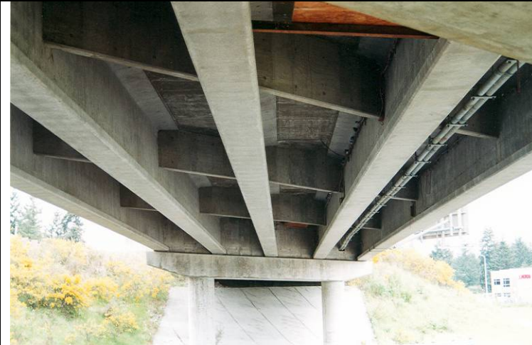
Photo 4: View of the general condition at underside of bridge.
