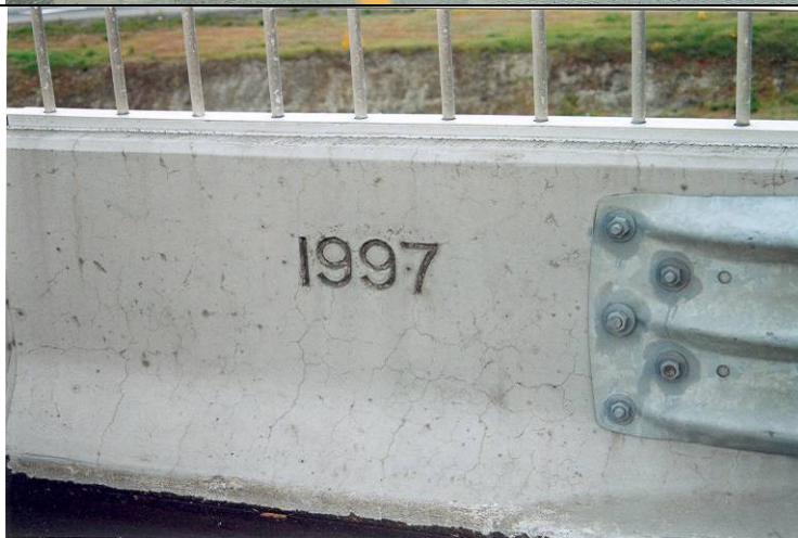
Photo 3: North facing side of the eastbound bridge at the western end.
