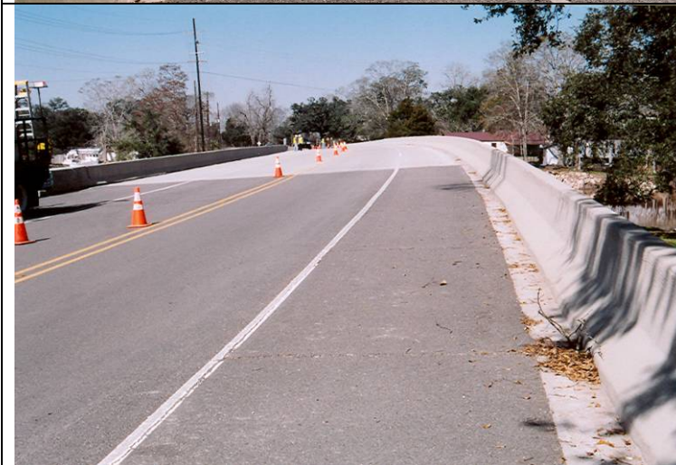
Photo 3: View looking west from the eastern end of the westbound bridge.
