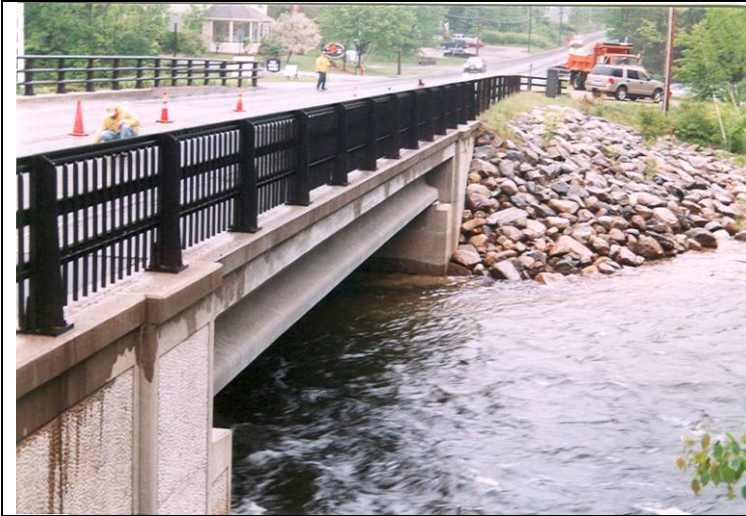
Photo 1: View looking south from the northern end of west facing bridge.
