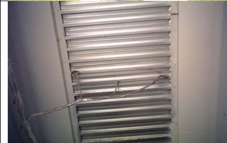
Photo 15: Underside of the deck. Note the connections for instrumentation.
