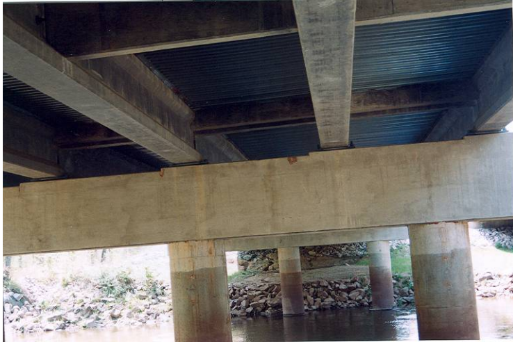
Photo 4: View of the underside of bridge.
