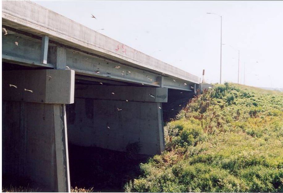
Figure 5. Photo. 120th Street and Giles Road Bridge near Omaha, Nebraska.
