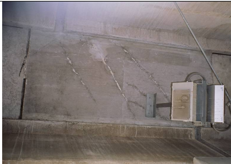
Photo 9: View showing underside of bridge at span end.
