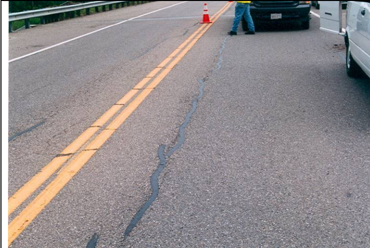
Photo 4: General overall view of the sealed cracks on asphalt wearing surface.
