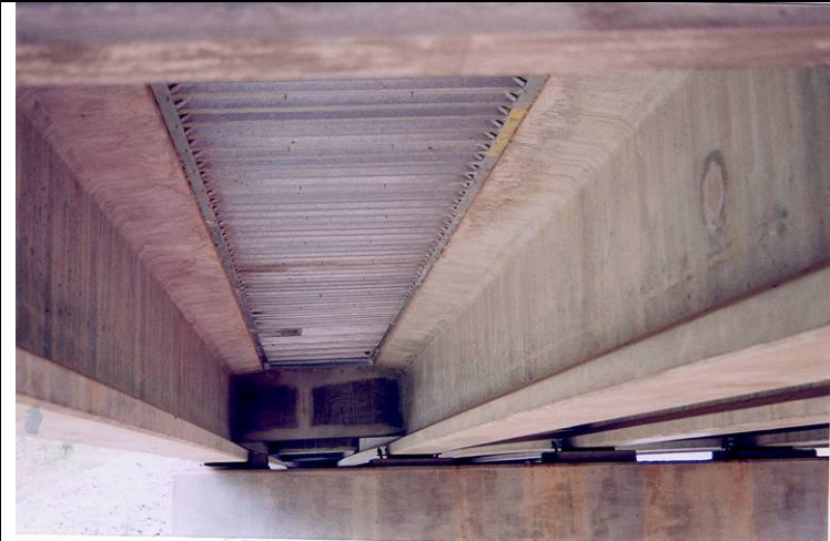
Photo 4: View of the underside of bridge.
