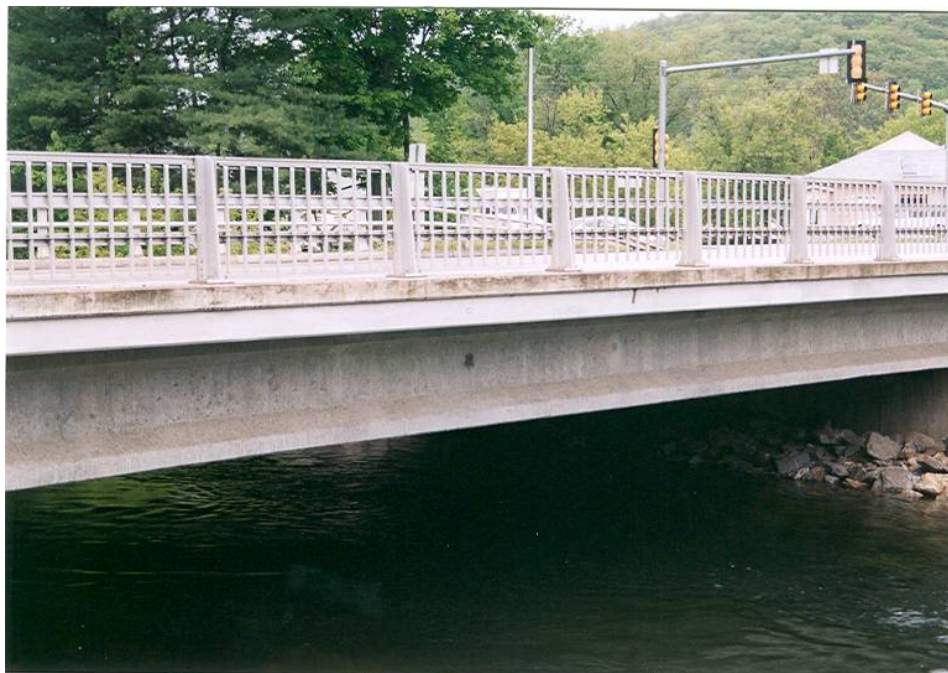
Figure 6. Photo. The Route 104 Bridge (Bristol, New Hampshire).
