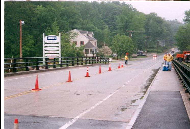
Photo 3: View looking south from the northern end of east facing bridge.
