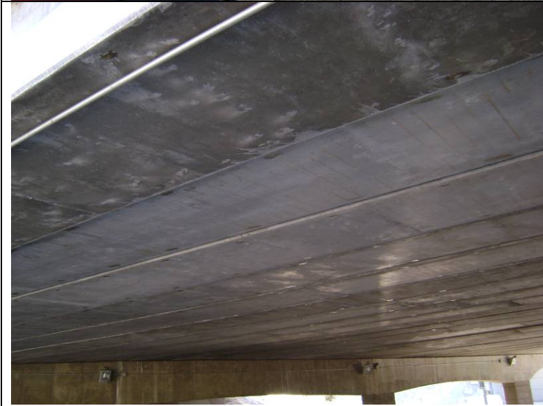
Photo 4: View showing bridge substructure consisting of box girders and columns.
