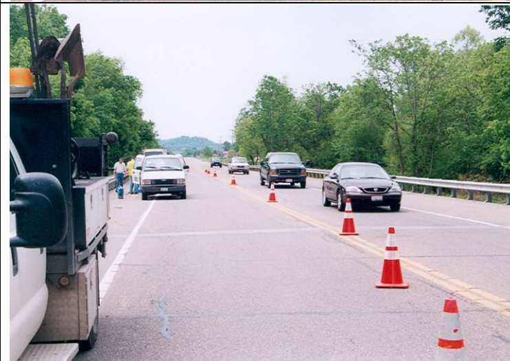
Photo 3: General overall view of the bridge facing east from the southern end bridge decks.
