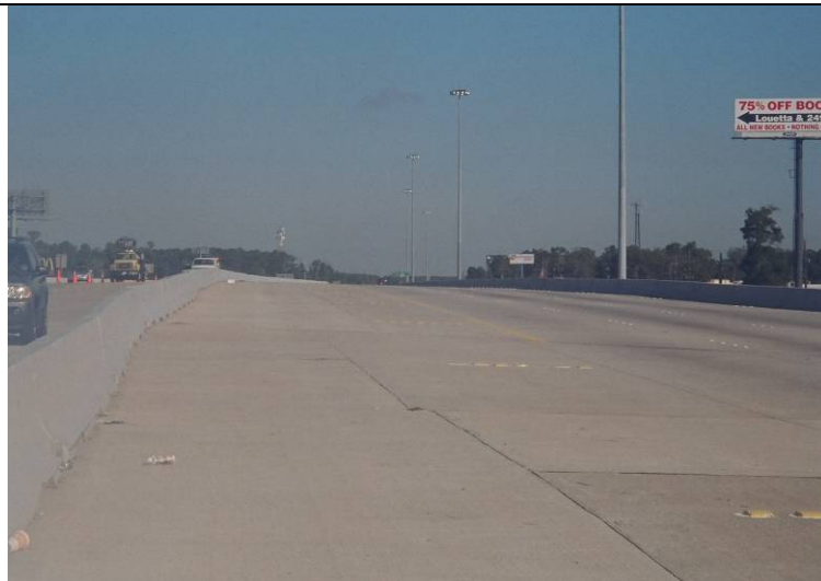
Photo 3: View looking north at the northbound bridge. The approach ramp is in foreground. Span 1 begins at mid-photo.
