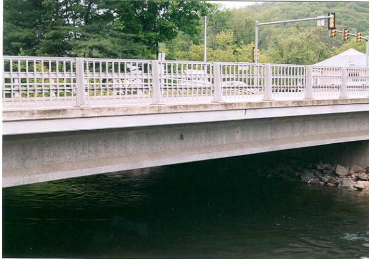
Photo 2: View looking north from the southern end of east facing bridge.
