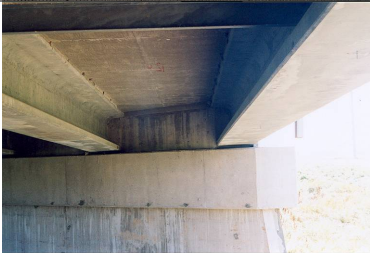
Photo 9: General overview of underside of the bridge.
