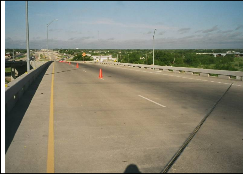
Photo 4: View looking west from the eastern end of the westbound bridge.
