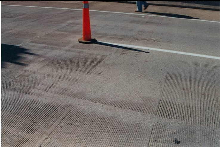
Photo 8: Close up view of polished deck surfaces.
