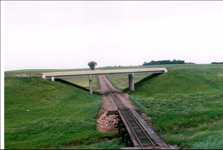
Photo 1: General Overview looking of the I-29 Southbound Bridge from the side.
