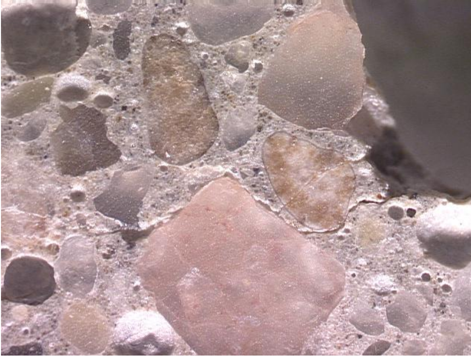
Figure L1-11: Crack at the aggregate-paste interface (crushed pink quartzite). Width of field is 4.0 mm. Polished surface image. Also a crack through an aggregate particle (a rounded natural sand particle with a weathering rim).
