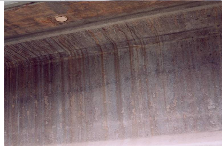
Photo 5: View of the girders from underside of bridge.
