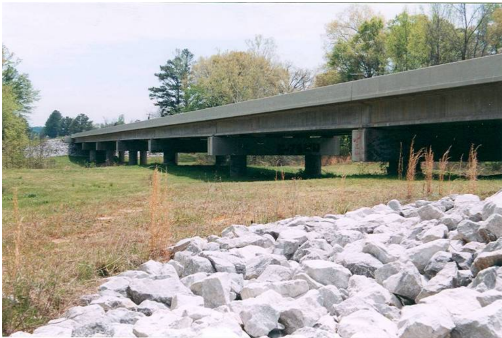
Figure 1. Photo. Uphapee Creek Bridge, Alabama Highway 199 (Macon County, Alabama).
