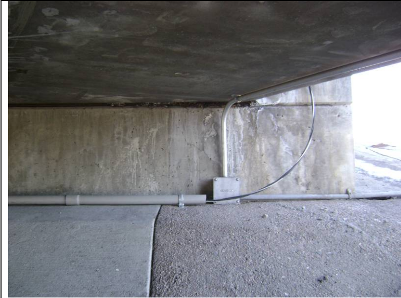
Photo 9: View showing underside of bridge at span end.
