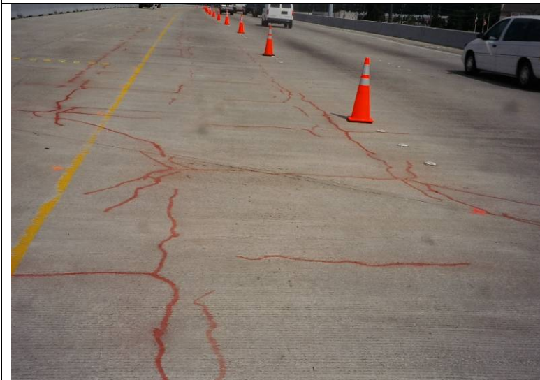
Photo 5: View looking north at the left side of the northbound bridge.
