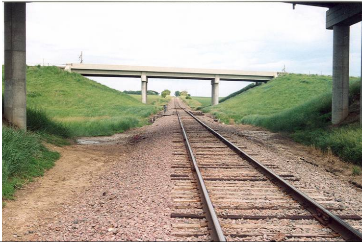
Photo 1: General Overview looking of the I-29 Northbound Bridge from the side.
