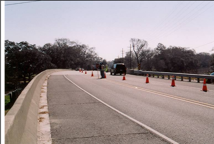
Photo 2: View looking east from the western end of the westbound bridge.
