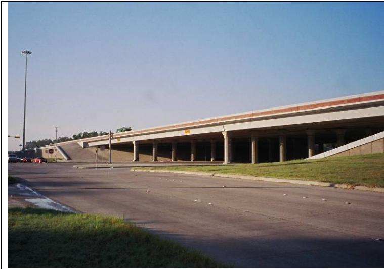
Photo 1: View looking south at the northbound bridge.
