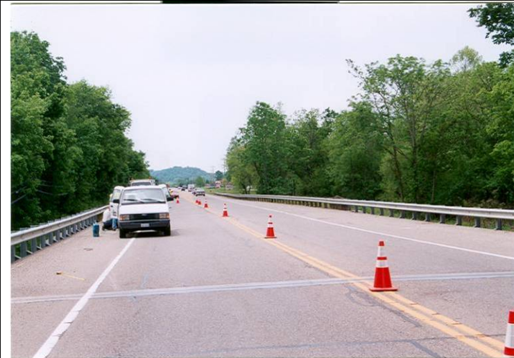
Photo 2: View looking north from the southern end of bridge decks.
