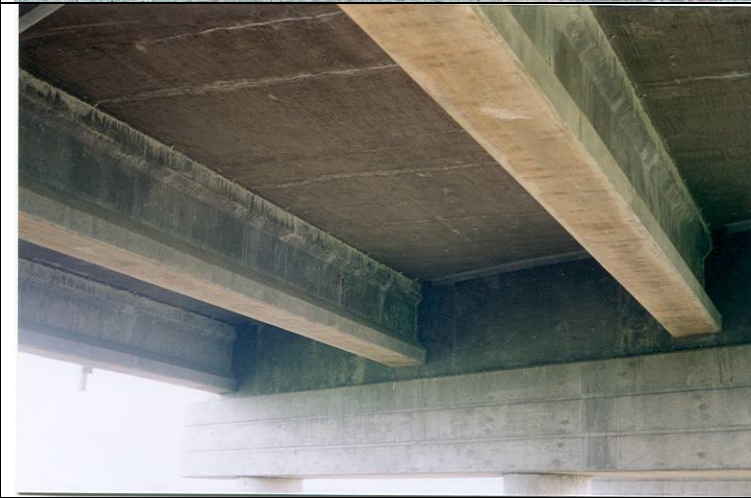
Photo 8: General overview of underside of the bridge.
