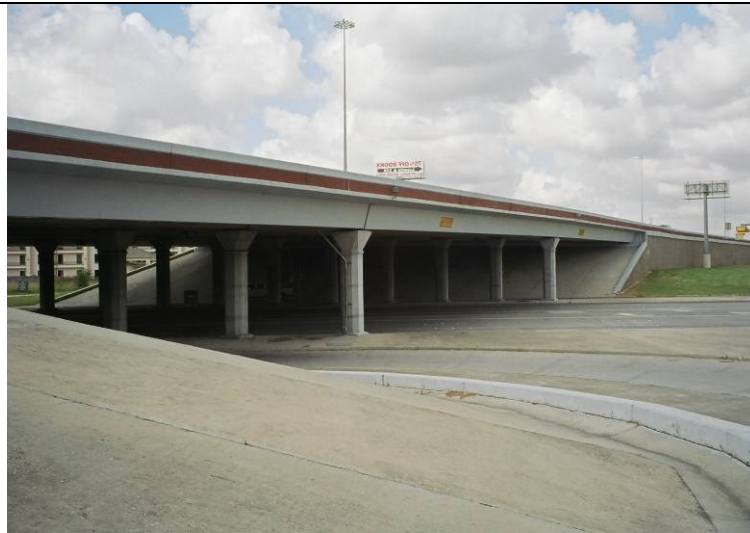
Photo 2: View looking south at the southbound bridge.
