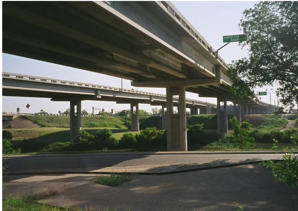
Figure 16. Photo. U.S. Route 67 Bridge (San Angelo, Texas). The eastbound bridge is in foreground, and the westbound bridge is in the background.
