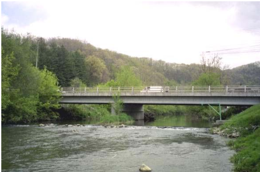
Figure 18. Photo. Virginia Avenue Bridge (Richlands, Virginia).
