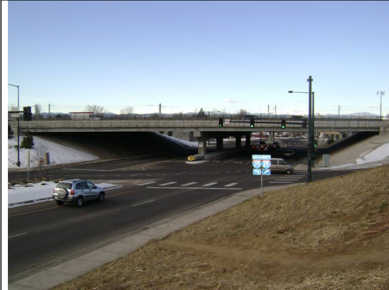
Photo 1: View from the east side of the bridge.
