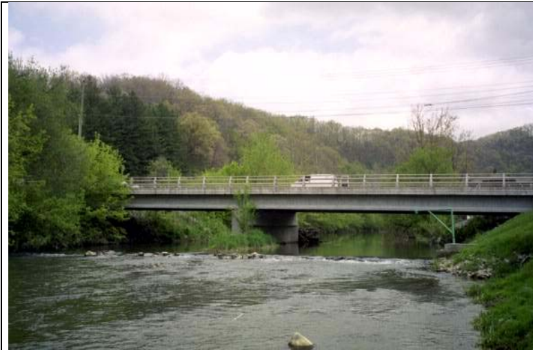
Photo 1: General view of the west elevation. Looking upstream.
