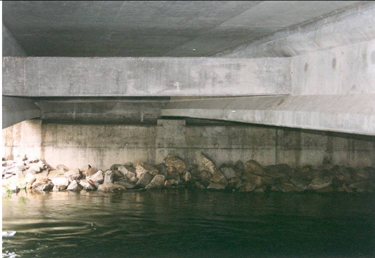
Photo 5: Close up view of bridge deck underside inspection using a boat.
