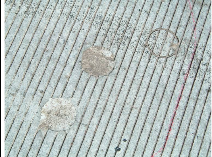
Photo 11: View of the existing drilled cores on Span 3 westbound bridge.
