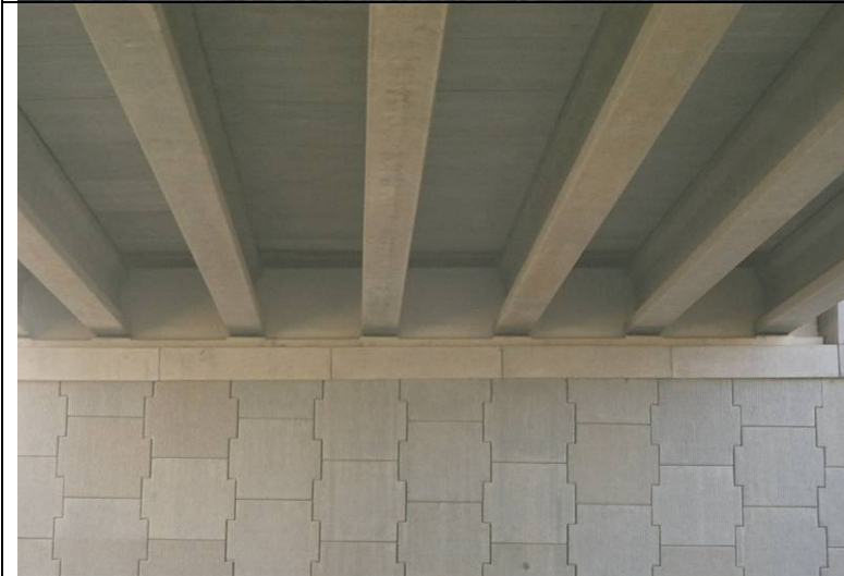
Photo 9: Typical condition of the underside of the deck.
