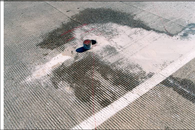
Photo 11: Taking core from a location over a transverse crack.
