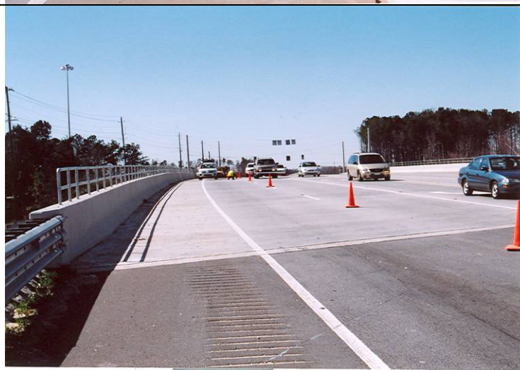
Photo 3: View looking east from the western end of the eastbound bridge.
