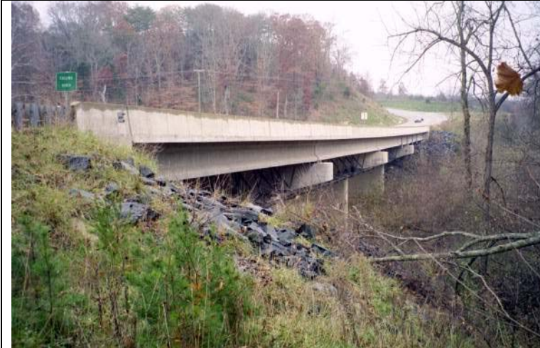
Photo 1: General view, south elevation.
