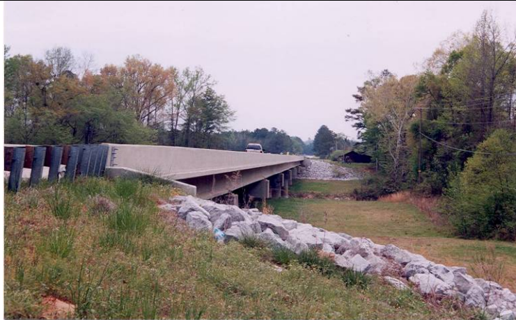
Photo 3: View looking south from the northern end of east facing bridge.
