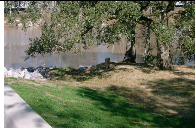
Photo 12: Close up view of the settlement at the eastern end of westbound bridge Span 5.
