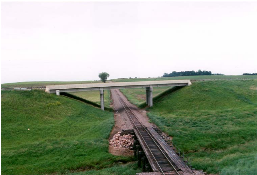
Figure 12. Photo. I-29 Southbound Bridge (Sioux Falls, South Dakota).
