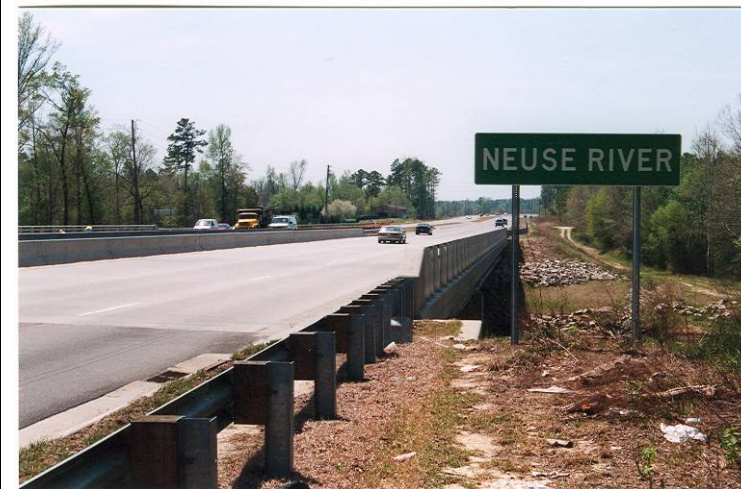
Photo 2: View looking north from the southern end of northbound bridge.
