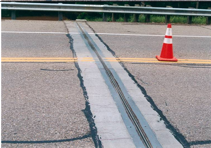
Photo 5: Transverse expansion joint at the end of the bridge.
