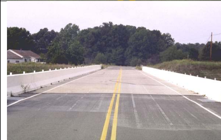
Photo 3: General view of the west approach.
