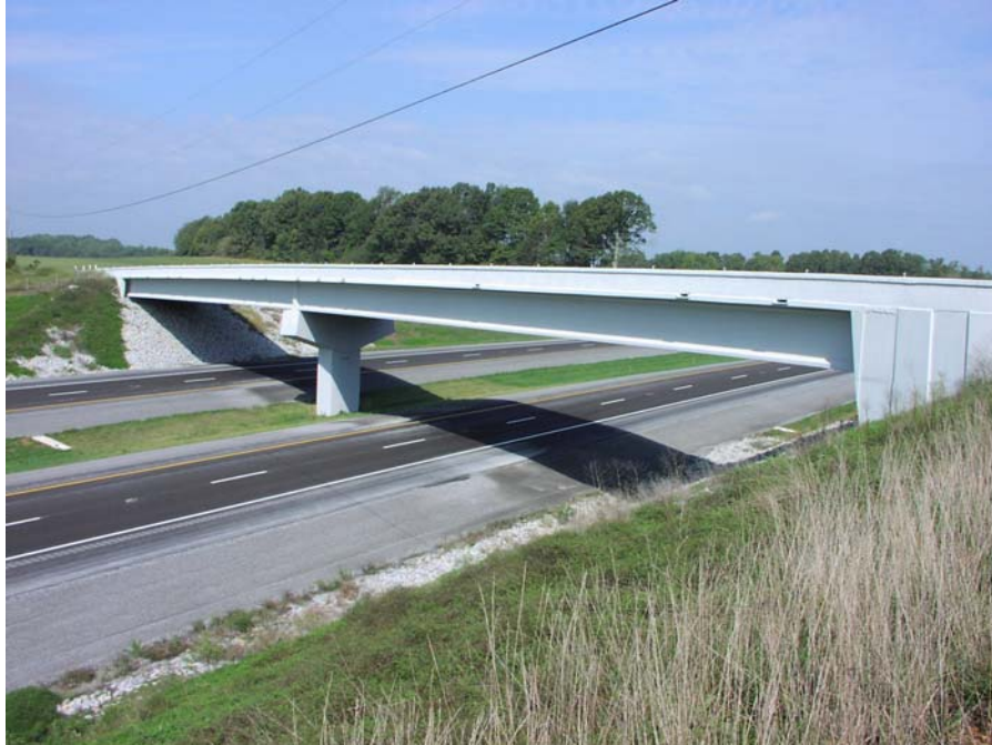
Figure 13. Photo. Porter Road (Dickson County, Tennessee).
