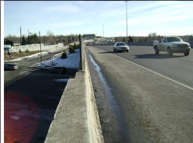
Photo 6: View looking at the east side of the northbound lanes.
