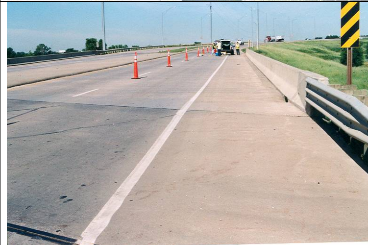
Photo 2: General view of the westbound bridge at eastern end.
