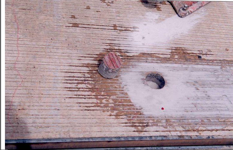
Photo 13: View of the drilled cores on bridge deck.
