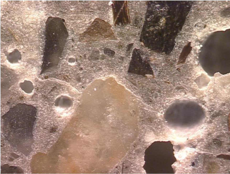
Figure F1-9: Cracks in the aggregate peripheral zone. Width of field is 2.0 mm. Polished surface image.
