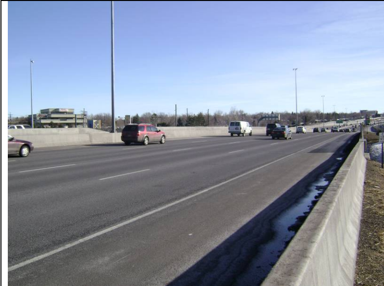
Photo 5: View looking south at the southbound lanes.
