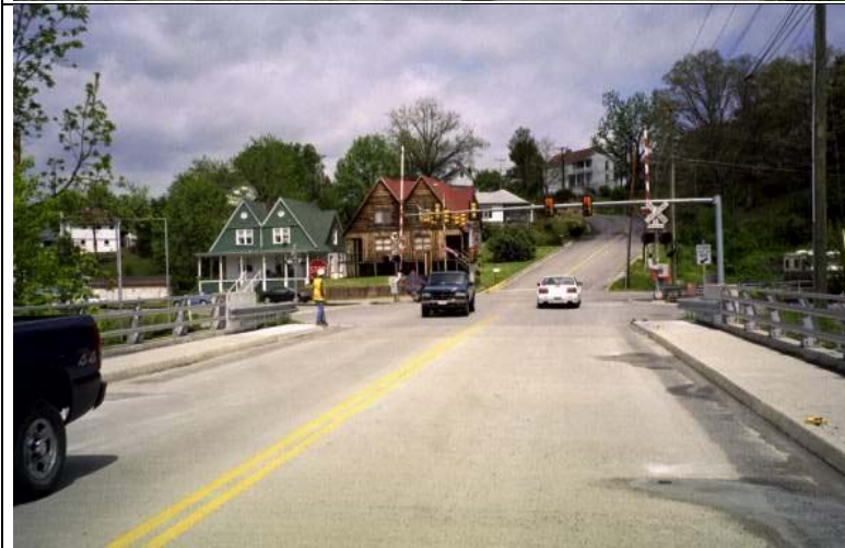
Photo 2: View looking at the north approach.
