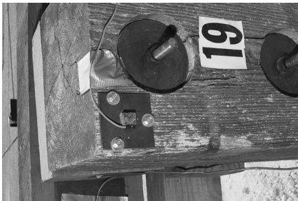
d) Accelerometer on Post 19.
