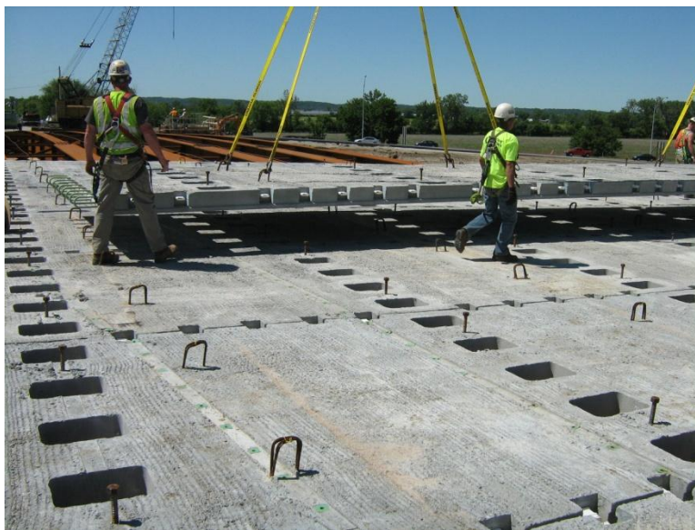
Figure 1 Bridge deck being constructed with full depth precast concrete deck panels (courtesy Iowa DOT).
