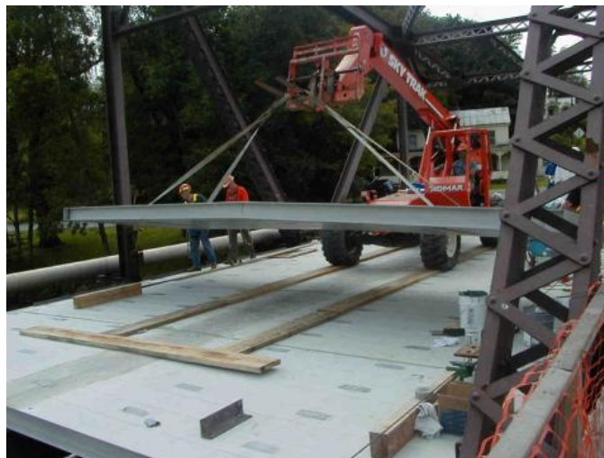
Figure 17 Photo showing the installation of an FRP deck panel for deck replacement project in New York State (courtesy NYSDOT and FHWA)
