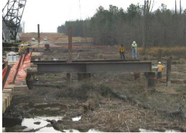
Figure 27 Steel pipe piles, steel pier caps, and steel framing, with a timber mat deck, form the structural system for this temporary work bridge.
