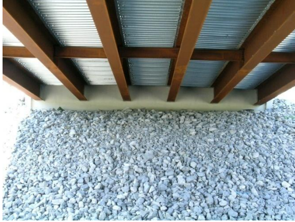
Figure 14 Photograph of a completed integral abutment.
