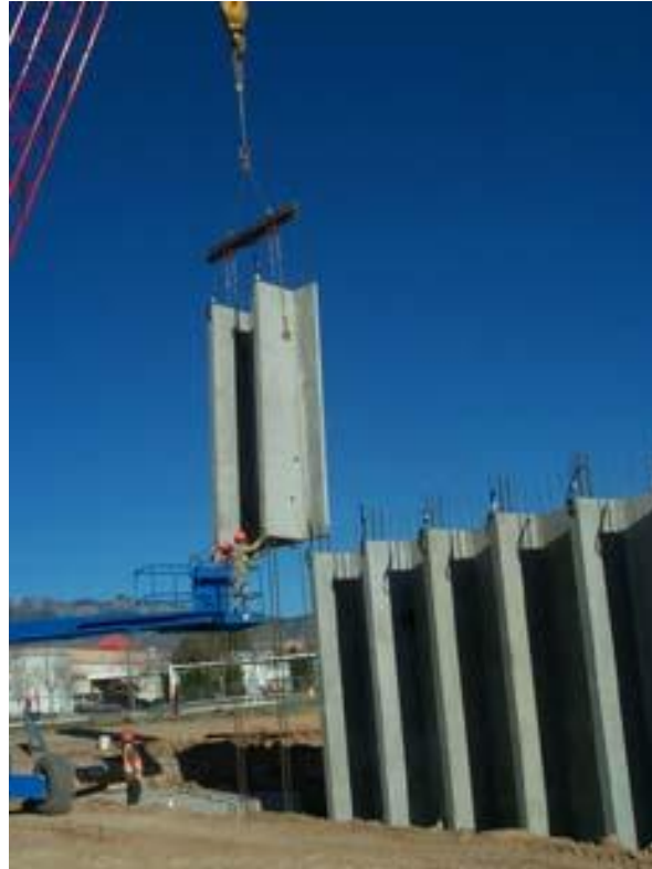
Figure 33 Opportunities abound for innovation in substructure design. This unique full height abutment which uses precast double-tees for the stem wall is one example of a creative solution that addressed the specific criteria of a given project.
