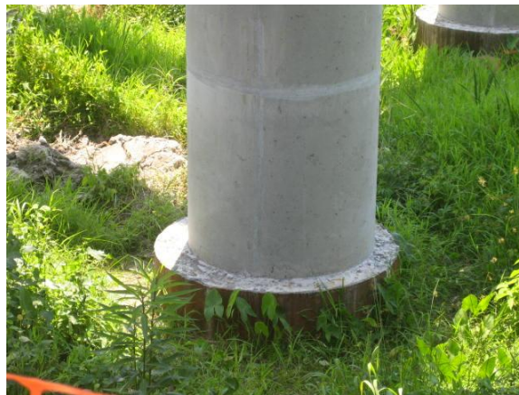
Figure 8 Single round column with an oversized, steel cased, drilled shaft.
