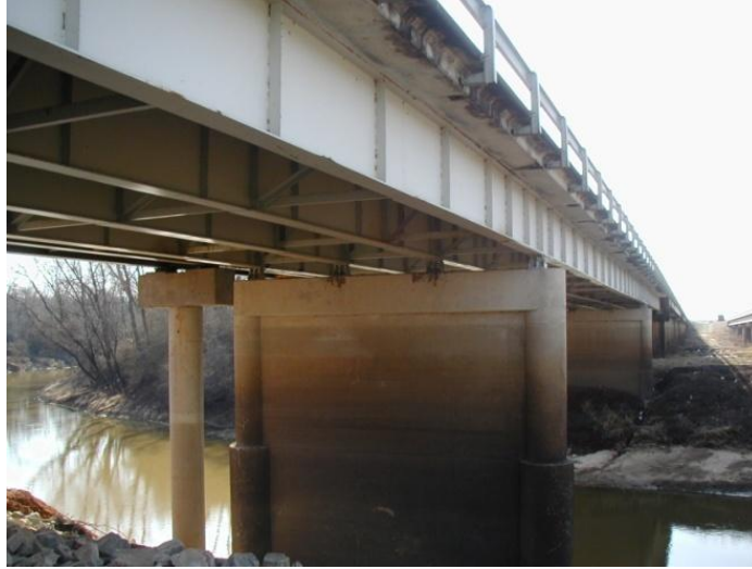
Figure 31 Example of the wide range of variations in pier types. This project featured the widening of an existing bridge which used multi-column piers with web walls. The widened section used single column hammerhead piers.
