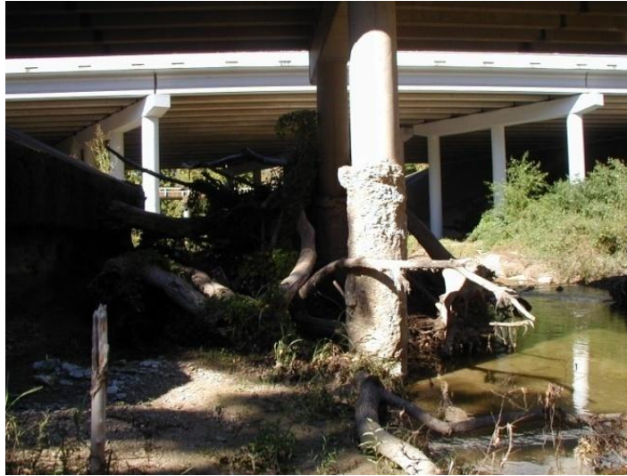
Figure 6 The effects of scour can be severe. Here a drilled shaft in a multicolumn bent has experienced over 6 feet of permanent (erosion) scour; during a flood event with higher velocity flow, there will be even more temporary (local pier) scour at this pier.
