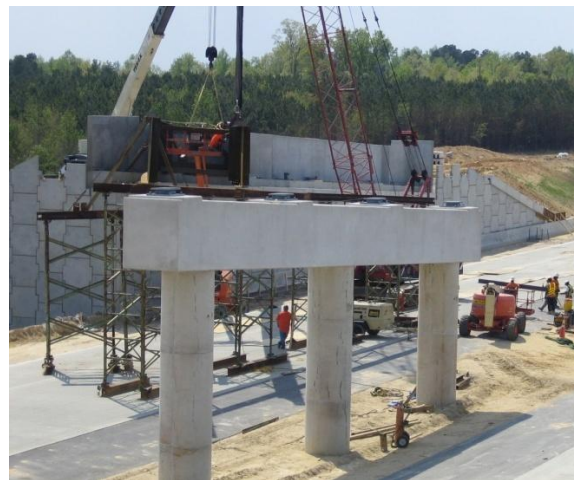
Figure 18 Typical multi-column pier with round columns and a stepped pier cap.
