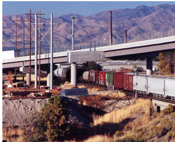
Figure 24 Example of a straddle bent carrying a highway bridge over a railroad line. In this case, the pier cap is also fully integral with the curved steel girder superstructure.
