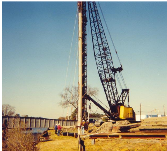
Figure 4 Driving of a precast concrete pile.
