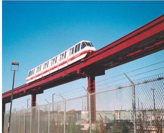
Figure 28 Steel single column hammerhead piers for a dual box girder automated people mover bridge.
