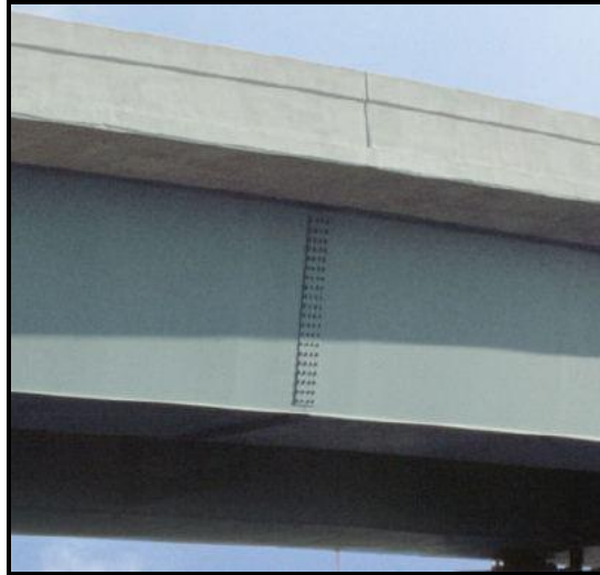
Figure 21 Photograph of a Box Girder Field Splice
