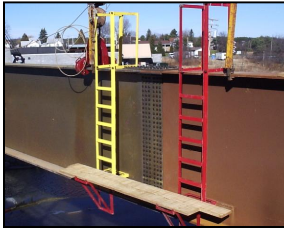
Figure 10 Photograph of a Girder Web Splice
