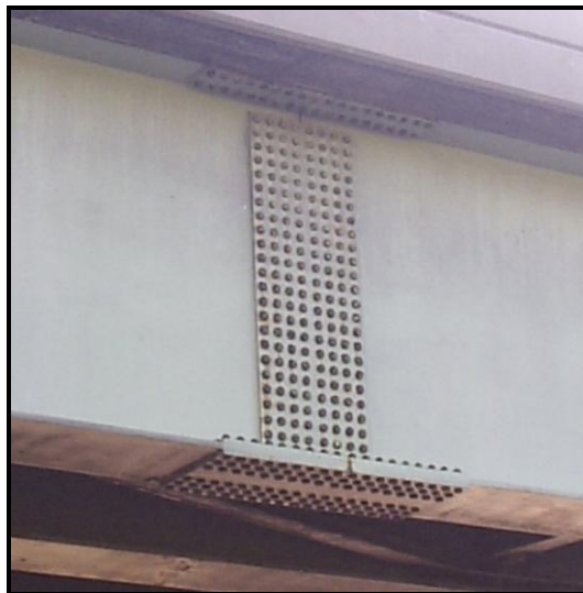
Figure 1 Photograph of a Steel Plate I-Girder Field Splice
