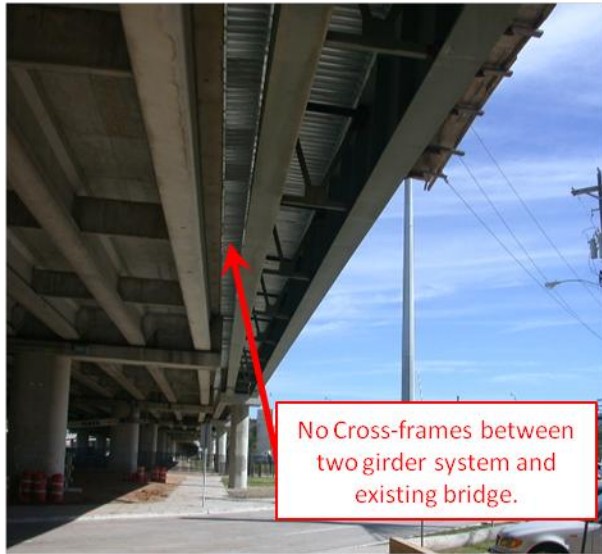
a) Twin Girder Widening
