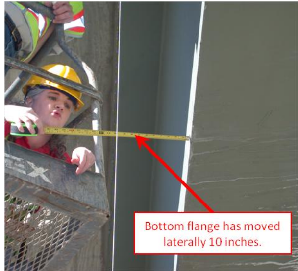
b) System Buckling
