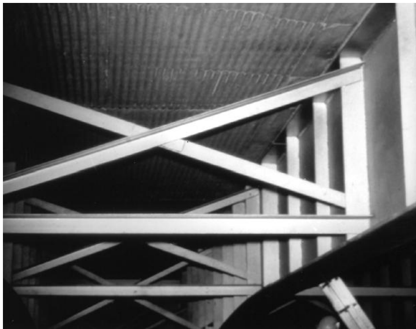
Figure 14 X-Bracing and Girders
