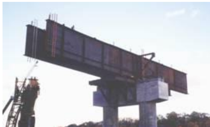
Figure 8 Photograph showing the use of pier brackets in an I-girder bridge
