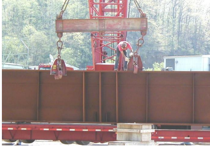
Figure 9 Photograph showing the use of a spreader beam for I-girder erection
