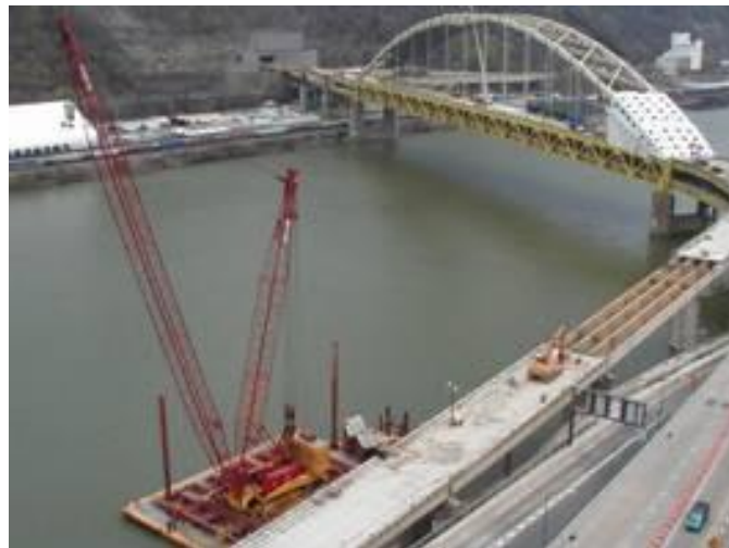
Figure 4 Photograph of a lattice ringer crane
