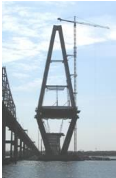
Figure 5 Photograph of a tower crane
