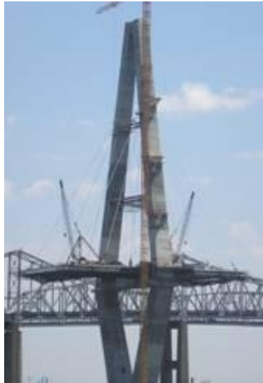
Figure 17 Photograph showing cantilever cable stayed bridge erection using deck mounted derricks
