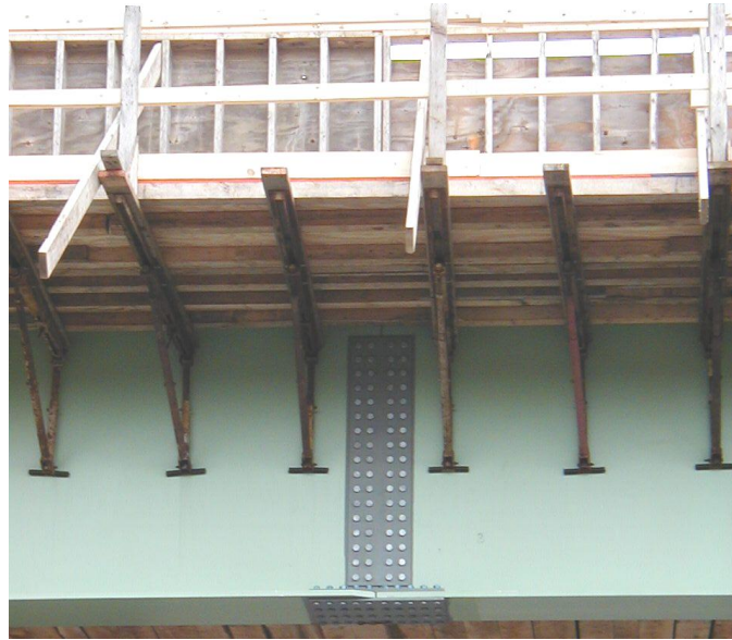
Figure 20 Photograph of a typical overhang bracket
