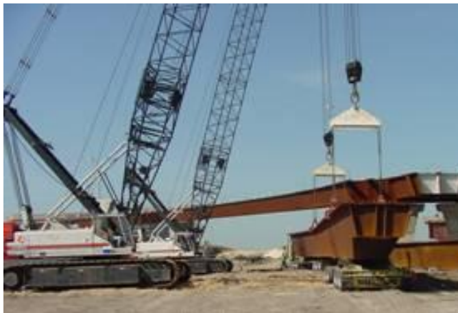
Figure 10 Photograph showing box girder erection using two crawler cranes
