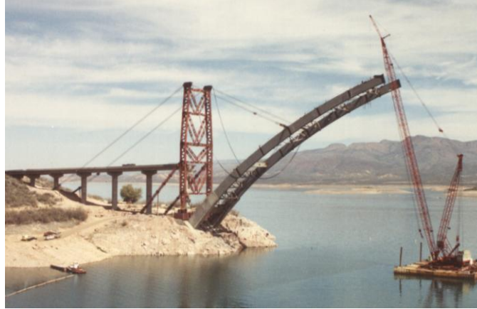
Figure 15 Photograph of an arch erection using stay towers and cables
