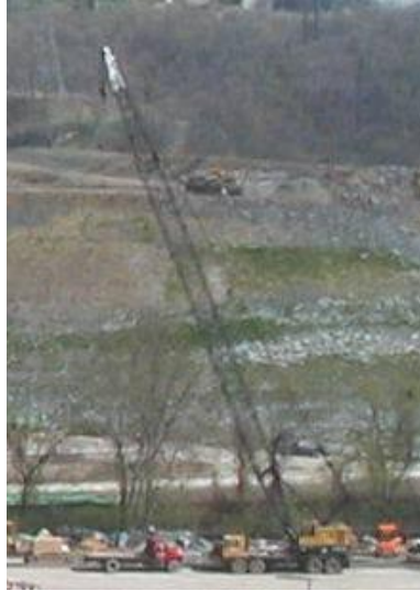
Figure 2 Photograph of a mobile lattice boom crane
