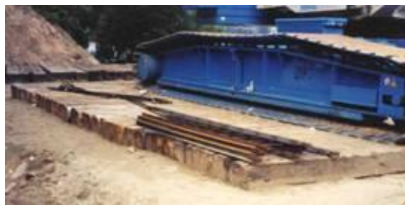
Figure 6 Photograph of a timber crane mat
