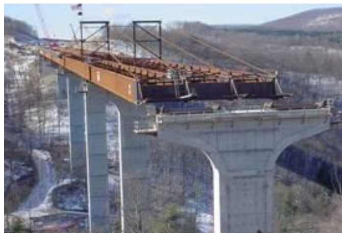
Figure 12 Photograph showing an I-girder launch with cable tie-backs
