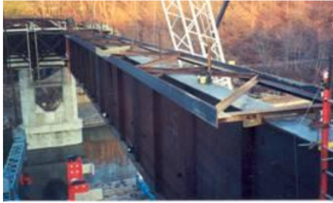
Figure 24 Photograph showing a temporary top flange stiffening truss
