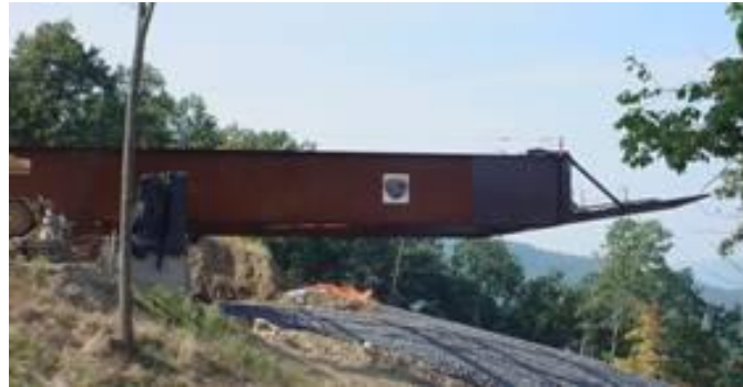
Figure 11 Photograph showing an I-girder bridge launching
