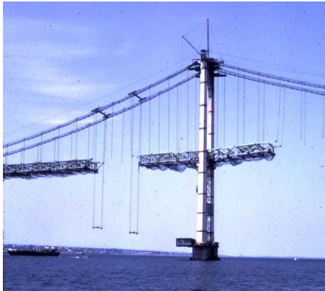
Figure 18 Photograph of a suspension bridge erection using cable travelers
