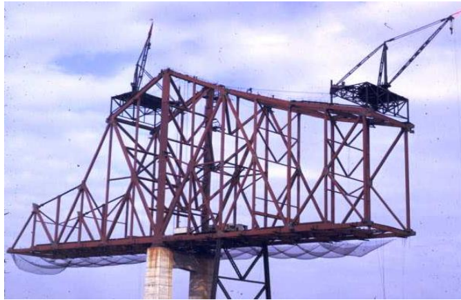
Figure 14 Photograph showing cantilever erection of a continuous truss using derricks
