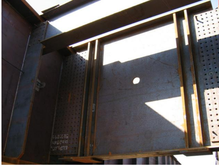
Figure 4 Photograph of a full-depth plate diaphragm at the end of a span
