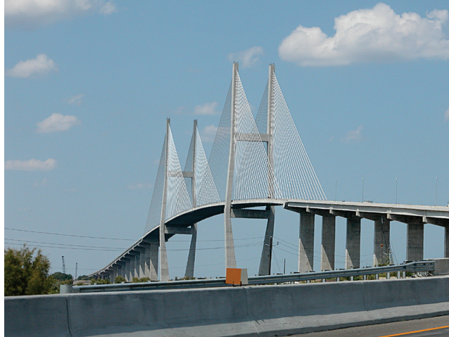
Figure 11 Photo of the Sydney Lanier Bridge, Brunswick, Georgia
