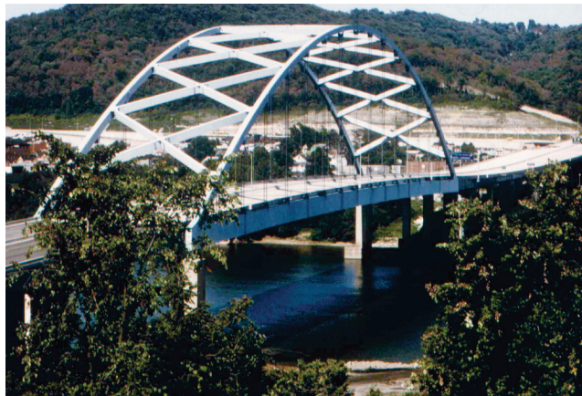
Figure 9 Photo of the I-470 Bridge over Ohio River, Wheeling, West Virginia
