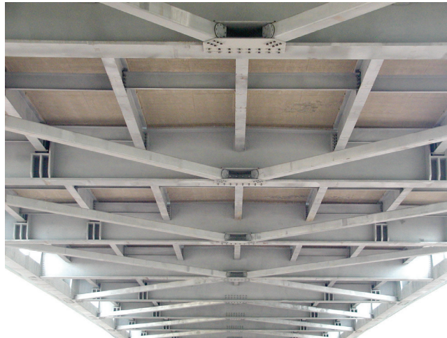
Figure 7 Photo of a typical framed floor system
