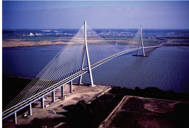
Figure 13 Photo of the Normandy Bridge over Seine River near Le Havre, France
