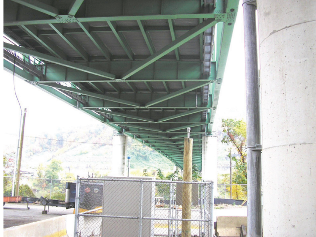
Figure 6 Photo showing a typical stacked floor system
