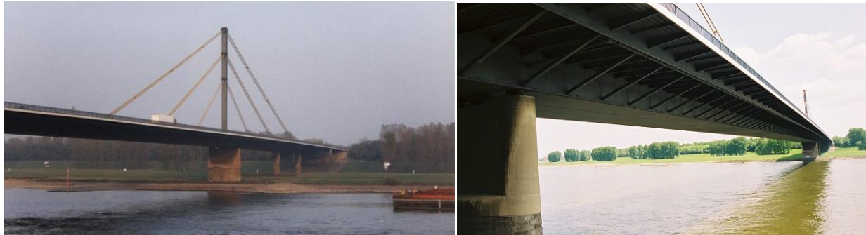
(a) Overall view
