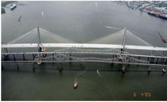
(a) Aerial view
