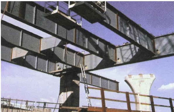
Figure 16 Straddle bents with integral steel pier caps (Abu-Hawash et al. 2005) (courtesy of Iowa DOT, HDR Engineering, and NSBA).
