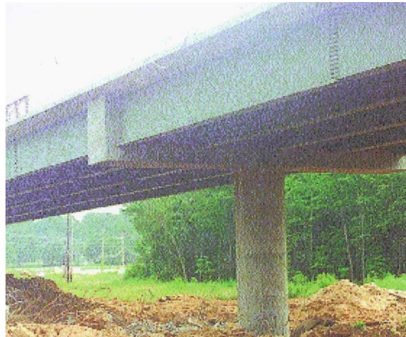
Figure 15 Typical post-tensioned concrete integral bent cap with a single column pier (Wasserman 1997) (courtesy of Tennessee DOT and NSBA).
