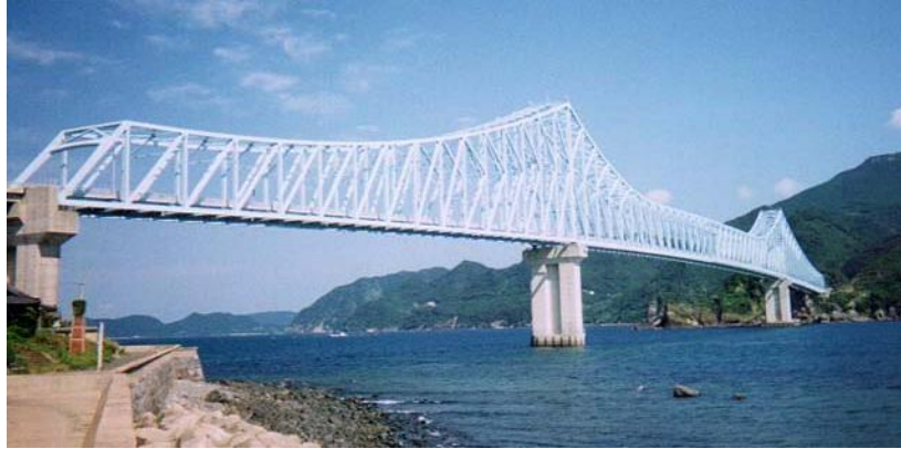
Figure 26 Ikitsuki Ohashi Bridge, Nagasaki, Japan, longest-span continuous truss bridge, 1300 ft main span ( www.sight-seeing.japan.com )
