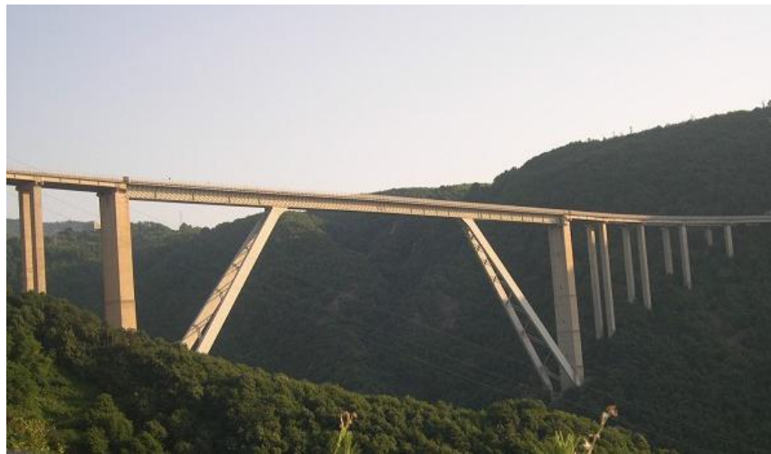
Figure 25 Sfalassà Bridge in Calabria, Italy, longest box-girder span, 1230 ft (courtesy of www.structurae.de )
