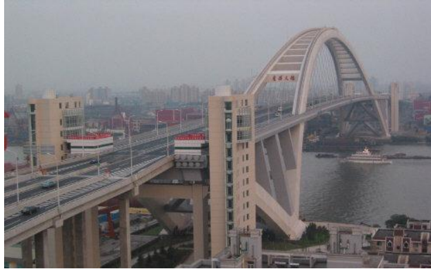
Figure 30 LuPu Bridge in Shanghai, China, longest span steel arch, 1800 ft (courtesy of www.structurae.de ).
