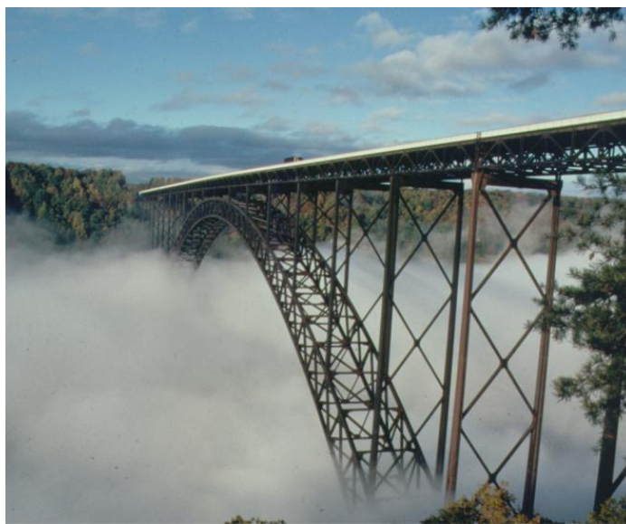
Figure 32 New River Gorge Bridge in West Virginia, longest span steel arch in the United States, 1700 ft (courtesy of HDR Engineering, Inc.)
