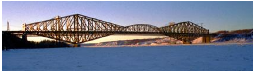
Figure 27 Quebec Bridge in Quebec, Canada, longest span cantilever truss bridge, 1800 ft main span (courtesy of www.structurae.de ).
