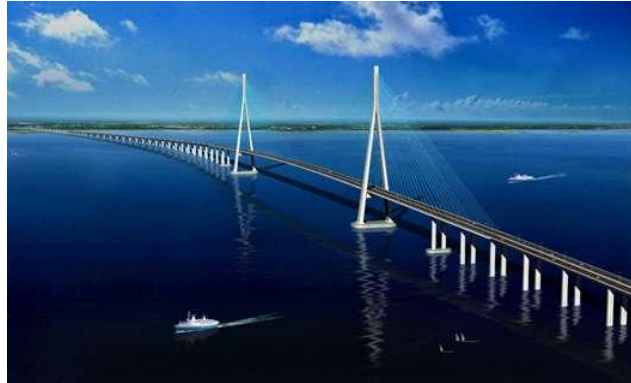
Figure 36 Sutong Bridge, longest cable-stayed span in the world (3570 ft) (courtesy of New Jersey DOT).
